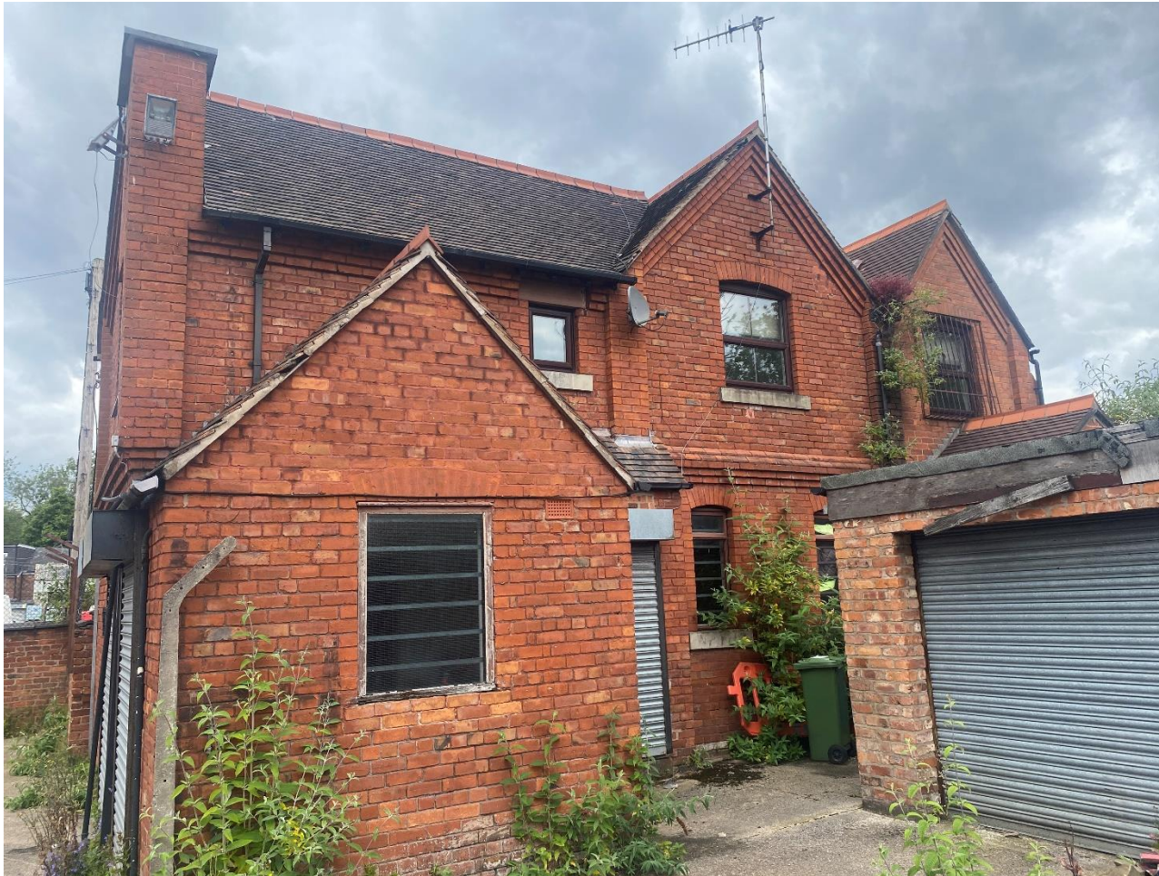
Photo 3: Southern elevation of B1.
