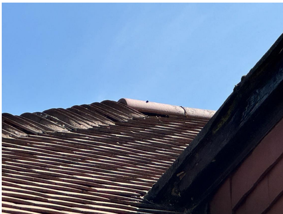
Photograph 8 - Raised ridge tile (Target Note 7)
