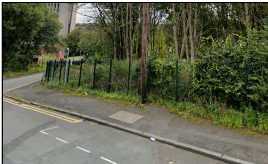
Online mapping (September 2020) shows the location of the Virgin Media underground chamber next to BT Pole.
