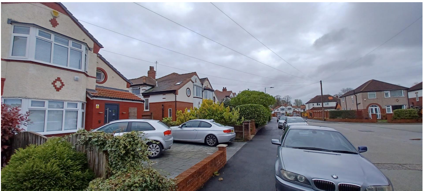
Figure 7. Precedent of similar works in surrounding area.
