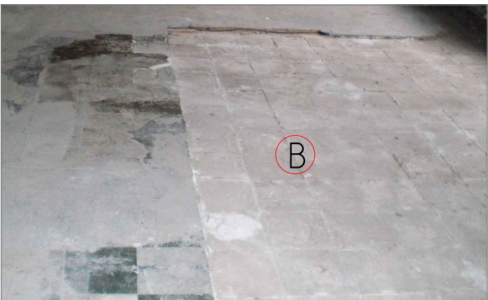
GROUND FLOOR EXPOSED SCREED
