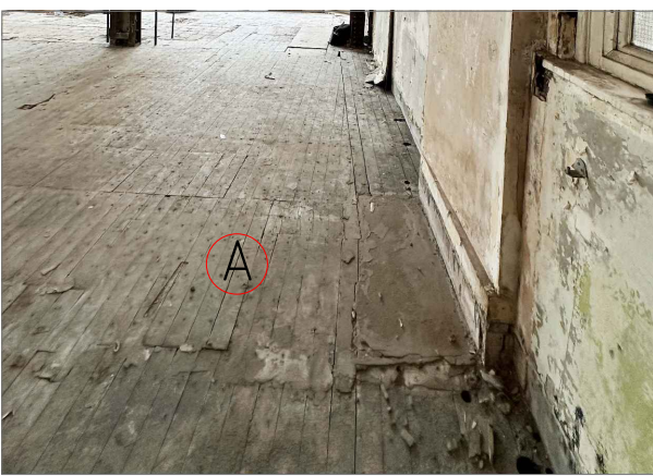
GROUND FLOOR FLOOR BOARDS
