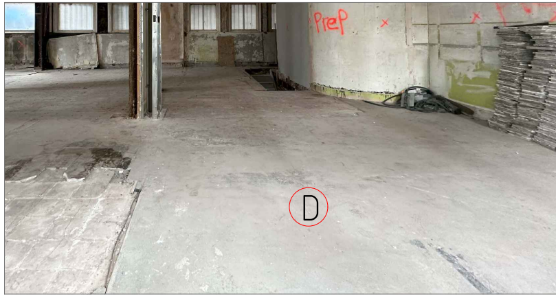
GROUND FLOOR LEVELING SCREED
