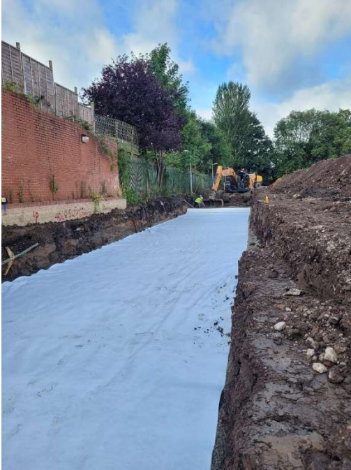
Images showing the attenuation tank being installed
