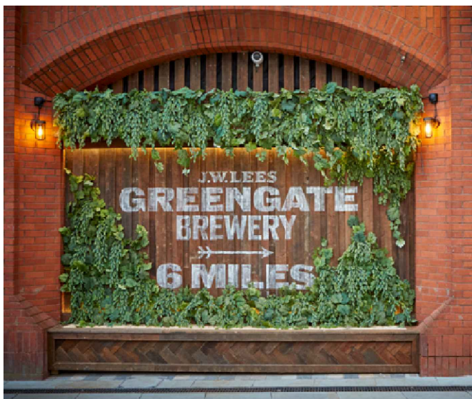
Photograph of as-built planters and reclaimed timber wall forming secure area for storing external seats and tables
