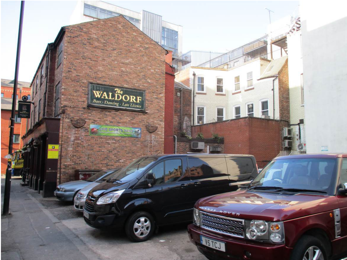
PLATE 3: CAR PARK ON GORE STREET
