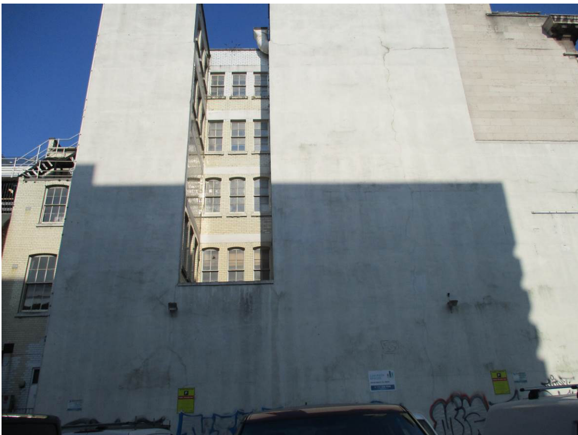
PLATE 3: REAR OF NOTHERN BUILDING
