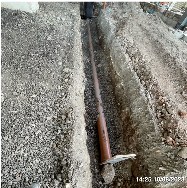
Observation 8 Drain line into F3
