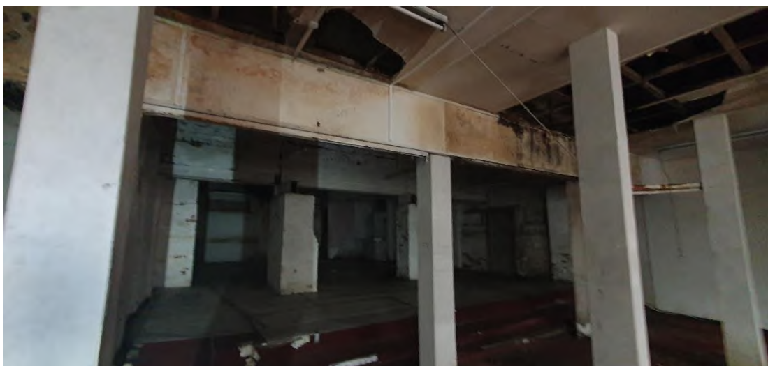
Photograph 7 – Interior of warehouses in southwest of the site
