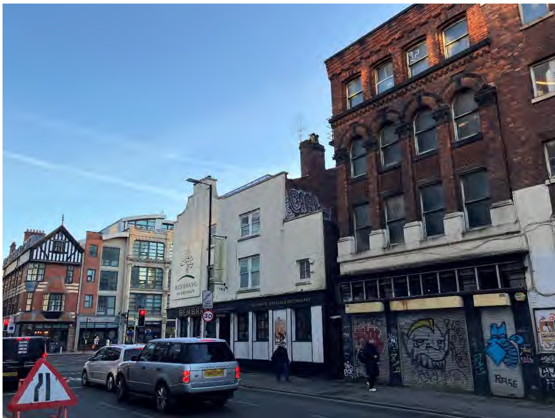
Photograph 4 - Photograph looking north-western elevation of the site from Lever Street
