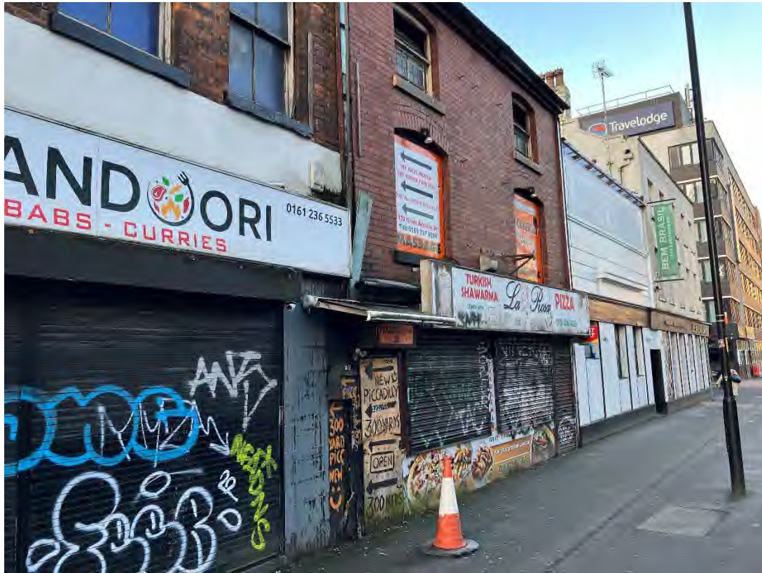
Photograph 3 – Looking along the north-eastern elevation of the site from Great Ancoats Street.
