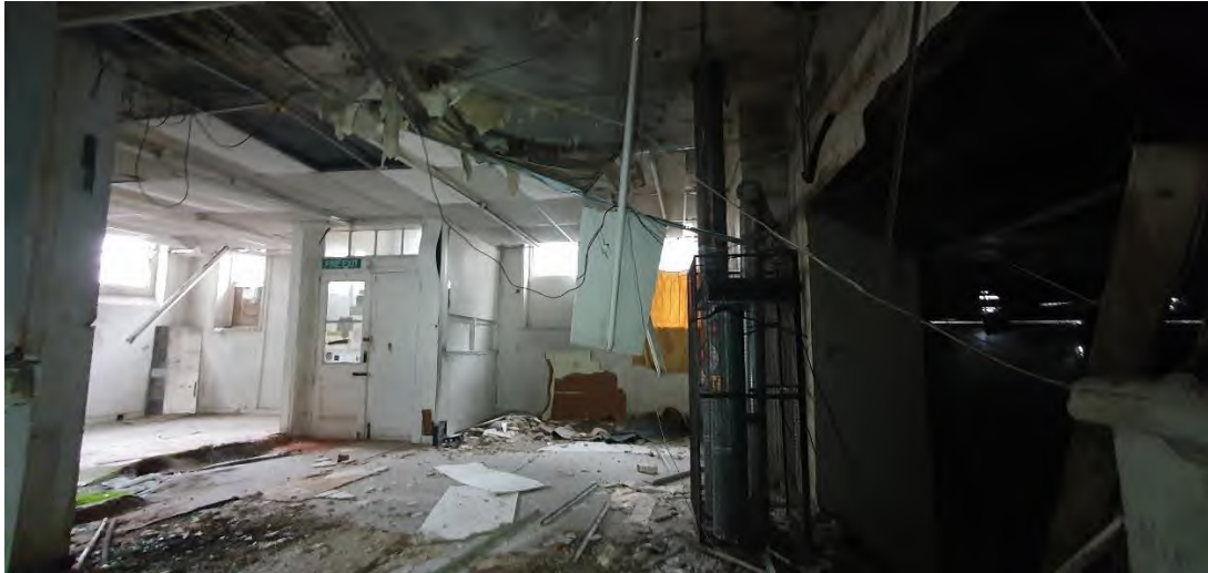
Photograph 5 – Interior of warehouses in southwest of the site
