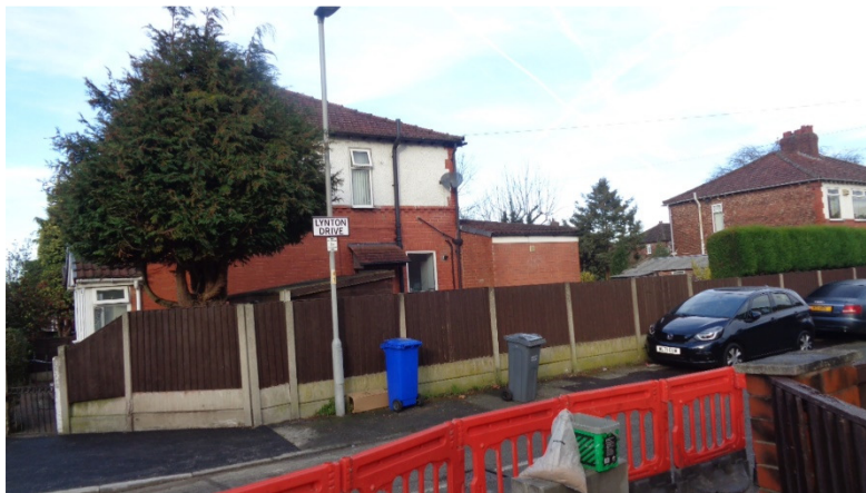
Gable Elevation of Application Property.
