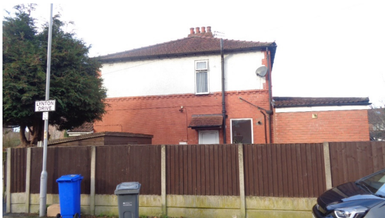
Gable Elevation of Application Property.
