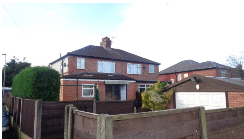
Rear of Application Property.
