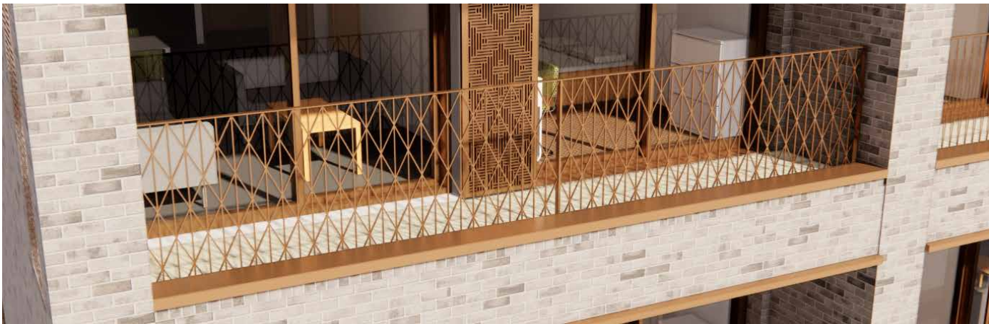
Metal projecting balcony balustrade
