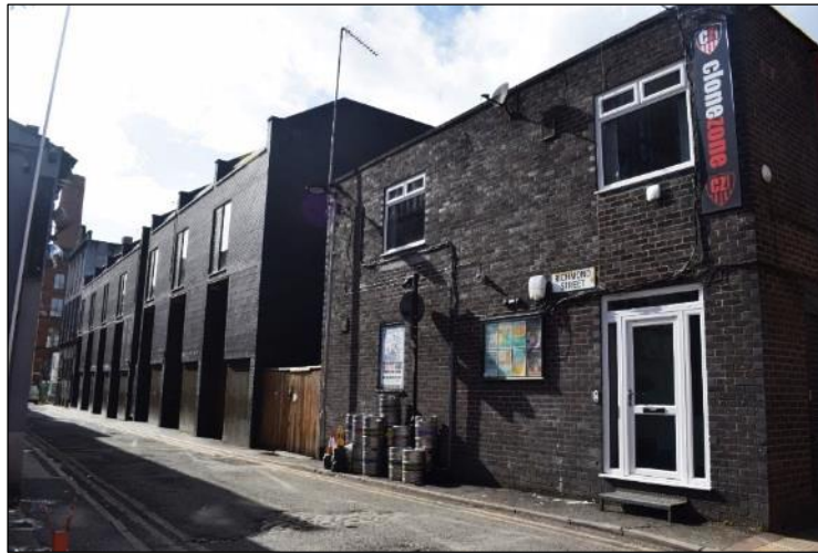
Photo 12: Modern infill, opposite site
