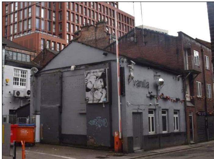
Photo 1: 39 - 41 Richmond Street, looking south
