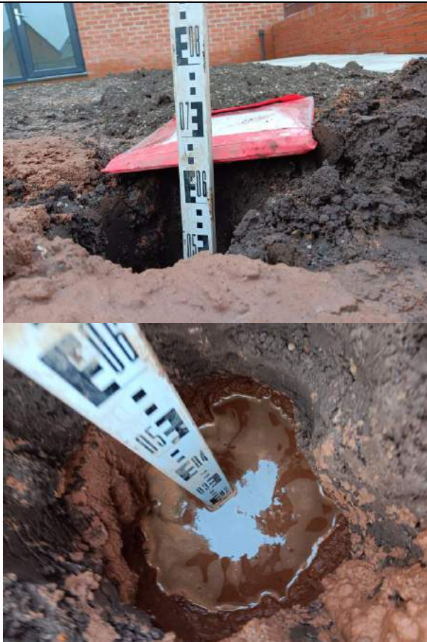
Photograph 8: Evidence of suitably chemically validated topsoil with a minimum of 150mm growing medium in garden areas (Plot 1) over natural strata.
