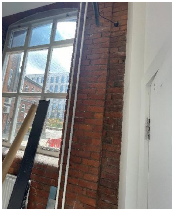
Figure 79: Room 07, showing the corner of the gable end of No 11 as it met with the rear elevation of the dwelling.
