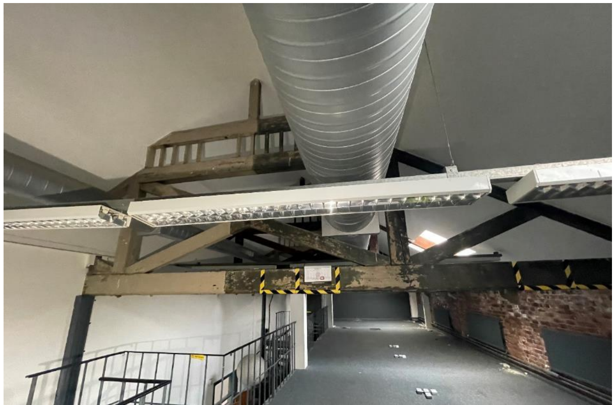
Figure 60: Looking west through the hay loft above room 27.
