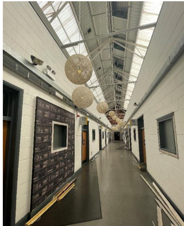
Figure 65: Looking east through the 1926-7 extension (room 37) showing the modern blockwork rooms to the left and right, and original steel truss roof structure.
