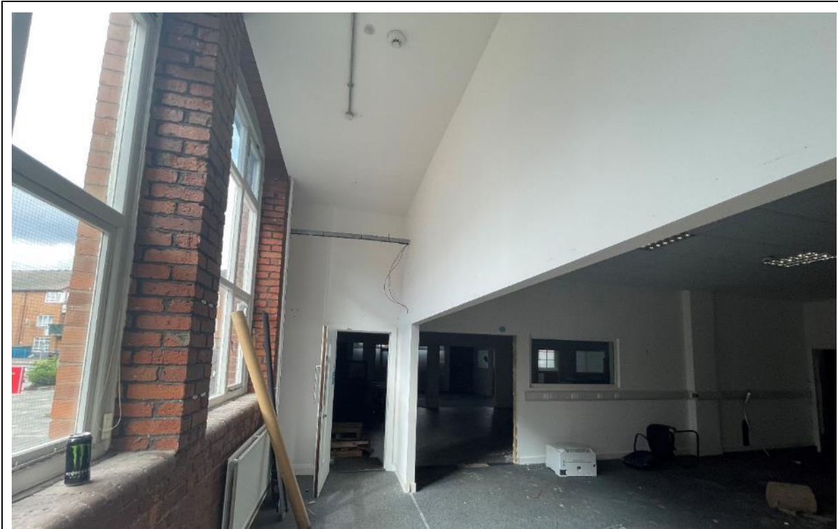
Figure 73: Looking west through room 07 (left) and room 08 (right).
