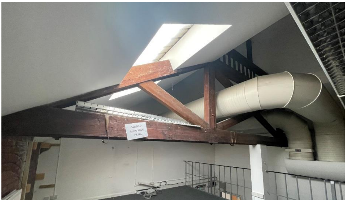
Figure 52: A view from the hay loft in room 17 (looking east).
