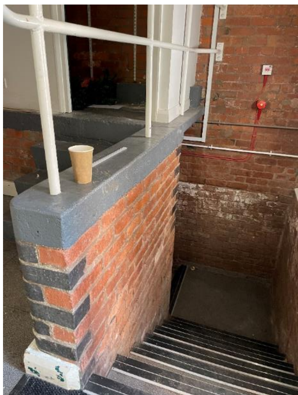
Figure 93: Looking into the basement stairs from room 13
