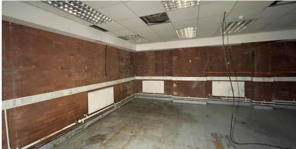
Figure 57: Looking north/north-west into the corner of room 17, showing what appears to be a chimneybreast and some alterations to the brickwork.
