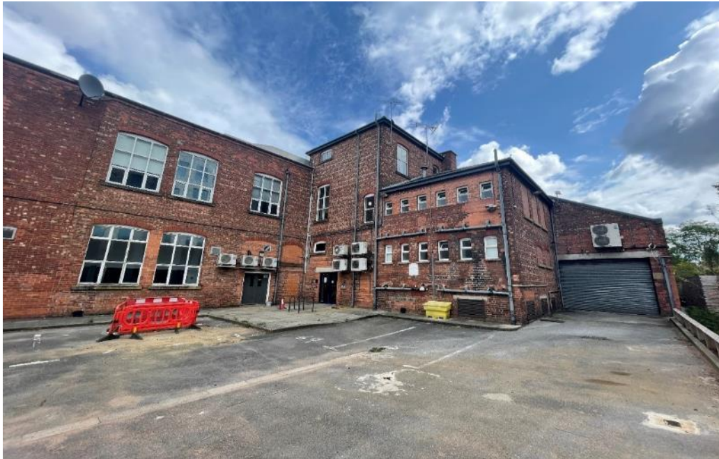
Figure 38: Looking east at the toilet block (right) and staircase hall (left)
