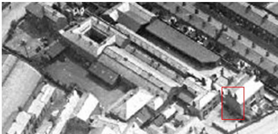
Figure 77: 1924 aerial view looking south-east across the site, showing the early 19 th century northern gable end of No. 11 Greenheys Lane outlined. When the 1926-7 newspaper stables extension was undertaken No. 11 was still standing, and so the gable was incorporated into the new build. No. 11 was then demolished in the 1930s/40s.
