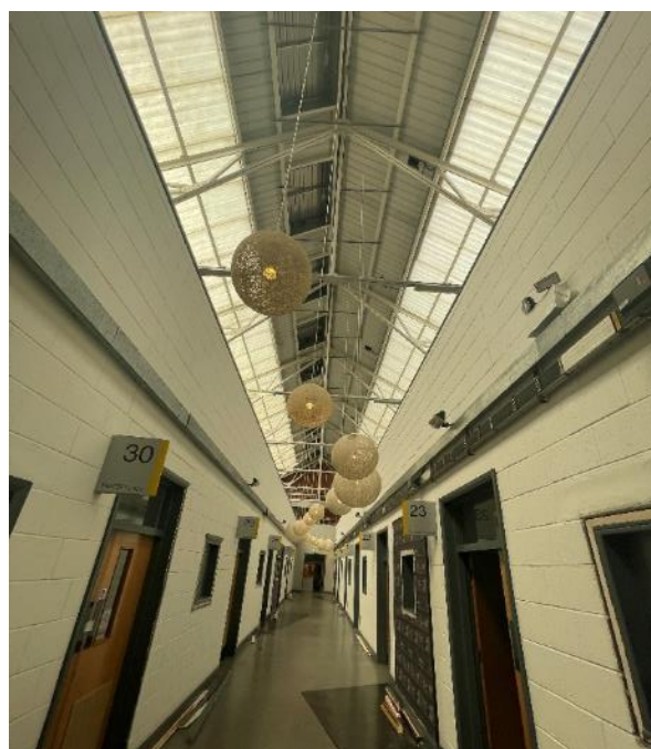
Figure 66: Looking east through the 1926-7 extension (room 37).
