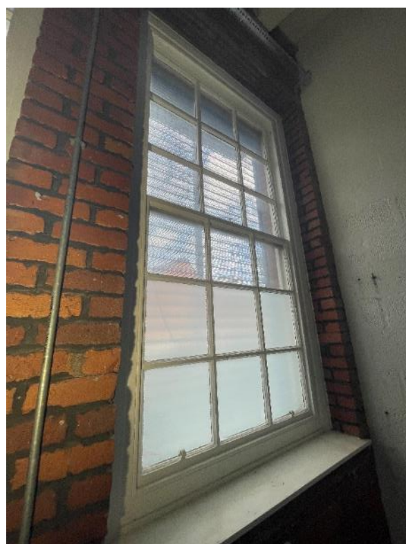
Figure 78b: Detailed view of one of the two sashes.
