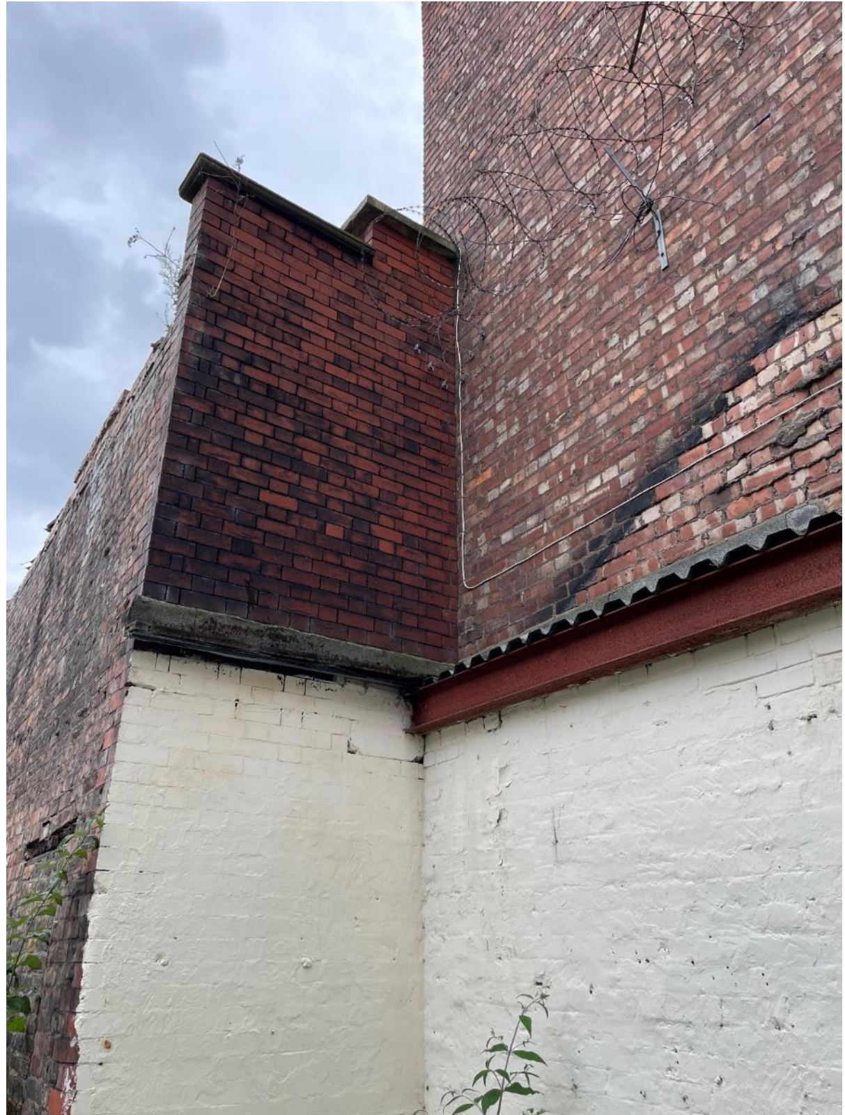
Figure 46: The original western front elevation of the 1893-1903 stables, which now forms part of the rear yard of the adjacent No. 9 Greenheys Lane. This elevation uses higher quality red brick and moulded capping stones.
