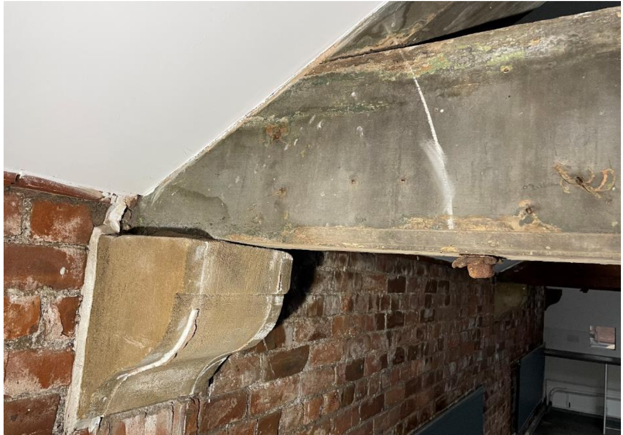
Figure 59: The hay loft in room 27, showing one of the original moulded stone corbels in the external wall.
