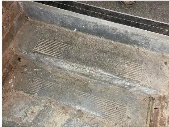
Figure 95: The stone basement steps with original non-slip treads cut into the stonework.
