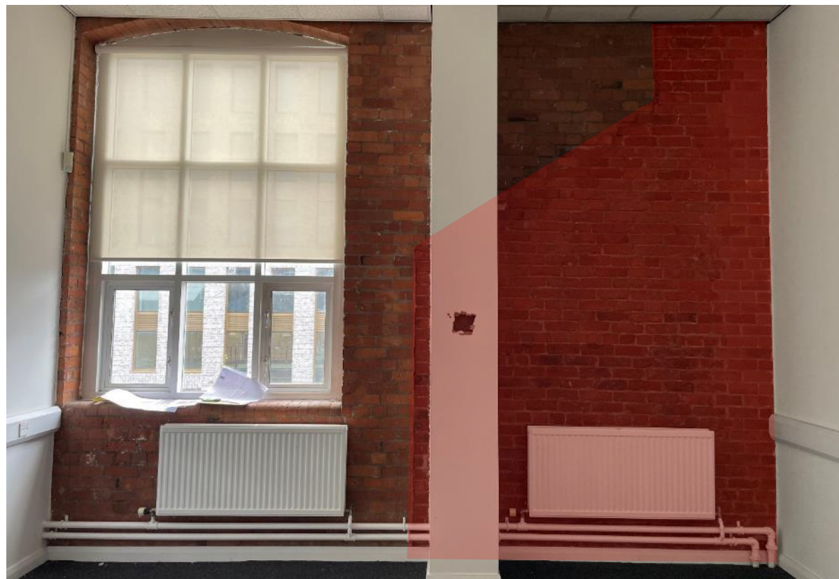
Figure 85: The southern wall of room 06, showing the first floor section of gable wall from No. 11, including the chimney and pitched roof (left).
