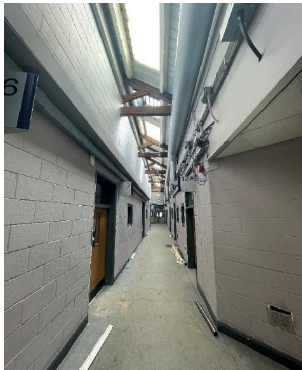
Figure 64: Looking east through the corridor in room 25, showing the modern blockwork rooms either side, and a narrow area of the building's original 1893-1903 roof structure.
