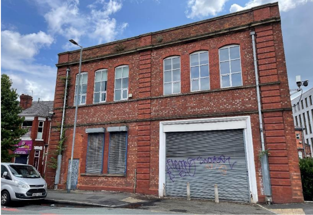
Figure 35: The principal western front of the 1926-7 building, showing the original entrance for the stables to the right. All windows were originally multi-pane timber sash windows, with only the two ground floor sashes now surviving. This elevation was intended to be extended to the right at a later date when the adjacent Nos. 11 and 13 Greenheys Lane were demolished, thus making a symmetrical frontage. It is not known why this later extension was never realised.
