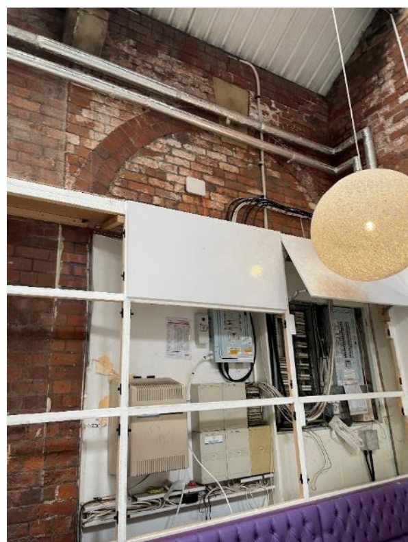
Figure 62: The blocked original entrance.
