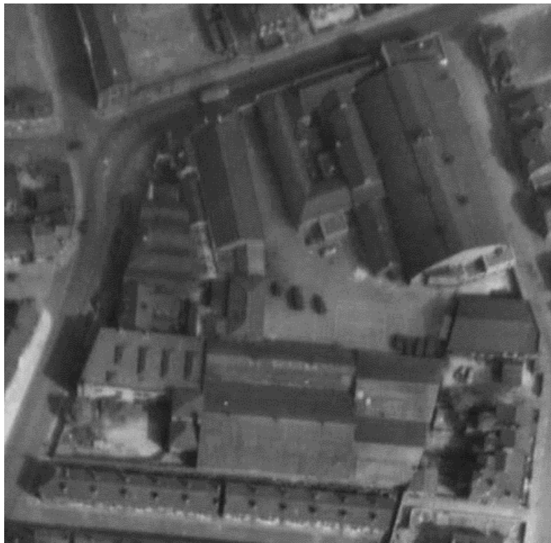
Figure 31: 1953 aerial view looking north, showing the Site to have remained the same. Note that the site of the demolished Nos. 11 and 13 has yet to be developed. (Source: Britain From Above)
