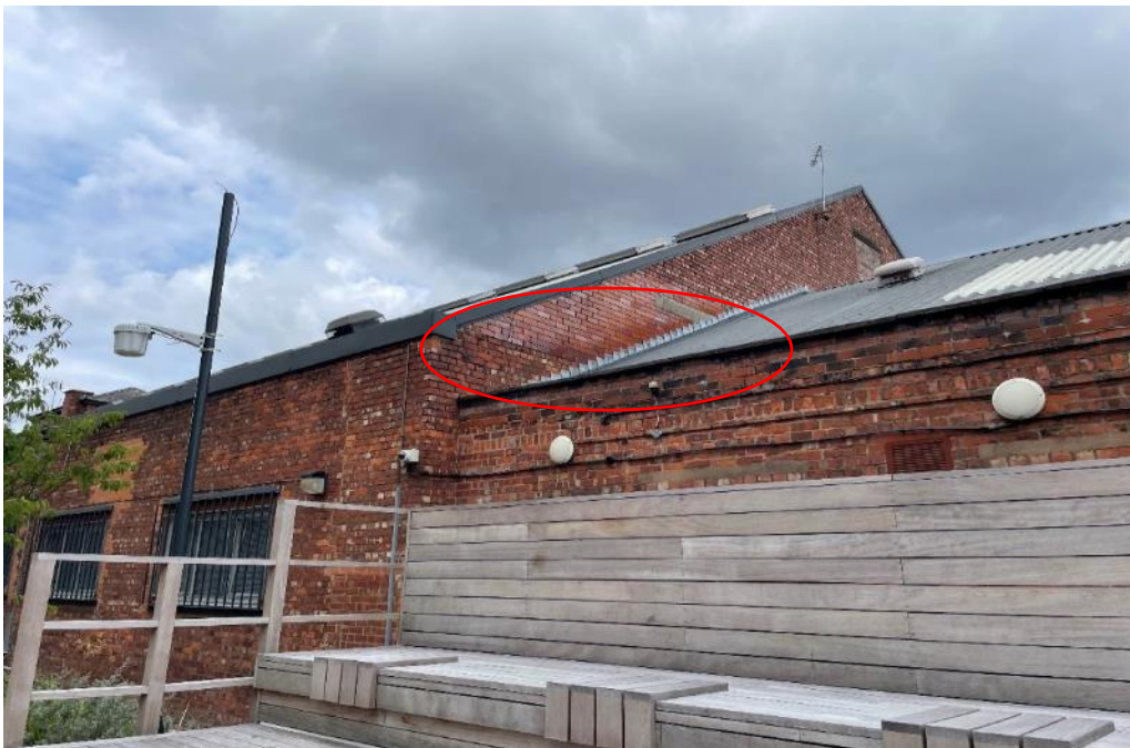
Figure 41: The join between the 1920s and 1930s shed, showing an area of brown glazed brickwork and stone lintel in the eastern gable end of the 1920s building, which is likely to have originally formed part of the two lightwell structures that were demolished and replaced with the current 1930s shed to the right.
