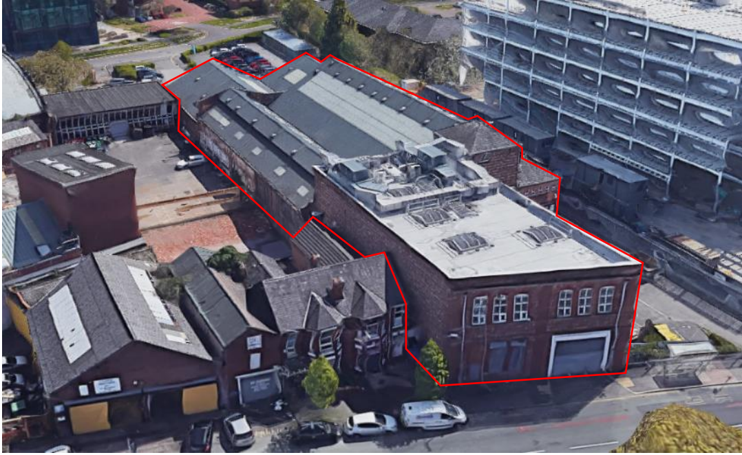
Figure 2: Aerial view looking east at the Greenheys Building (outlined) (Source: Google Maps).
