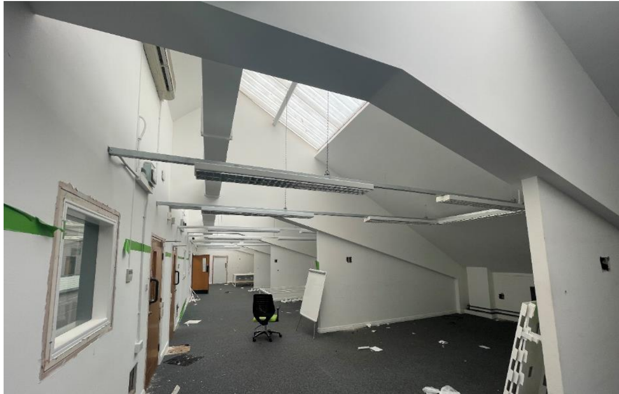
Figure 83: Looking east through the open plan rooms along the southern side of the first floor of the 1926-27, which are accessed from room 25.
