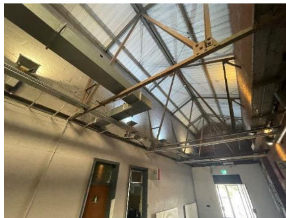
Figure 80b: Looking east at the steel truss roof of the 1936-7 extension (room 52)
