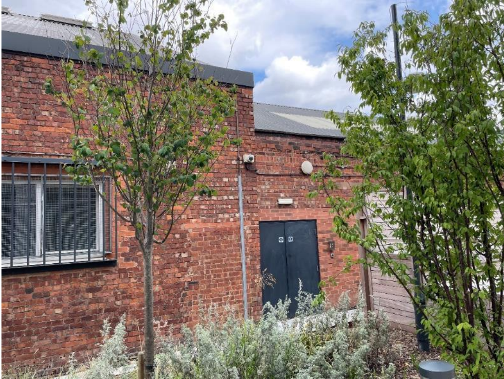
Figure 40: The south elevation of the 1926-7 shed (left) where it meets the 1936-7 shed extension (right).
