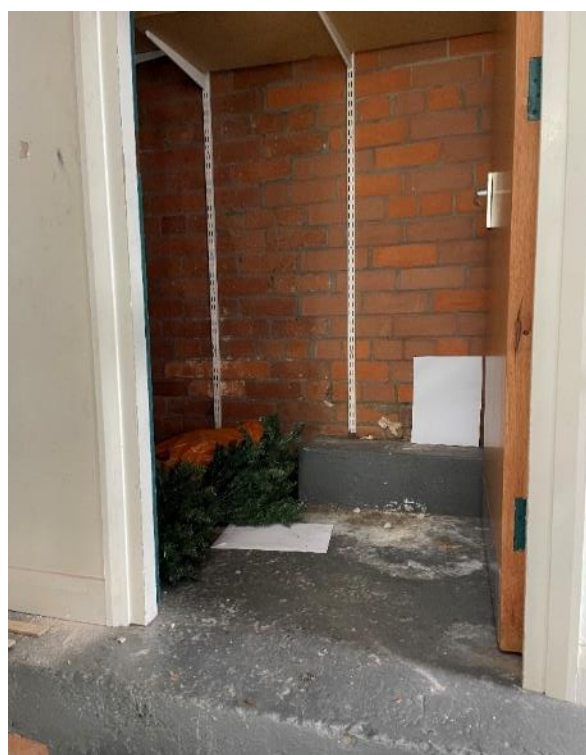
Figure 72: The blocked door opening into the original male toilets.
