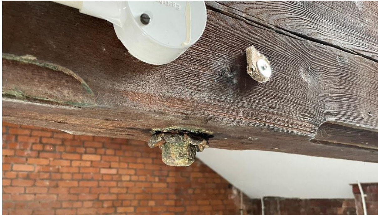
Figure 55: An example of the decorative flower nut and bolt to the underside of the roof structure. Note the decorative chamfer mouldings.
