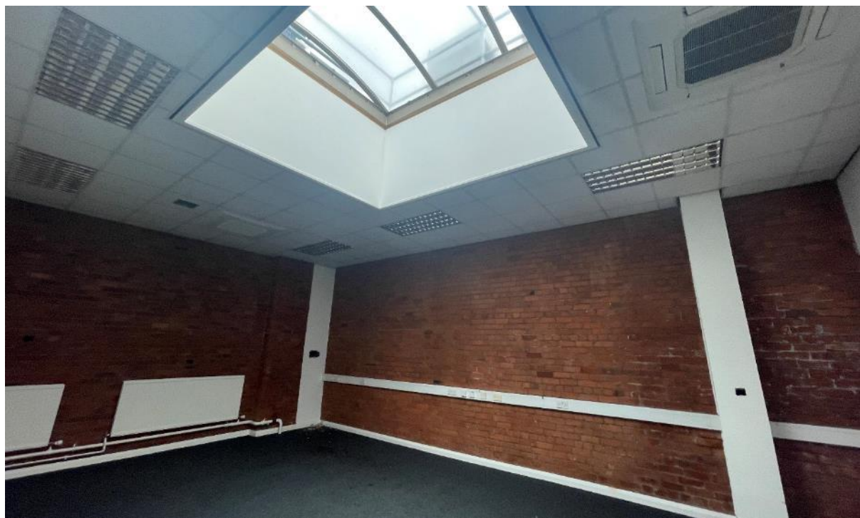
Figure 84: Looking north-east through room 11.
