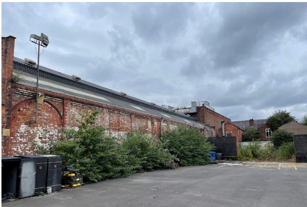
Figure 43: The north elevation of the 1893-1903 stables, showing the original external wall and now blocked arched entrance (left).
