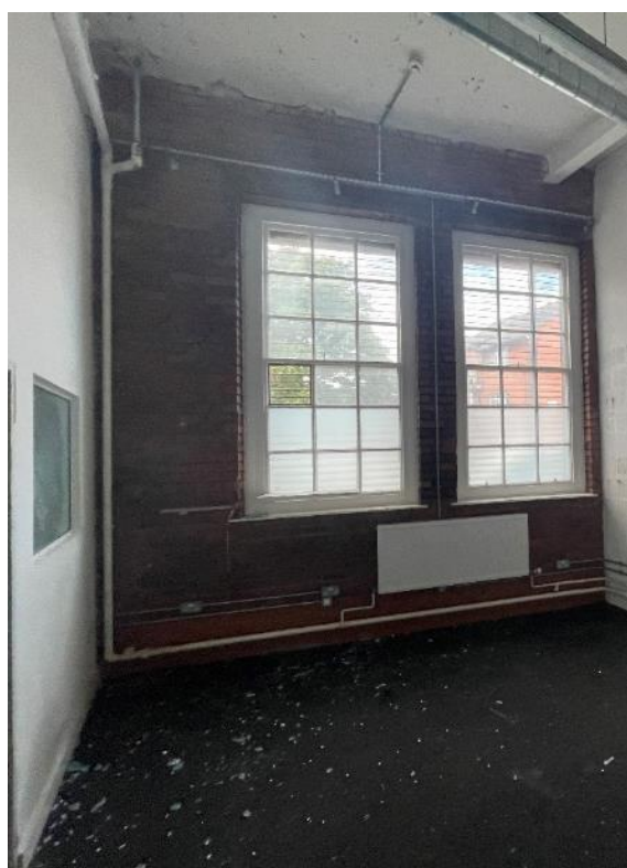
Figure 78a: The two remaining original 1926-7 multi-pane timber sash windows to the west elevation of room 02.
