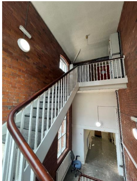
Figure 90: Looking up into the second floor level from the staircase, which gives access to the roof level.
