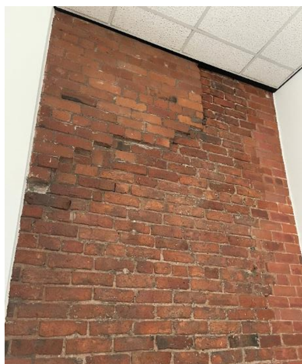
Figure 86: Detail of the outline of the pitched roof and chimney of No. 11.
