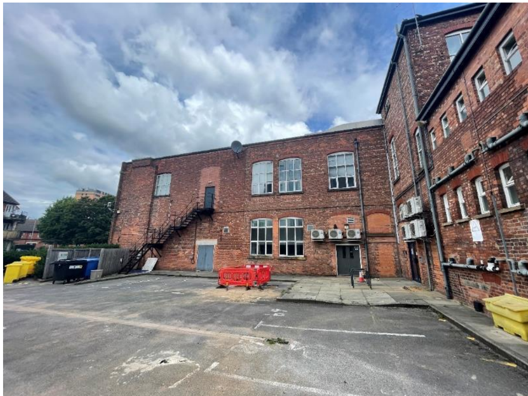
Figure 37: Looking north at the southern elevation of the 1926-7 entrance building.
