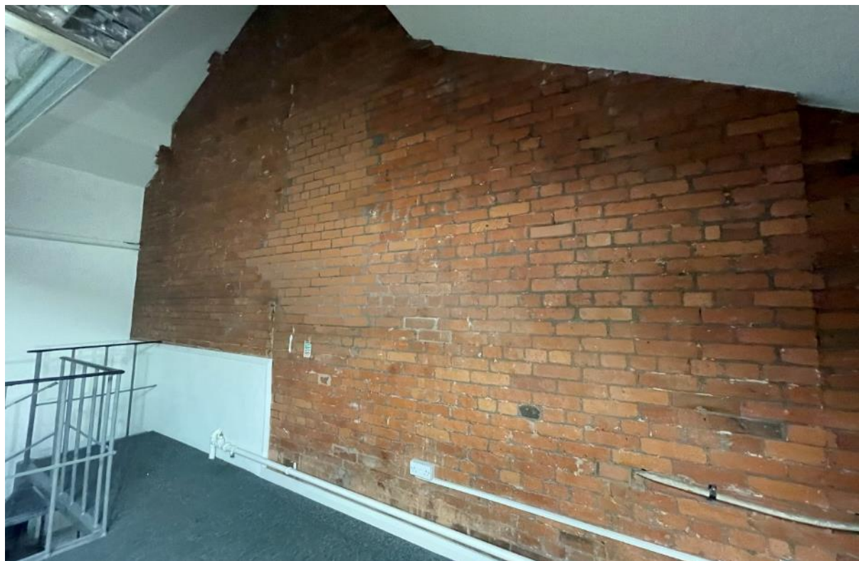
Figure 56: The west wall of room 17 and its hay loft, showing later alterations to the centre and right sides, whilst the applied painted boarding to the left denotes the original location of the stable's entrance from Greenheys Lane.
