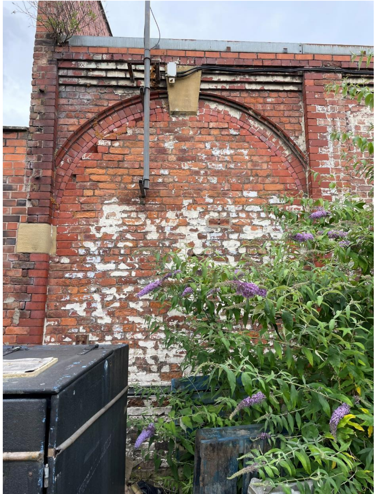
Figure 45: The now blocked original entrance into the stables from the north.
