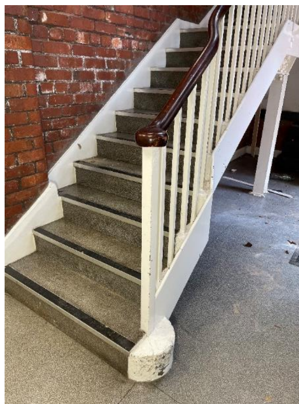
Figure 69: Detail of the 1926-7 staircase.
