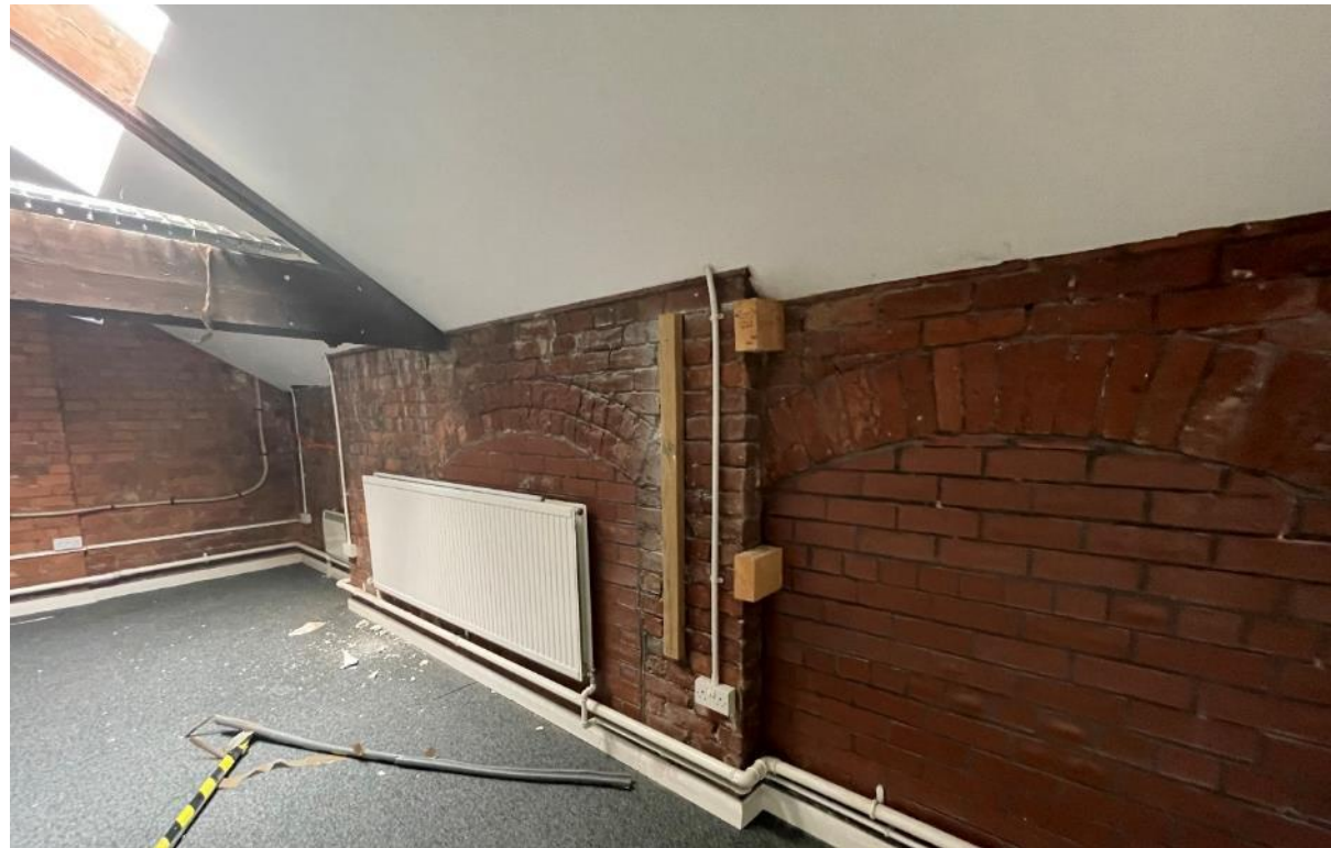
Figure 53: The northern wall of the hay loft in room 17, showing three now blocked openings.
