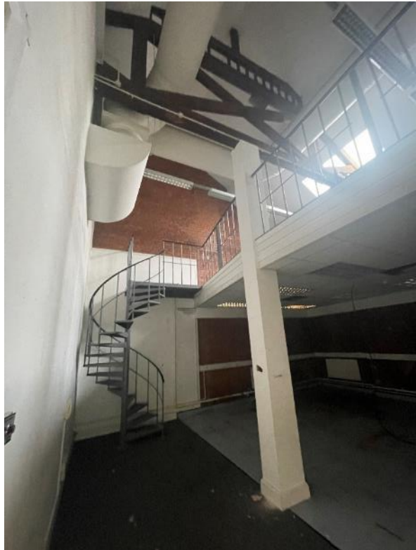
Figure 50: Looking west towards the original 1893-1903 entrance wall of the first phase of the stables (room 17), showing the original exposed roof structure and hay loft.
