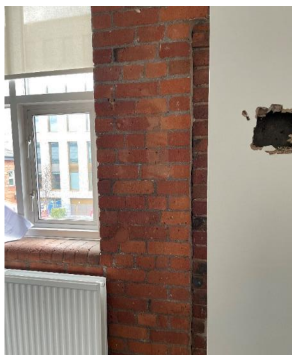
Figure 87: The vertical joint marking the end of No. 11's gable (right) and the start of the 1926-7 building (left).
