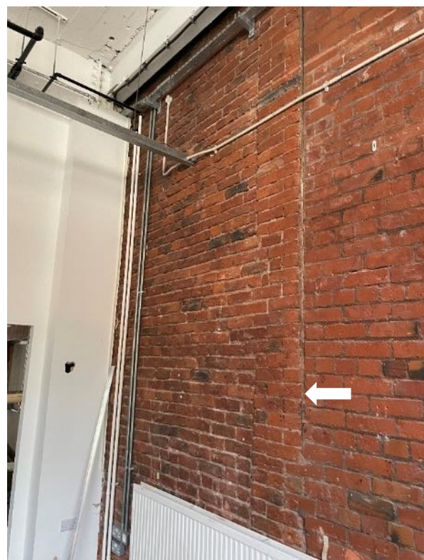
Figure 75: A detail of the original front (west elevation) of No. 11.
