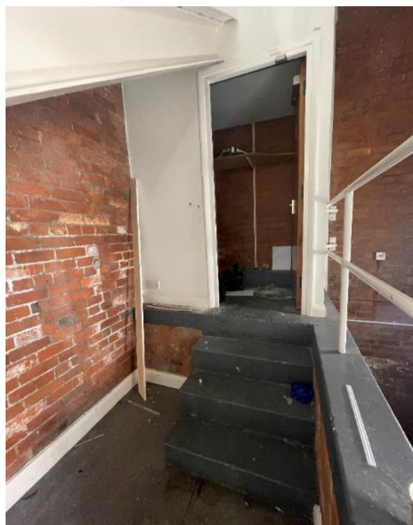
Figure 71: Looking south into the original entrance into the male toilets beneath the main staircase. The entrance into the toilets (rooms 15-16) is now accessed from room 20.
