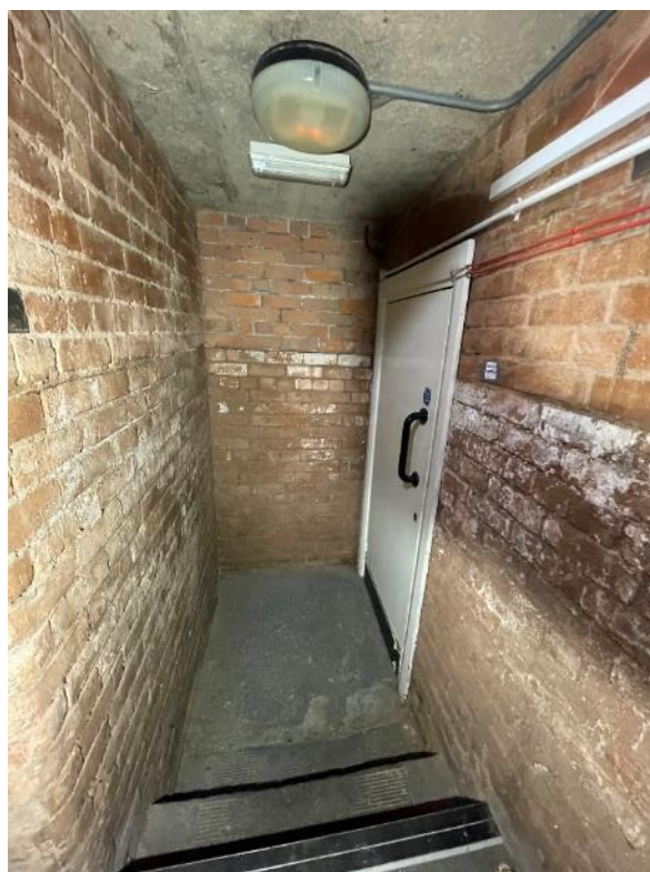
Figure 94: The basement entrance.
