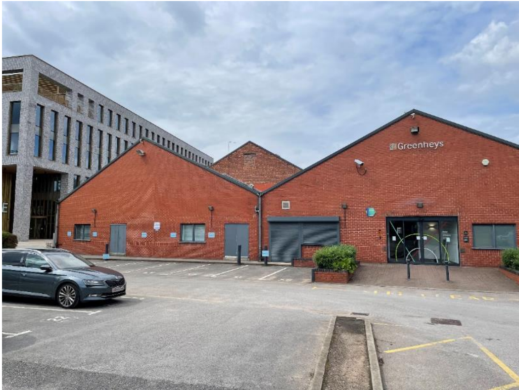
Figure 42: The eastern elevation of the 1930s shed (showing a modern brick skin) with the gable of the 1920s shed in between.
