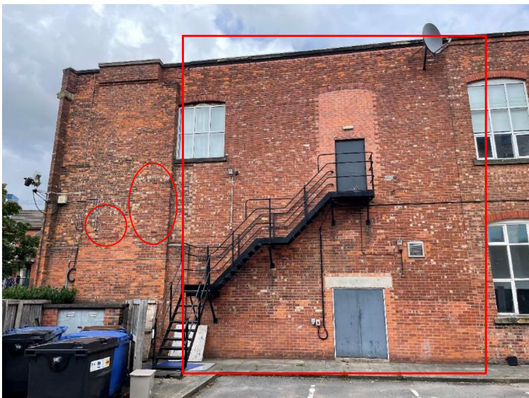
Figure 39: The south elevation of the entrance building, showing the original location of the gable wall of No. 11 (red square), whilst the two red circles show the location of a fireplace and a doorway which it is presumed was in anticipation of future expansion of the building on the empty plot in the foreground.
