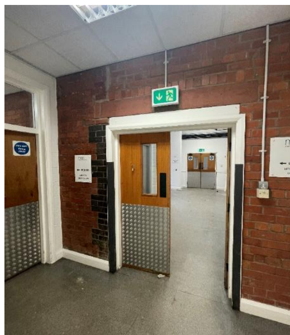
Figure 67: Looking west from room 19 into room 13, showing the original 1926-7 blue brickwork of a door jamb (left) and the insertion of a wider, modern double doors.
