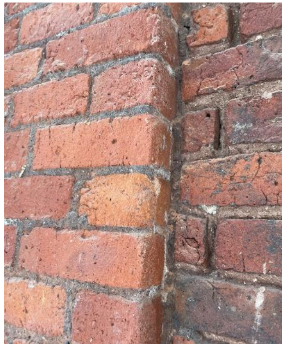
Figure 80: Closer view showing the end of No. 11 (right) and the 1926-7 building to the left.
