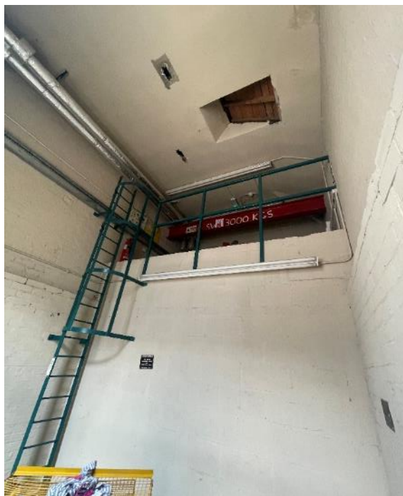
Figure 91: The lift mechanism room looking north-west.
