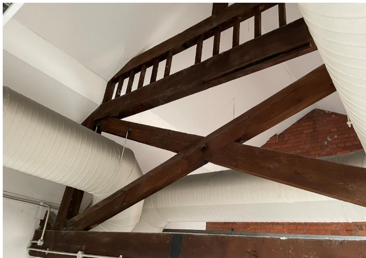
Figure 54: Looking west at the exposed roof structure in room 17's hay loft.
