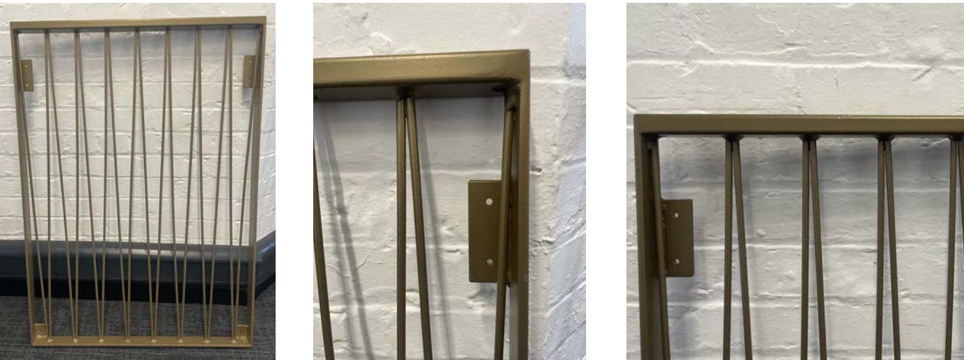
The images above show the initial design for the new balustrade, which proposed this angled rods in a 'zig-zag' format as a loose reference to the diamond motif.
