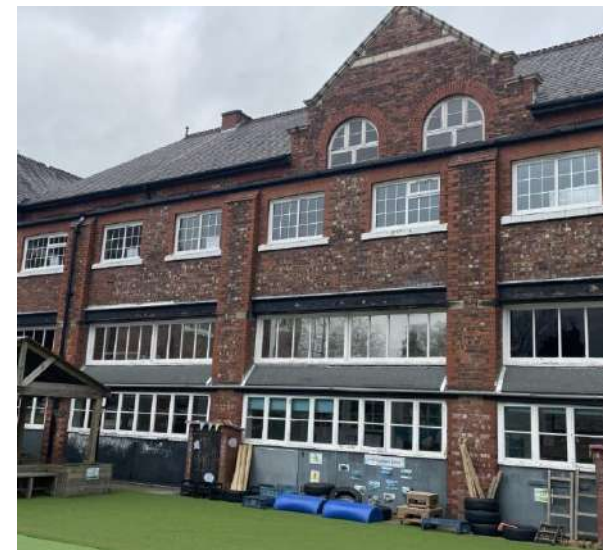
2nd Floor Classrooms. Solar Control Glass. Type 4 Glazing
