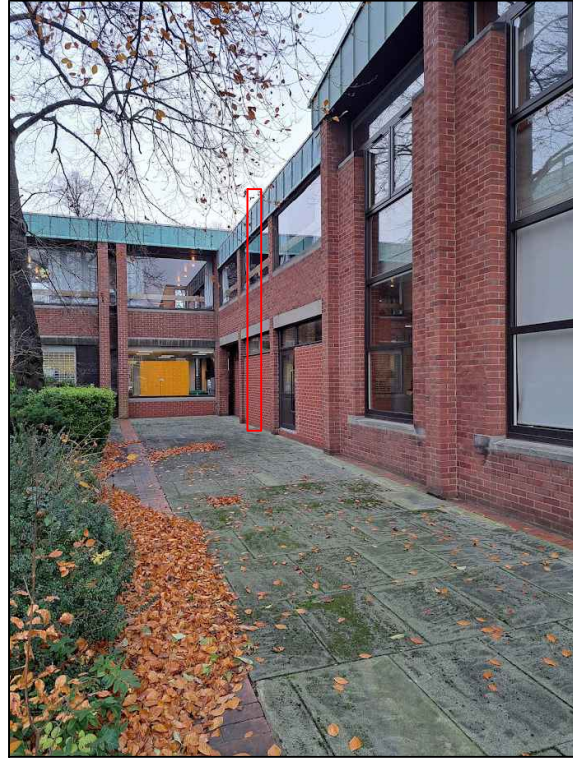
Photo 2. Rear of Reception - Ladder location considered and discounted to avoid impacting on glazing and key architectural features
