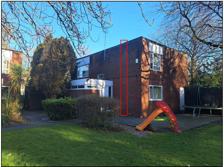
Photo 10. Rear of RLO Building / Wardens Lodge - Proposed ladder location
