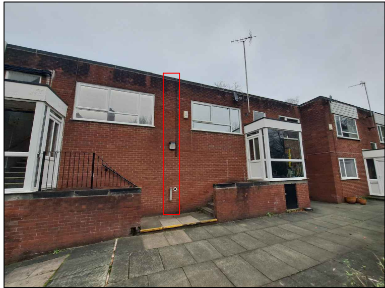
Photo 9. Rear of Accommodation block - Proposed ladder location
