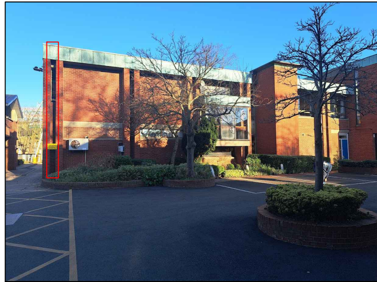
Photo 6. Rear of Reception & Bar - Ladder location considered and discounted to avoid impacting on key architectural features and being on a prominent elevation
