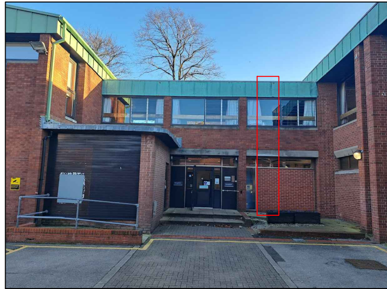
Photo 1. Main Entrance / Reception - Ladder location considered and discounted to avoid impacting on glazing, key architectural features and being on a prominent elevation
