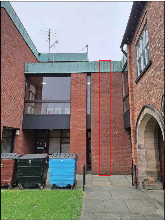
Photo 8. Rear staircase - Ladder location considered and discounted to avoid impacting on the Grade II building
