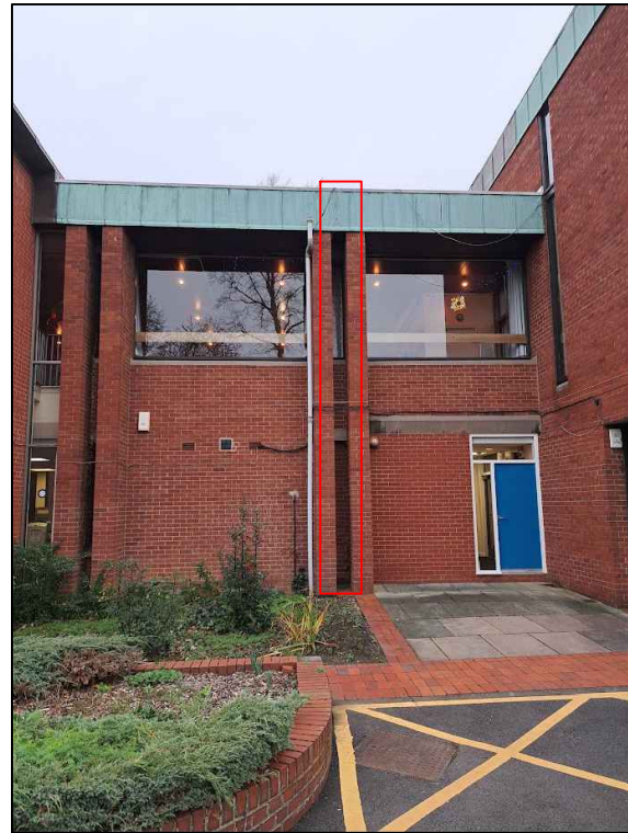
Photo 7. External entrance to Officers - Ladder location considered and discounted to avoid impacting on key architectural features
