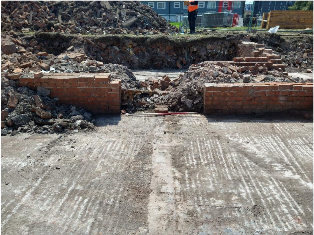
Plate 33: Gap for doorway between southwest end of wall [114] and northeast end of wall [111], looking southeast. Scale: 1 x 1m.
