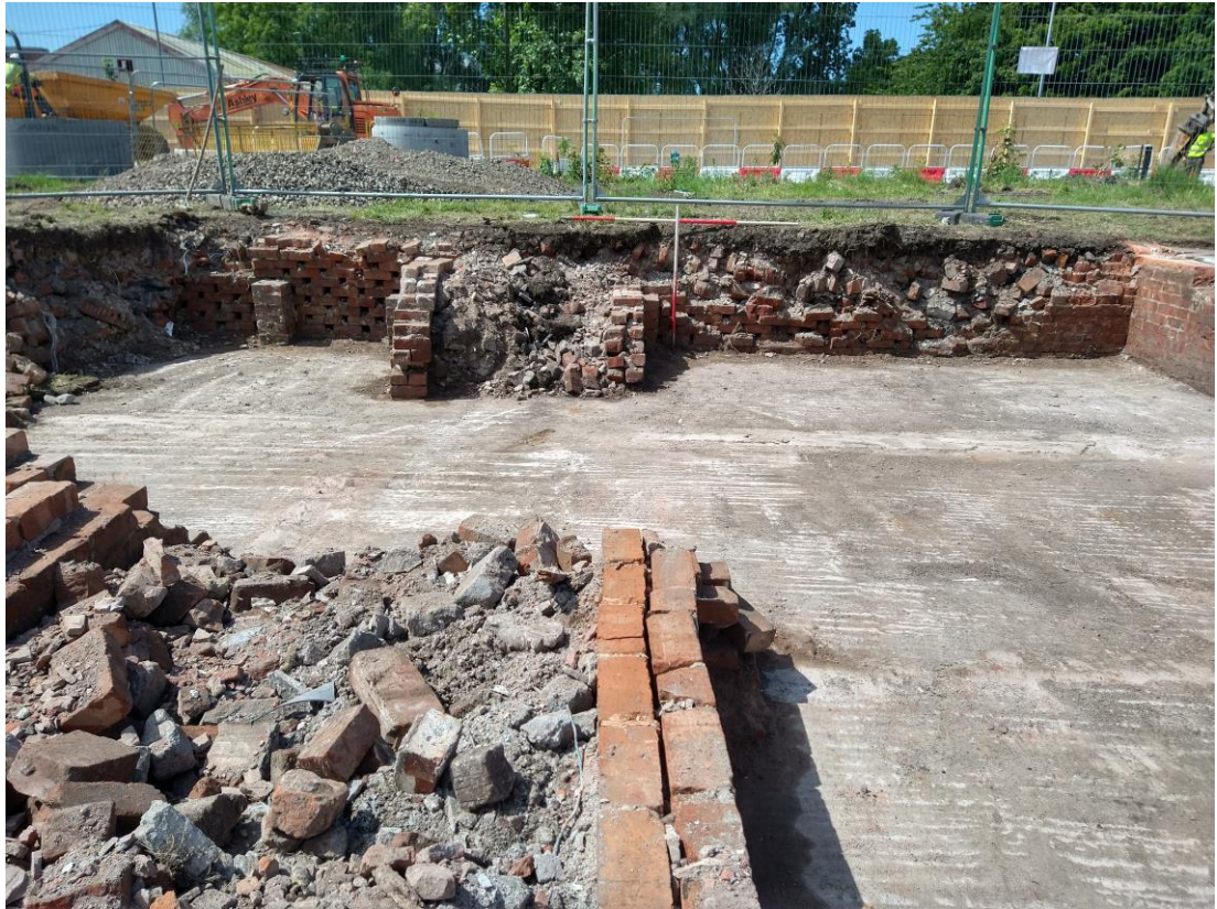
Plate 30: General shot of wall [104] with buttresses [107] and [108], and walls [106] and [105], looking southwest. Scale: 1 x 2m and 1 x 1m.
