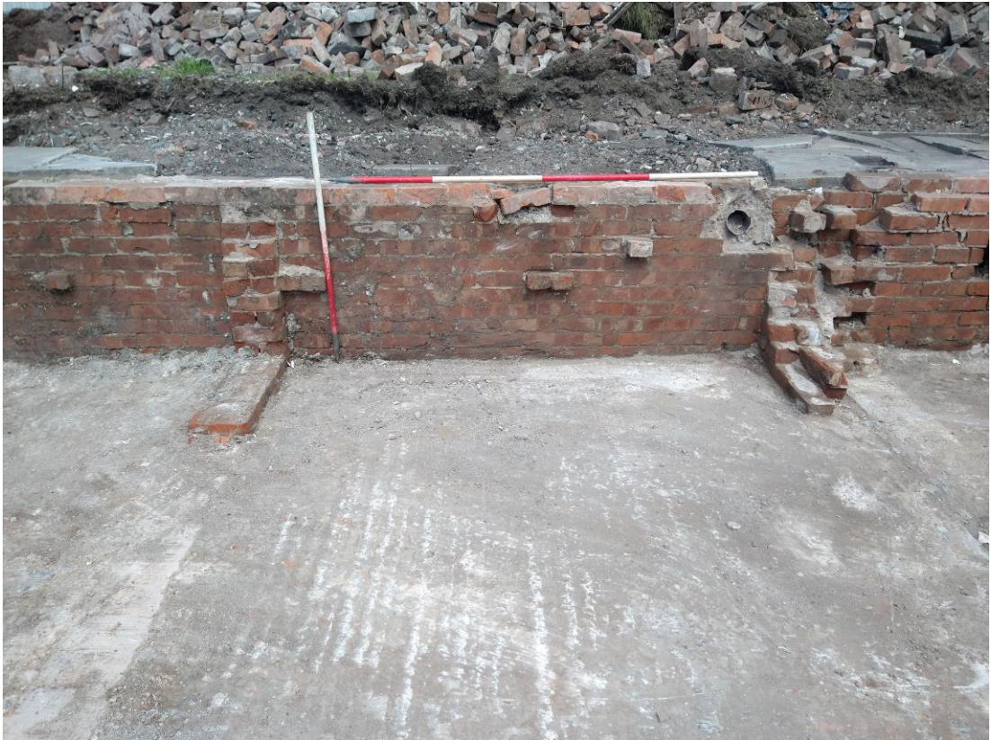
Plate 26: General shot of southeast face of wall [103] looking northwest. Scale: 2m and 1m.
