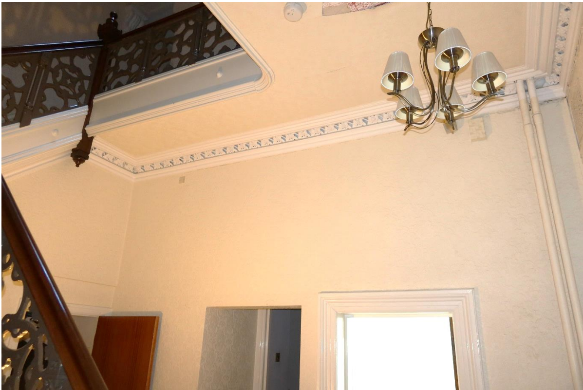
Fig 1: Typical decorative plaster and joinery details in the stairwell
