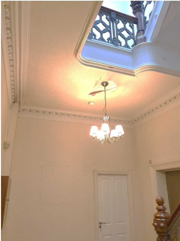
Fig 2: Typical location of smoke detector in stairwell. Remove existing equipment, replace with new. Access to cable route from floor above, using existing access provision
