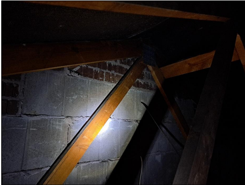
Photograph 4 showing the northwest gable wall
