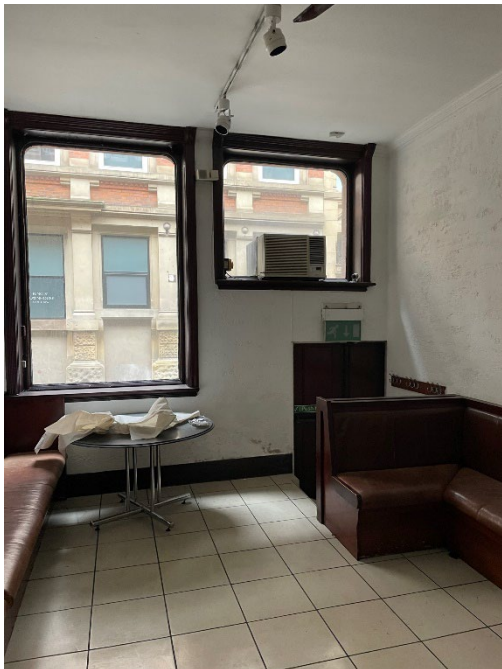
Figure 14: Looking north-east onto Kennedy Street. Some original walls and cornice remain, but internally the finishings are modern and of no heritage significance .
