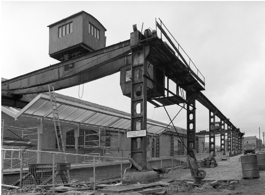
Figure 6: The Crane Gantry, 1982.
