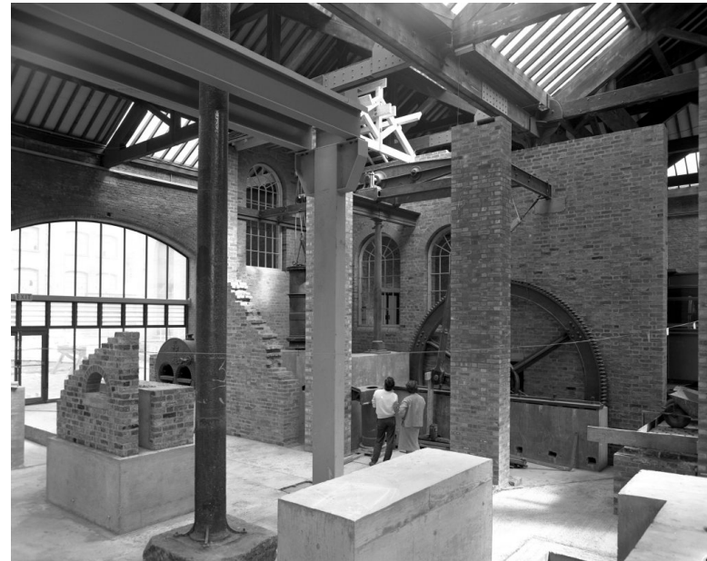
Figure 5: Power Hall progress shots from 1982-1983.
