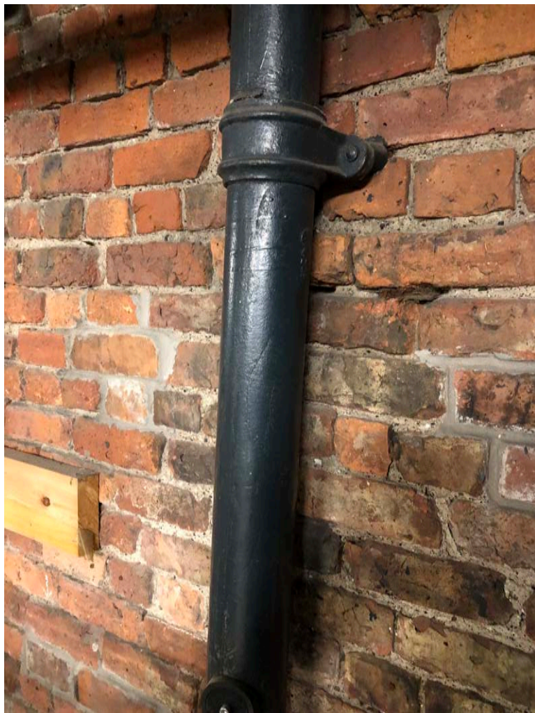
Figure 8: Representative rain water goods, section of internal downpipe (now identified as late C20th replacements)
