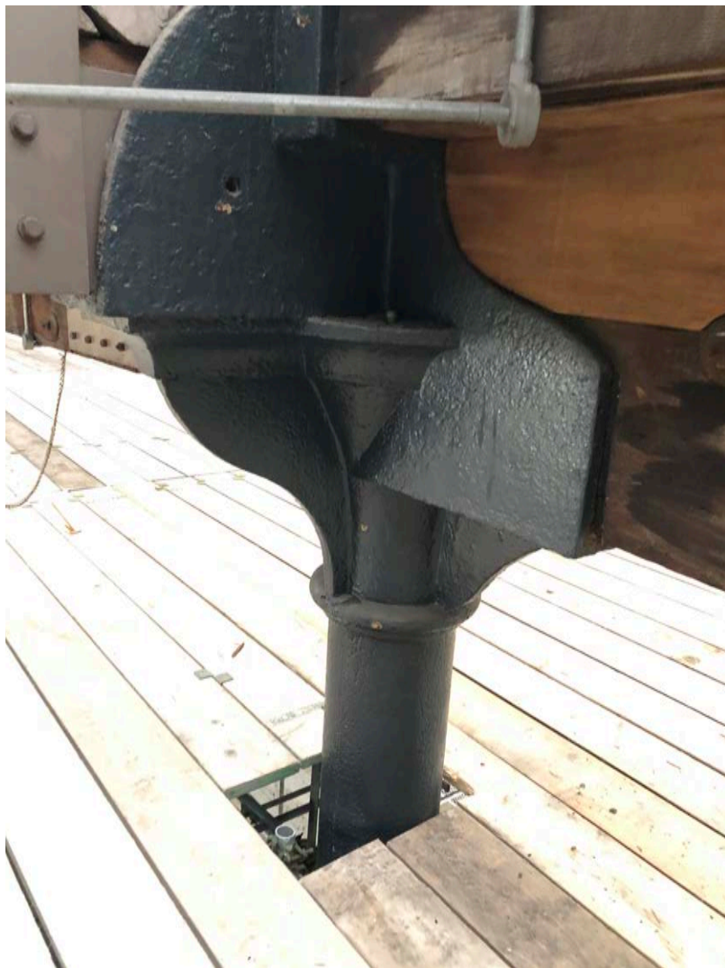
Figure 12: Large iron column capital
