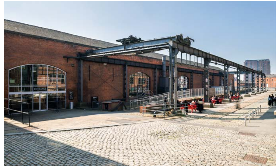
Figure 7: The Crane Gantry in its present form
