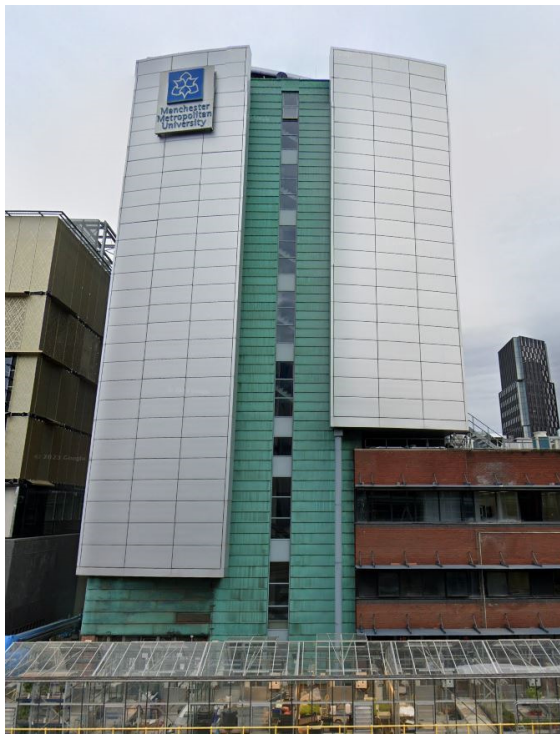
Existing Sign and Fixings showing impact on numerous cladding panels
