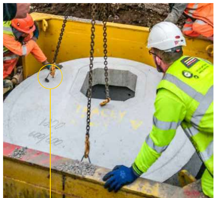
Cast in lifting loops
