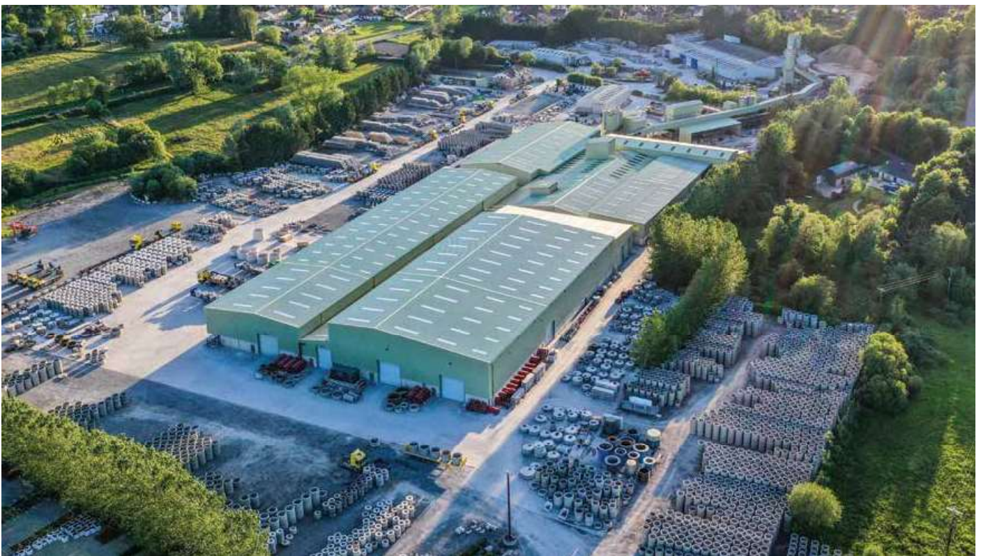
Tracey Concrete's Precast Drainage Factory - Enniskillen
