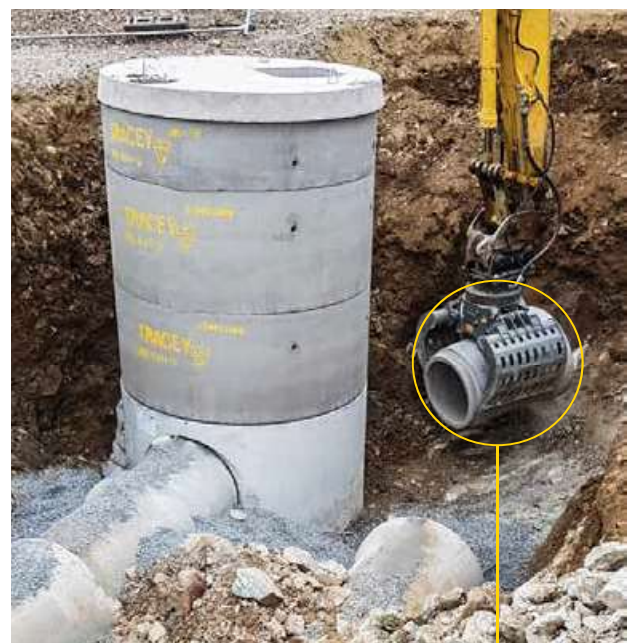
Rocker Pipe being installed
