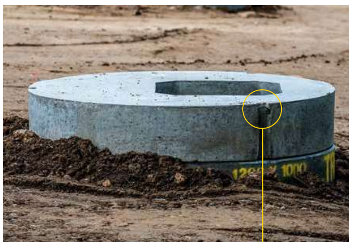
Cast in lifting loop
