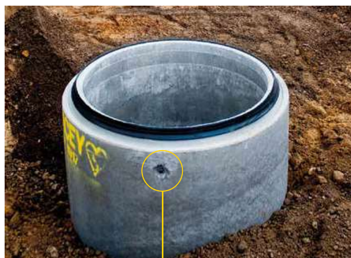
Cast in lifting Anchor
