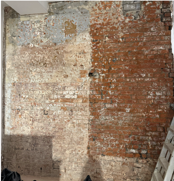
Figure 6: Existing brickwork on site
