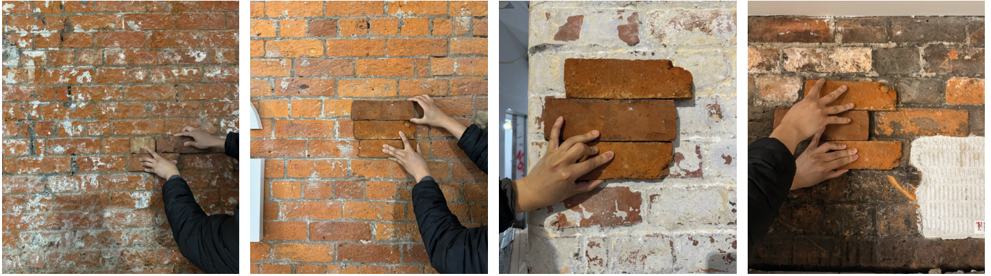
Figure 4: Existing brickwork on site with the proposed Oldham brick slip
