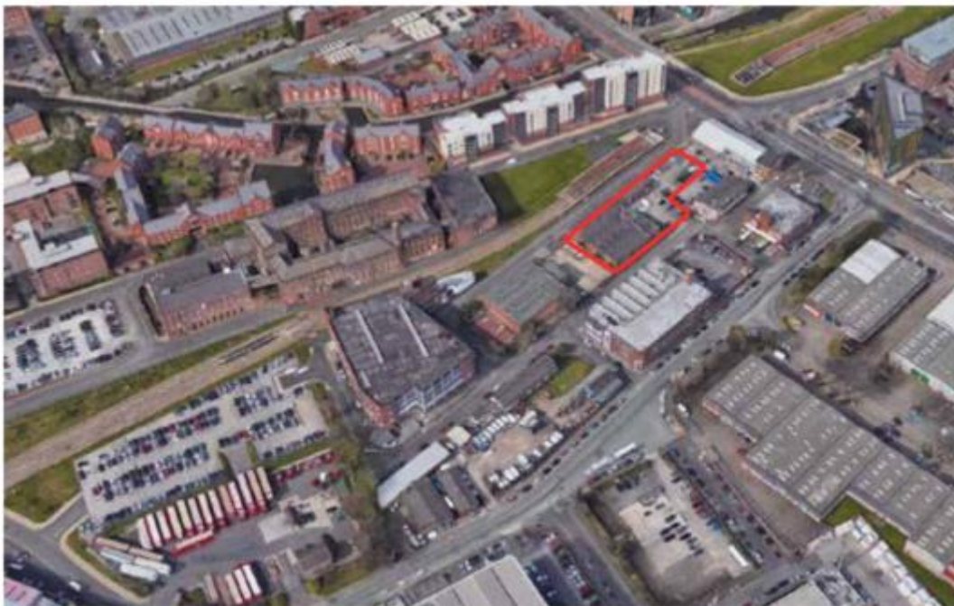
Site Location: Aerial View from the south
