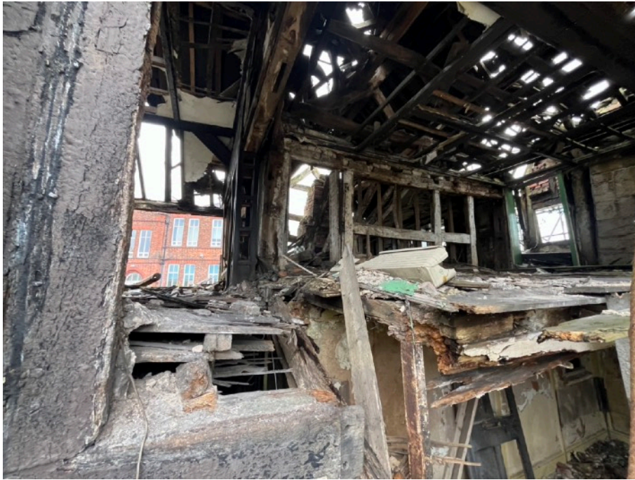
The timber frame is evident within the west wing.
