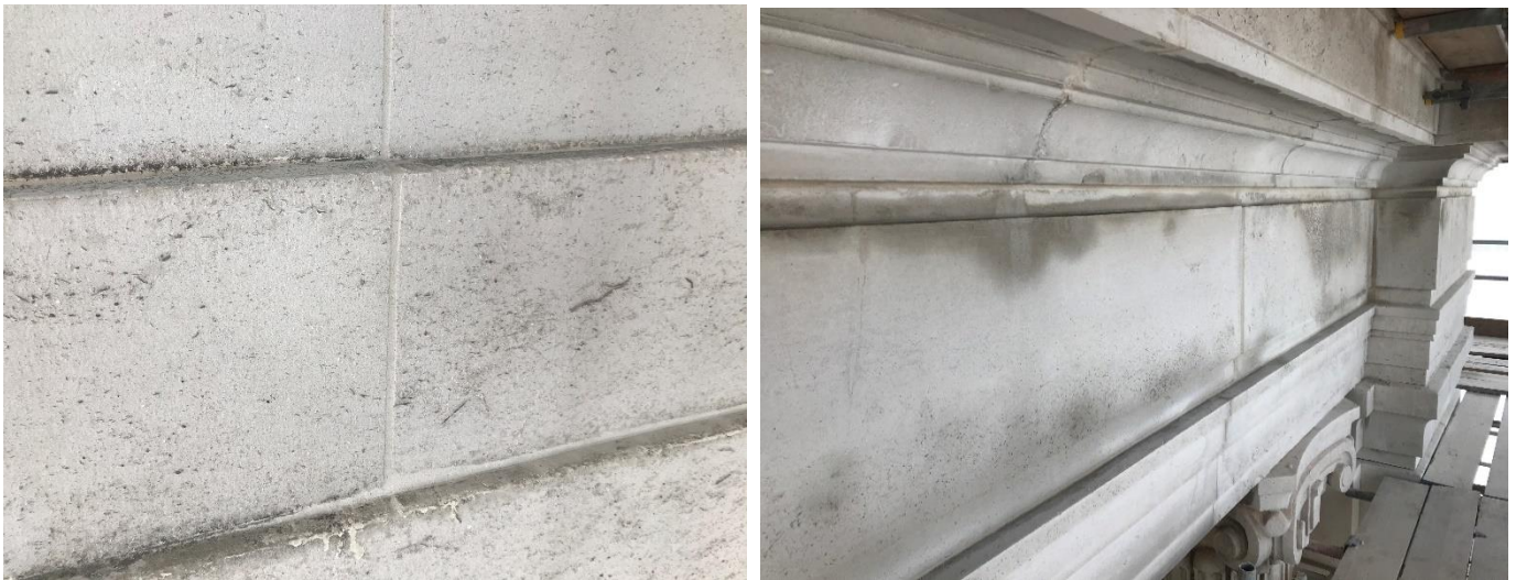
Figure 3a and 3b – Examples of previous installations finished product of cabling chased into mortar joints
