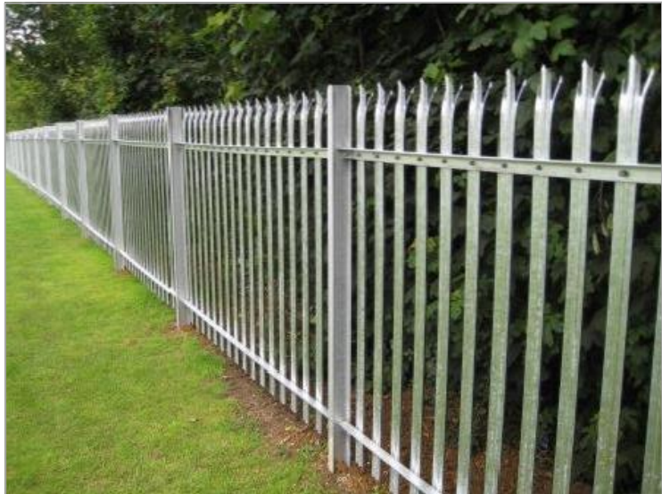
Image of Palisade Fencing
