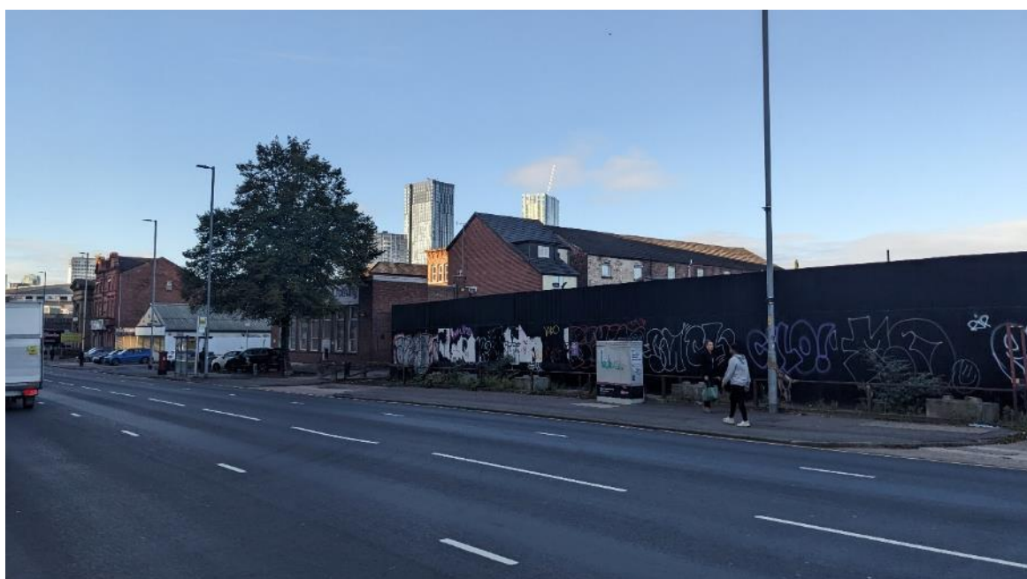
Figure 16: Looking south-west along Cheetham Hill Road showing the graffiti-ridden hoarded site boundary and surrounding multi-phase development.
