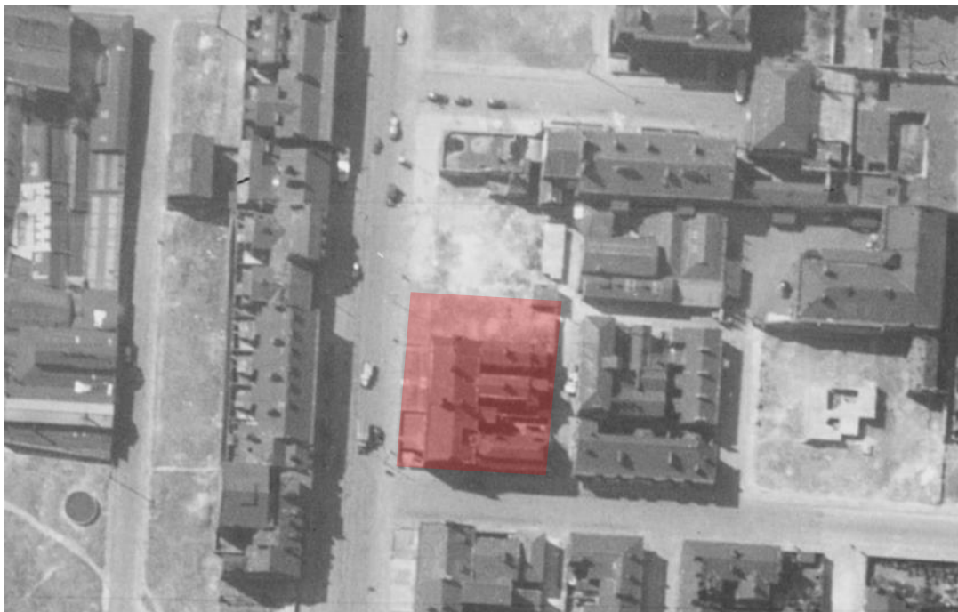
Figure 12: An aerial view looking south across the Site in 1946 showing that the southern two terraced houses (top) have been demolished and site remains cleared. (Source: Britain From Above)
