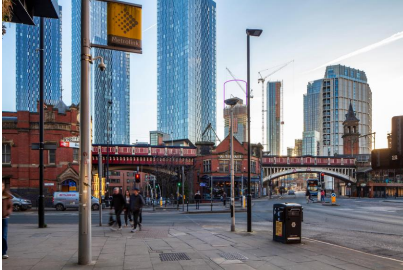
View 10 – Existing view looking south west along Deansgate
