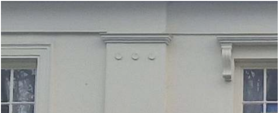
Detail of Rose Ornament at Pilaster Heads
