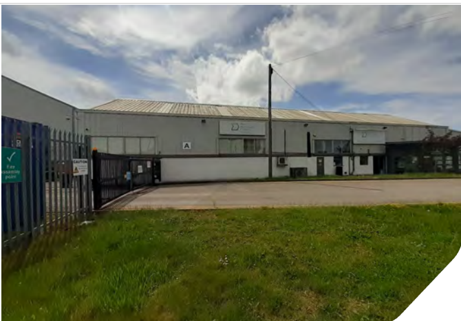
Photo 02: View of the Manchester School of Building from the north
