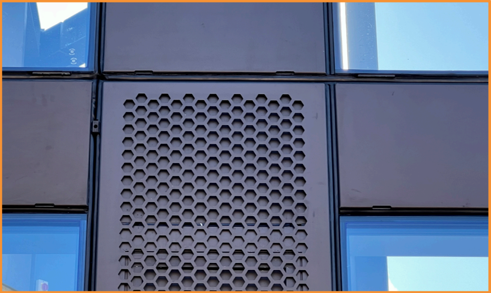
VMU - TOWER FACADE WITHOUT FINS
