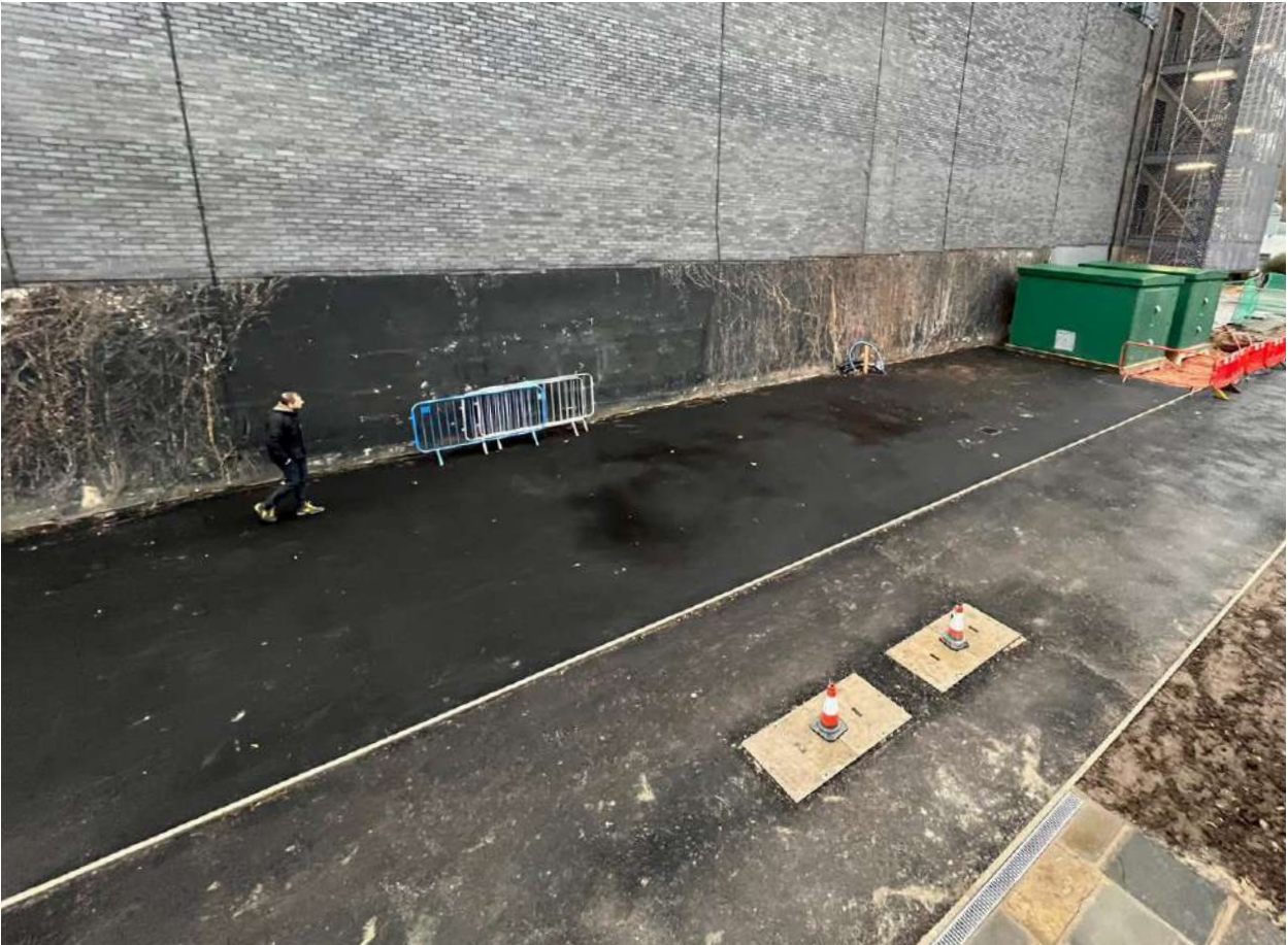
View looking east, showing the existing substations (Feb 2024)
