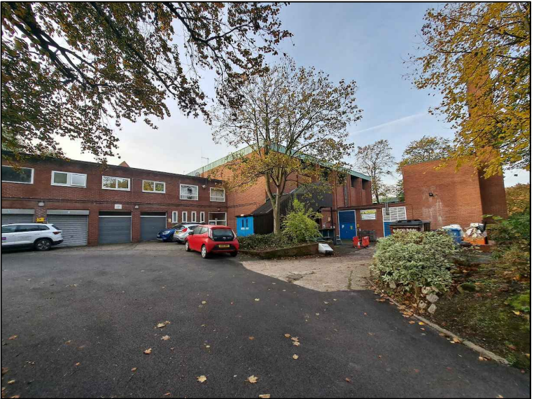
Photo 5. Standing on Oxford Place looking at Accommodation Block & Dining Hall - Roof access ladder C would be visible. Handrails on dining room would be obscured. Handrails on staff accommodation would be partly visible.
