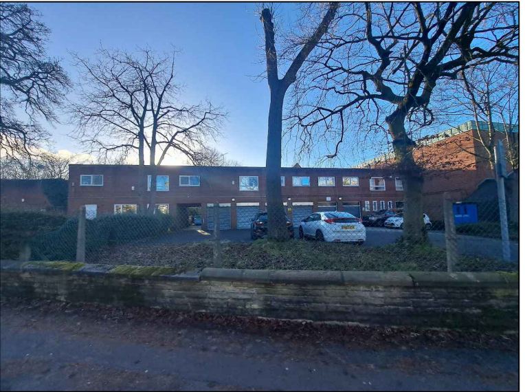
Photo 6. Standing on Oxford Place looking at Accommodation Block - Roof access ladder C would be obscured. Handrails on dining room would be obscured. Handrails on staff accommodation would be partly visible.
