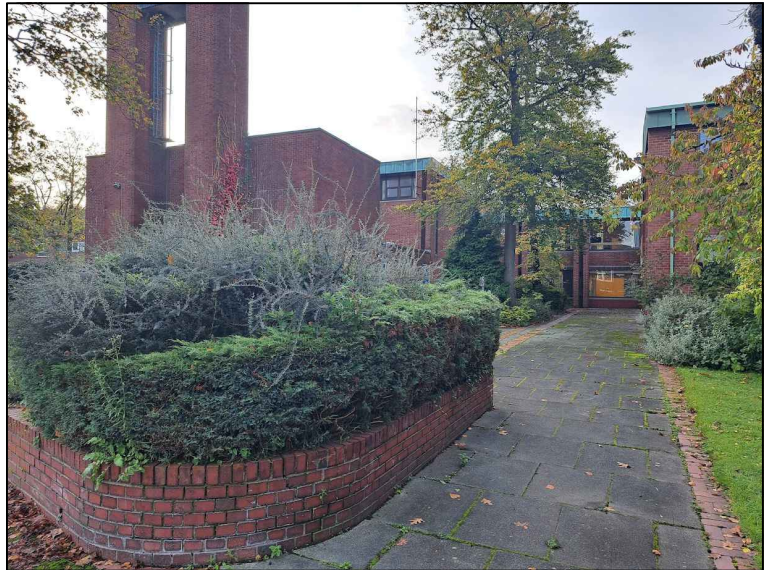
Photo 2. Standing on Oxford Place looking at Dining Hall - Roof access ladder D would not be visible. External roof access ladder A would be obscured. Handrails on dining room would be mostly obscured by the trees and plant room 2nd storey roof.
