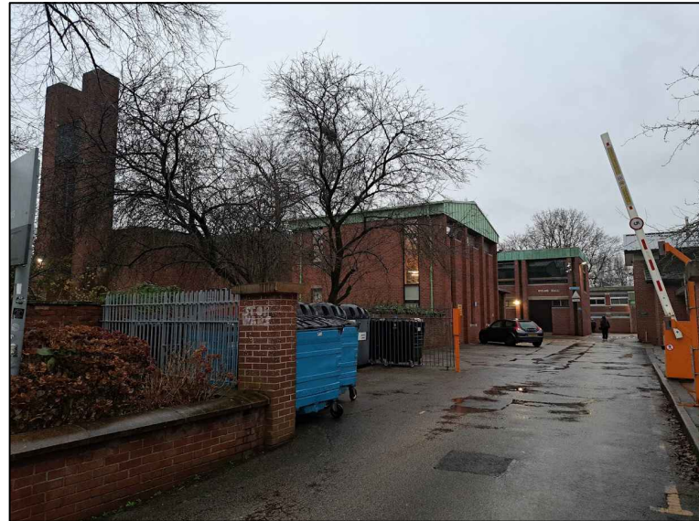
Photo 1. Standing on Oxford Place looking towards Main entrance - Roof access ladder E would not be visible. Handrails on dining room would be obscured.
