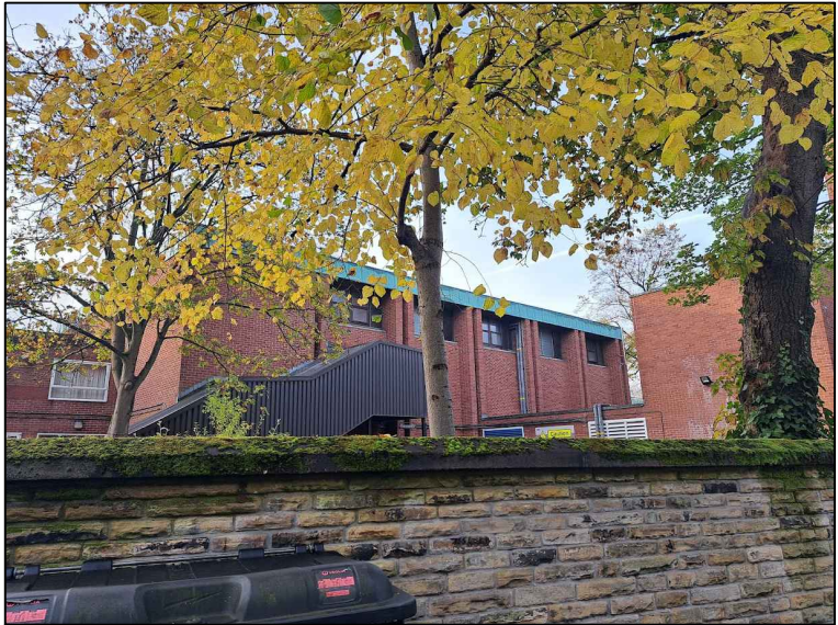
Photo 4. Standing on Oxford Place looking at Dining Hall - Roof access ladder C would be obscured. Handrails on dining room would be obscured.
