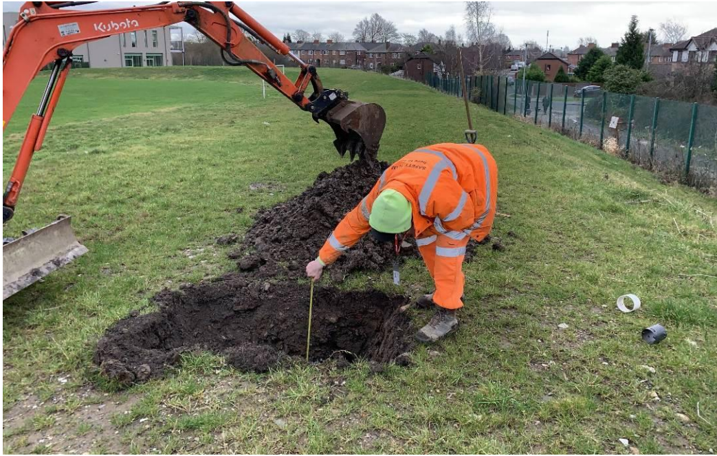
Above and below – trial pit on the spoil mound, proposed 3G STP south-western corner.
