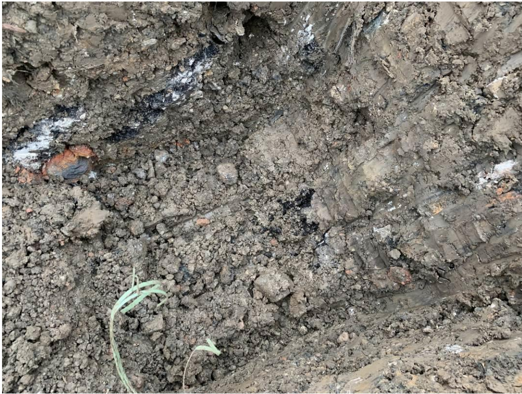
Spoil mound – clay mixed with brick, macadam, concrete, plastic, etc.
