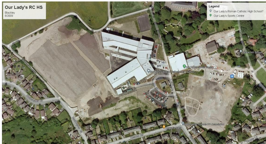
Old school demolished, new school constructed, topsoil being re-laid over the playing field area, 2009
