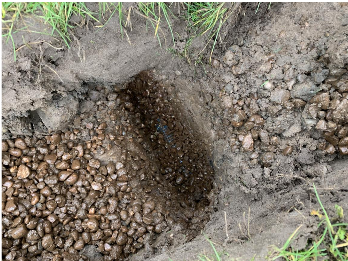
80mm uPVC corrugated plastic land drains at 5-metre centres over part of the playing field
