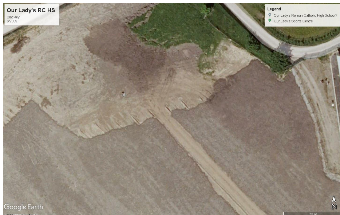
Drainage trenches in the fill material, installed prior to topsoiling, Approximately 5-metre centres, apparently not extending fully to Pitch A
