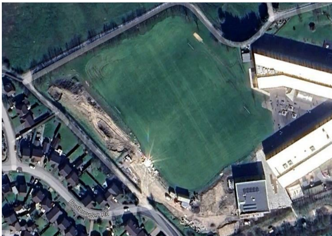
The playing field area in early 2023, new extension building work underway, spoil mound created from the building foundations on the western boundary.
