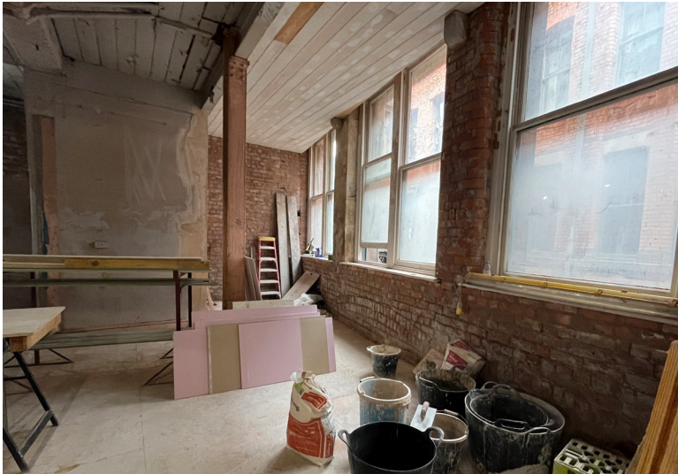
First Floor no 14- CAT works ongoing in accordance with extant consent
