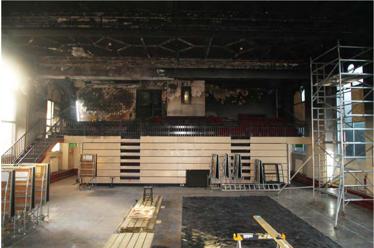
Plate 18. Hall, showing balcony with raked seating under, viewed from north.
