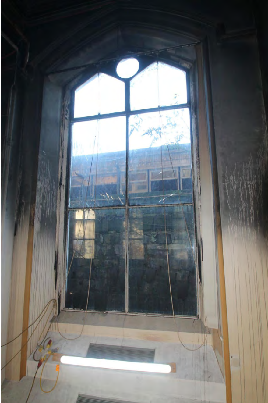
Plate 19. Window on west side of Hall, bay 4, viewed from east.
