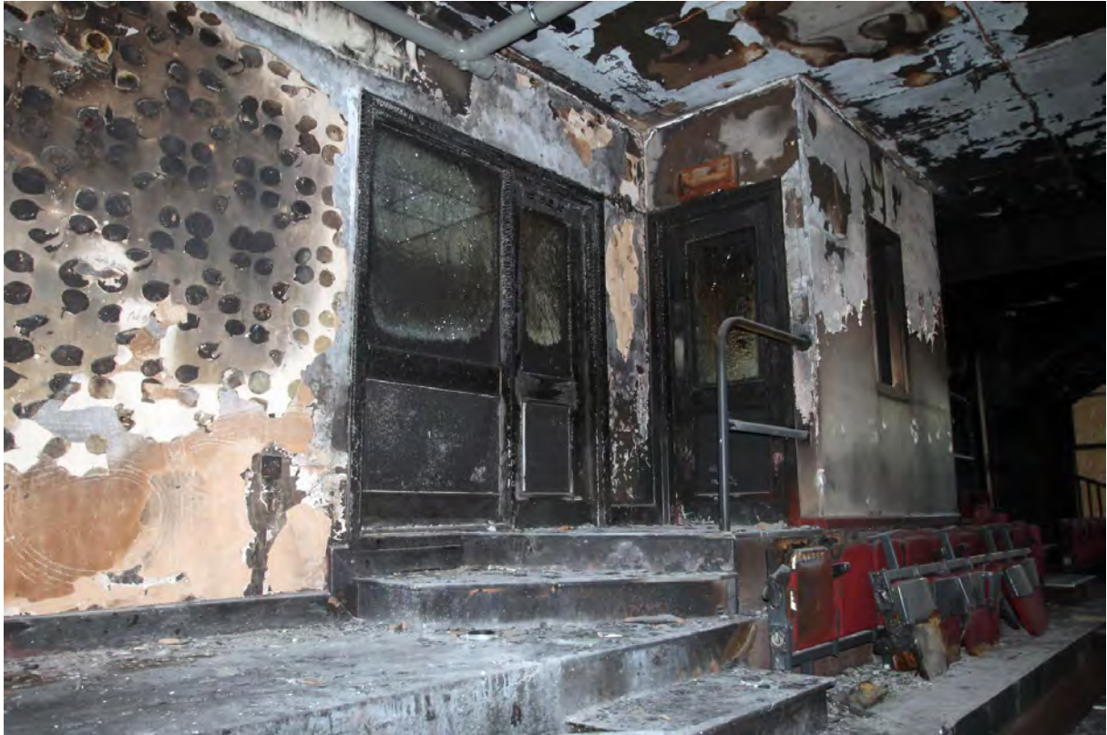
Plate 27. Balcony, bay 1, viewed from east.
