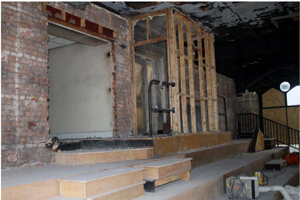
Plate 48. South wall of balcony, viewed from north-east, showing inserted doorway.
