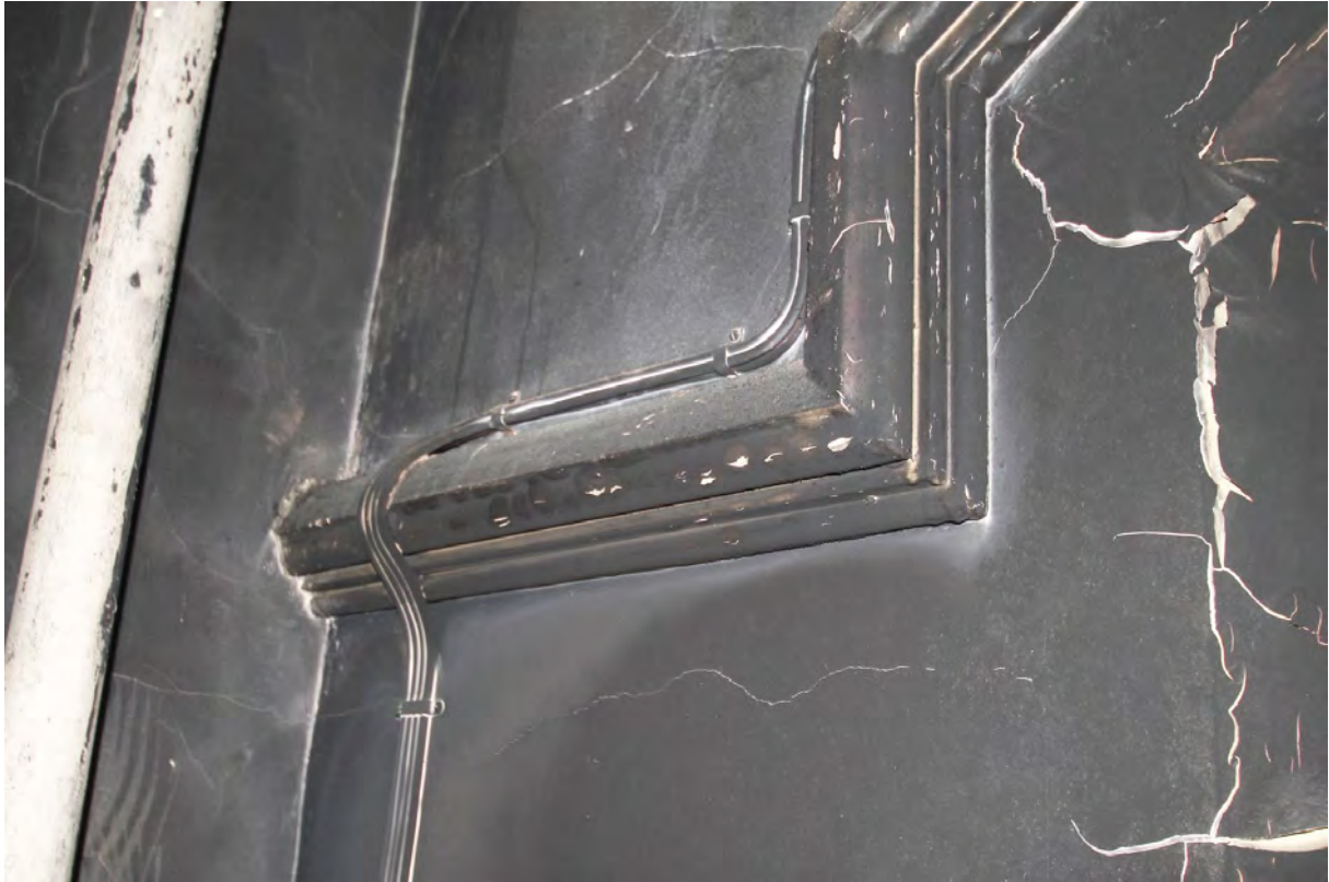
Plate 32. Plaster moulding around window, west elevation, bay 1, viewed from north-east.
