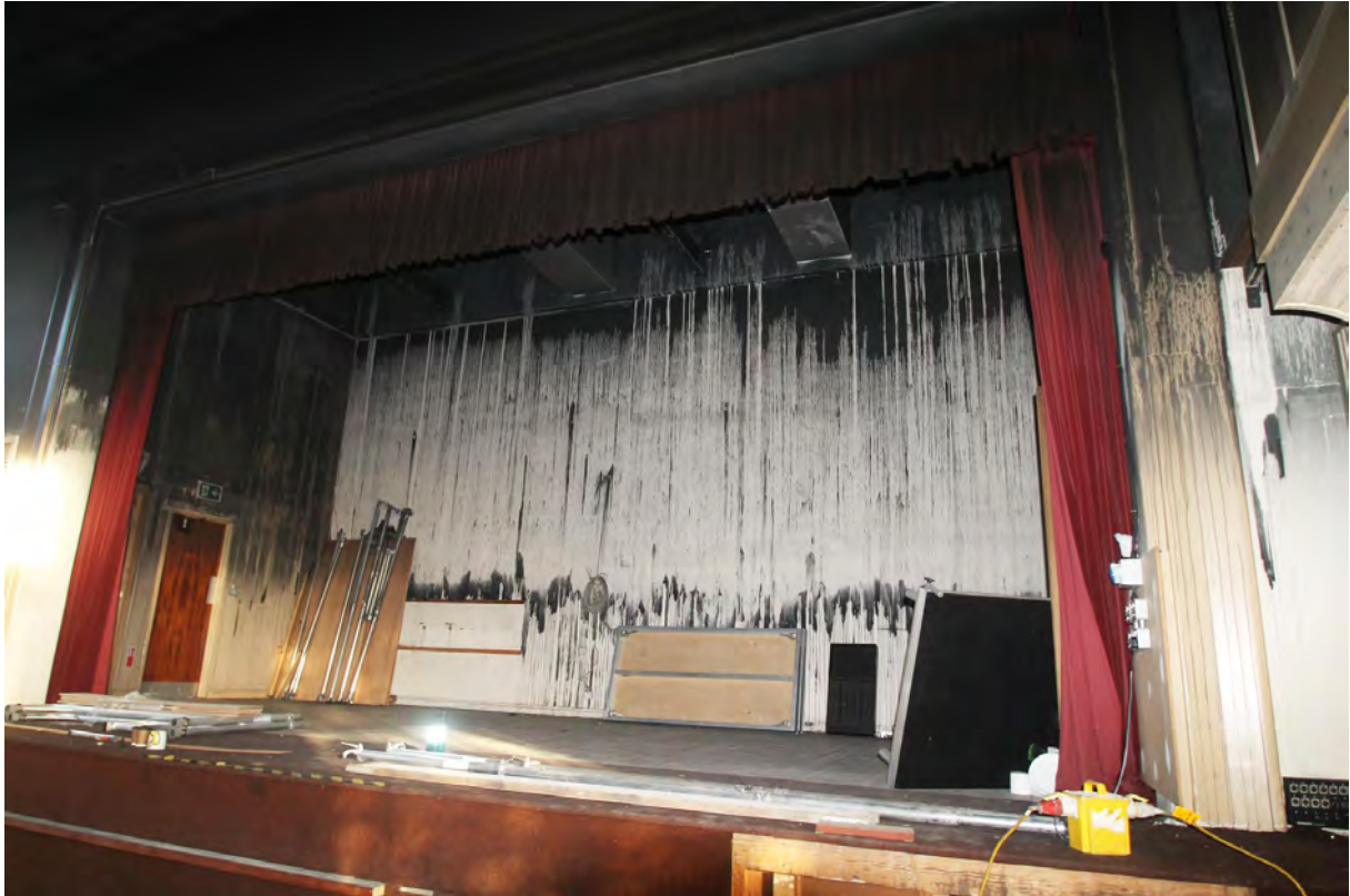
Plate 7. Stage, viewed from south-east.
