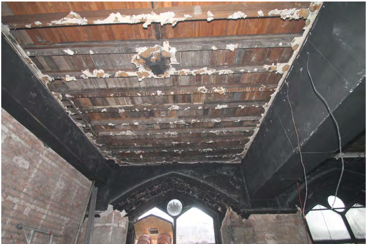
Plate 58. Bay 1, following removal of later plasterboard ceiling, viewed from east.
