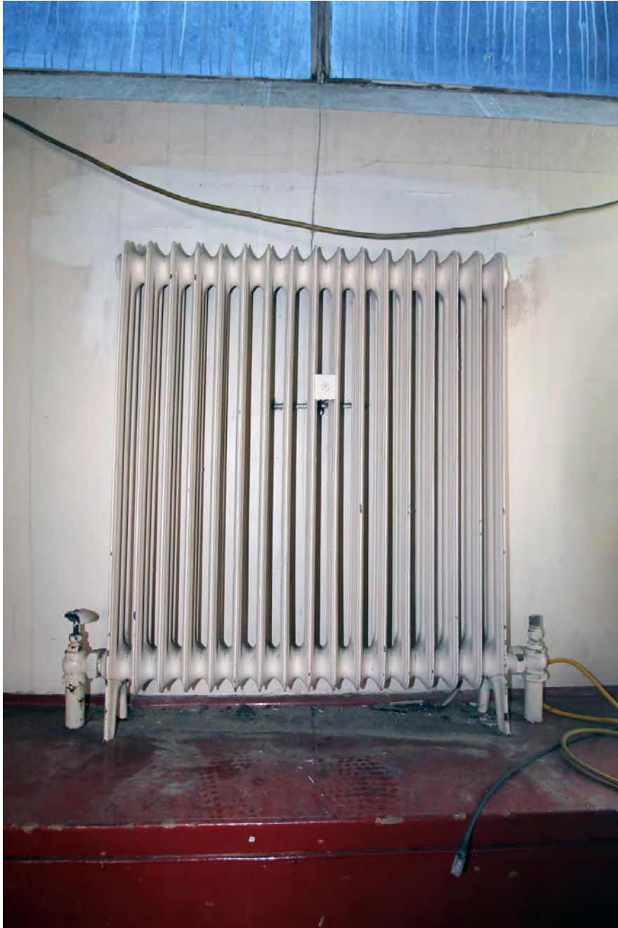
Plate 21. Radiator before removal, bay 3, viewed from east.
