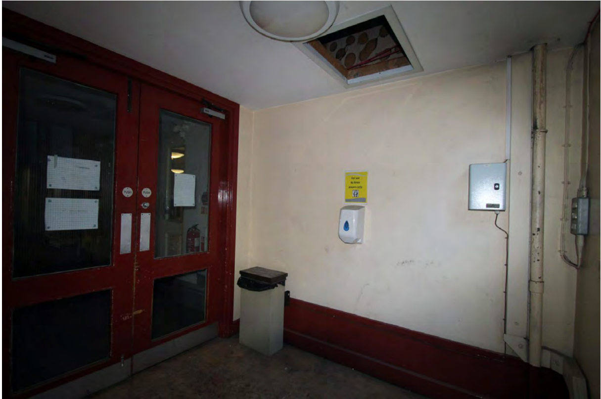
Plate 23. Corridor in bay 1, viewed from north-west.
