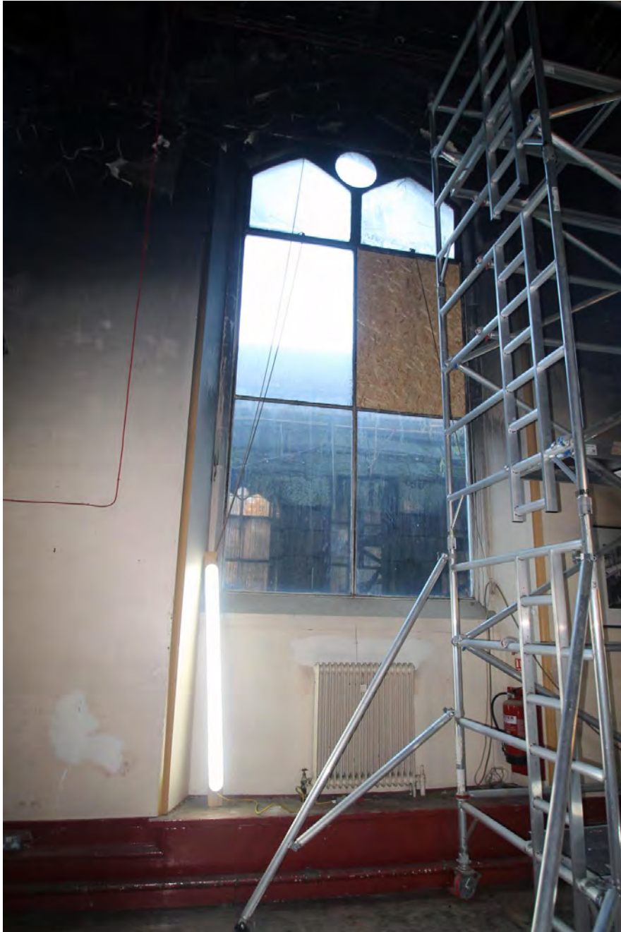
Plate 22. Window, west side of Hall, bay 2, viewed from east.
