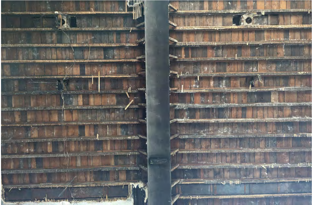
Plate 59. Ceiling of bays 2 and 3, following removal of plasterwork. Viewed from below.
