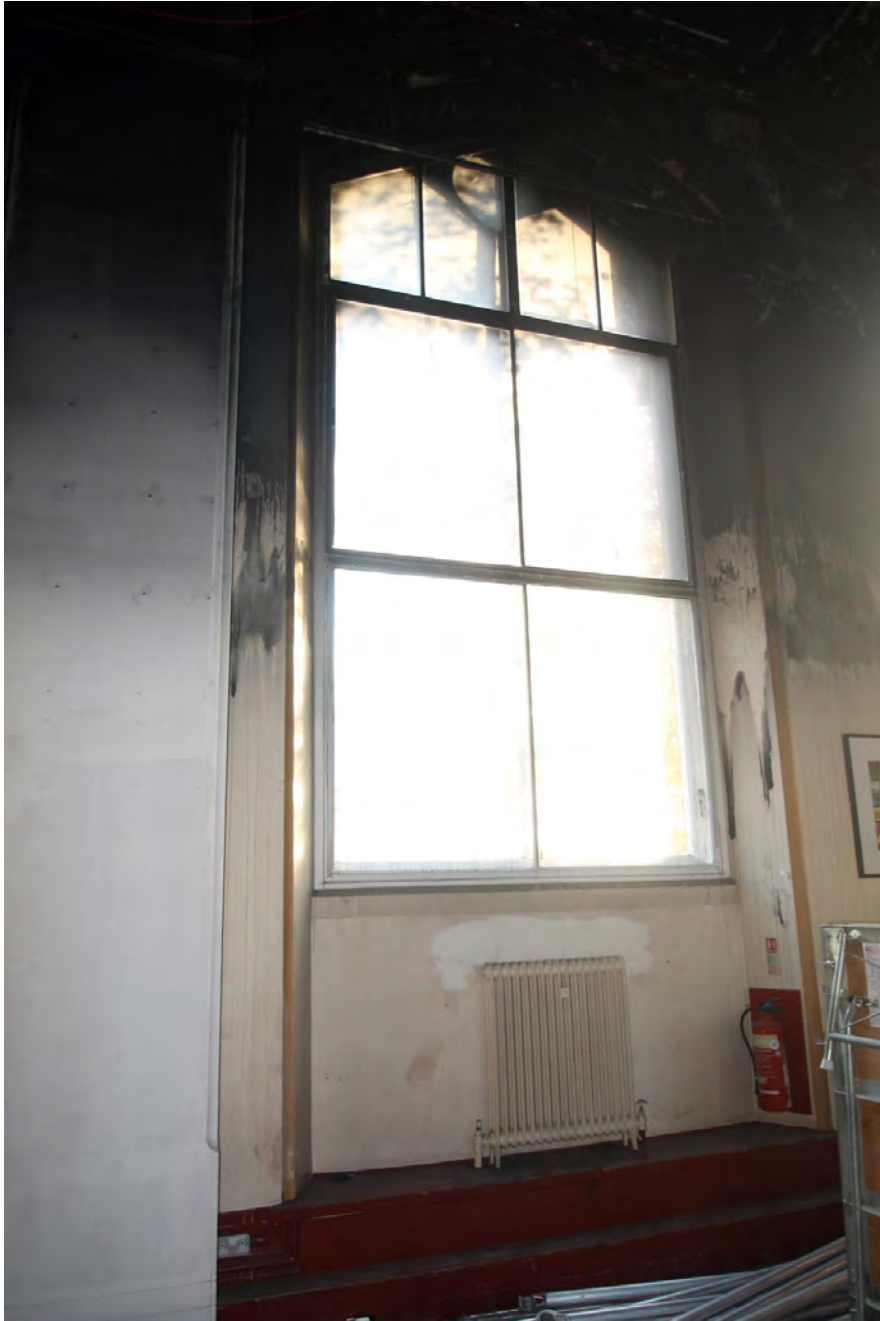
Plate 25. Window in east elevation, bay 3, viewed from north-west.
