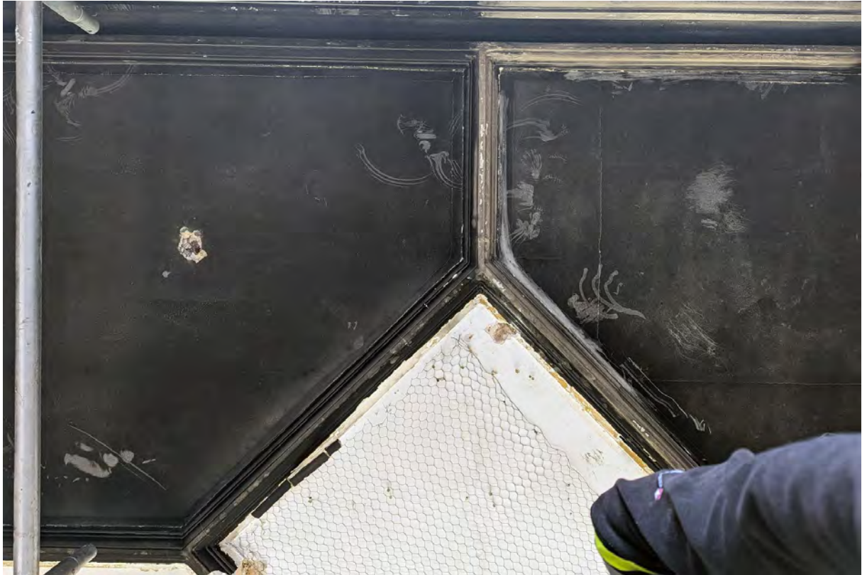
Plate 57. Intact plasterwork ceiling panels, bay 2, west side. Viewed from below.
