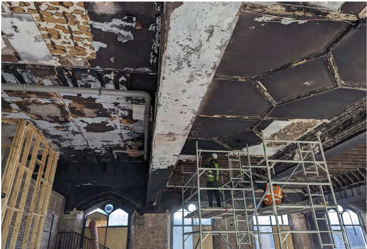
Plate 46. Ceiling removal within bay 2, viewed from east.
