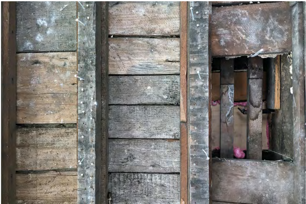
Plate 60. Ceiling of bay 2, following removal of plasterwork. Floor over seen through gap.
