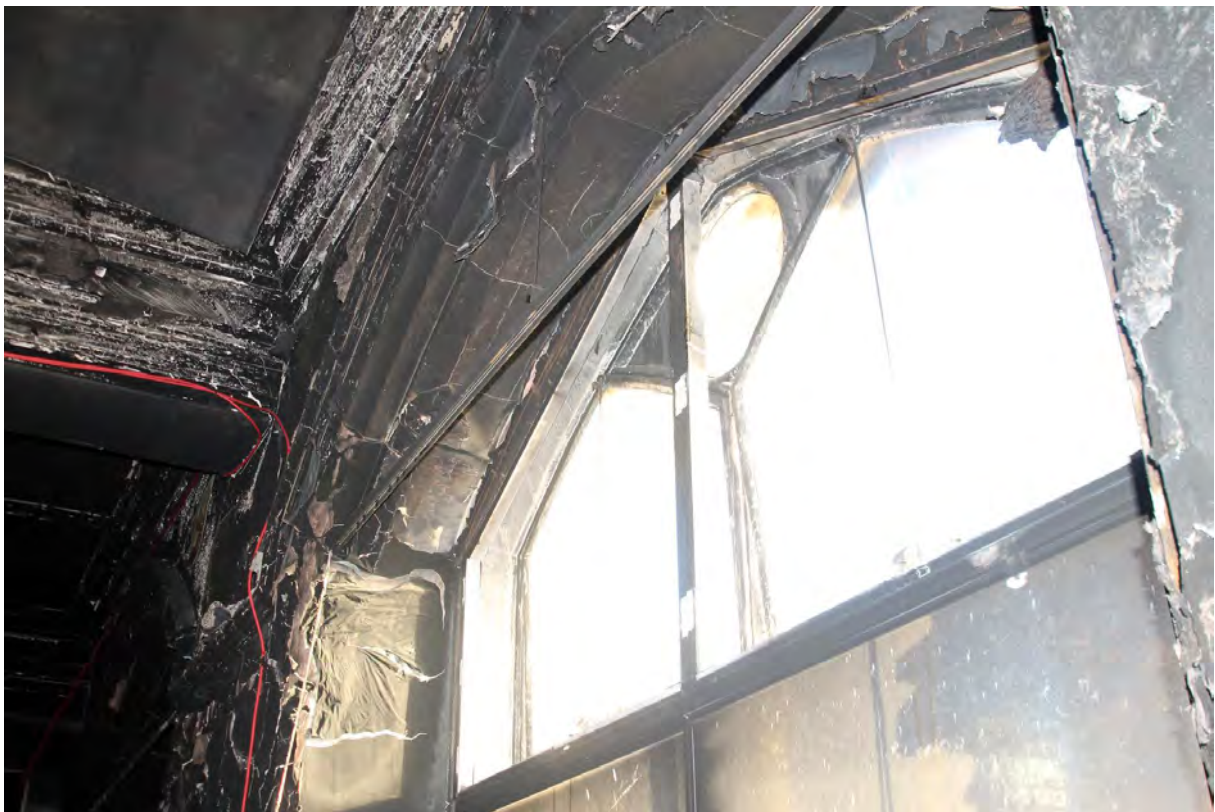
Plate 37. Window, east elevation, bay 2, viewed from south-west.
