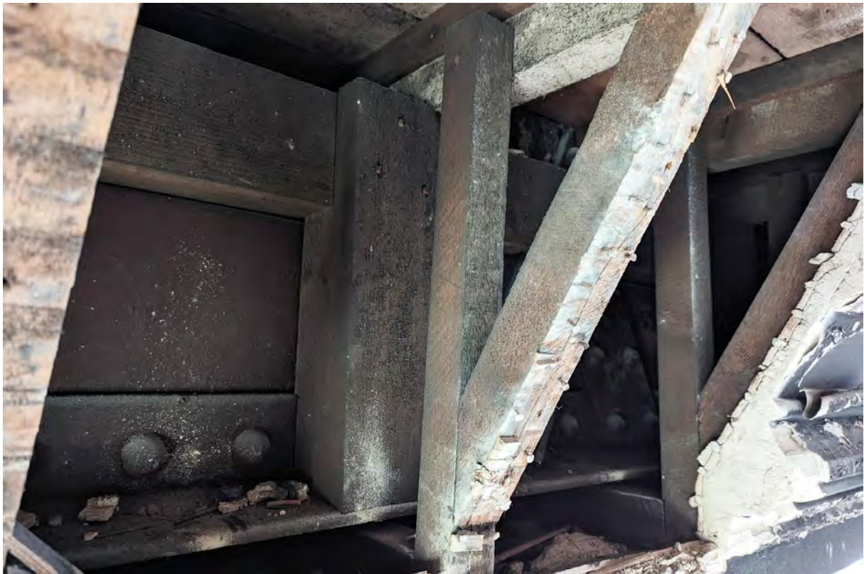
Plate 56. Wrought iron beam, bay 2, viewed from north-east, showing timber formwork.
