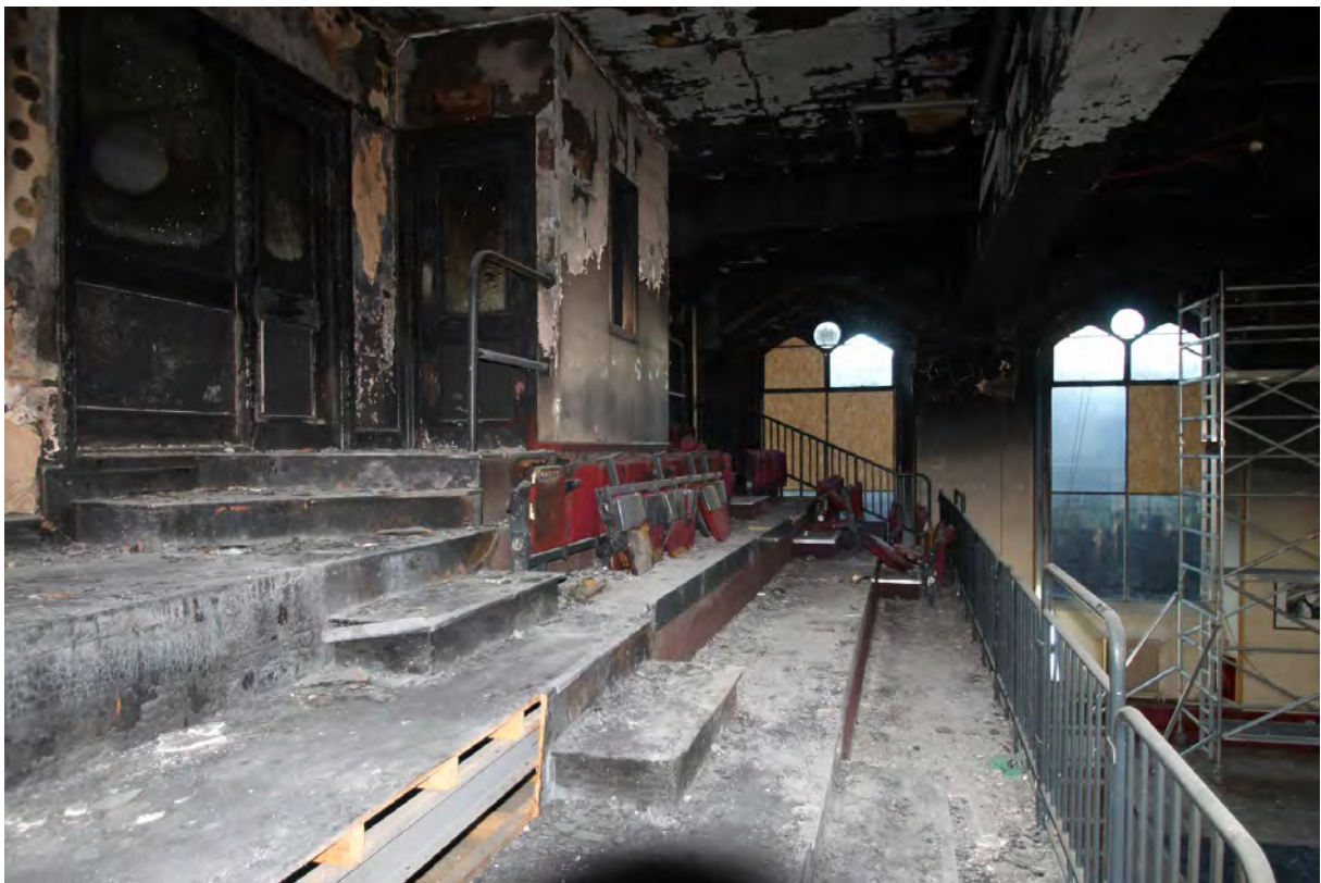
Plate 28. Balcony, bay 1, viewed from east.
