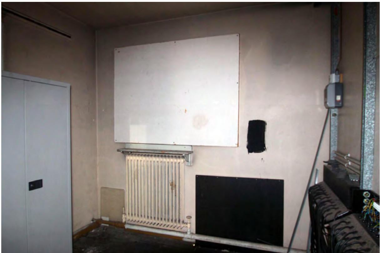
Plate 15. Stage, east side, store, viewed from west.
