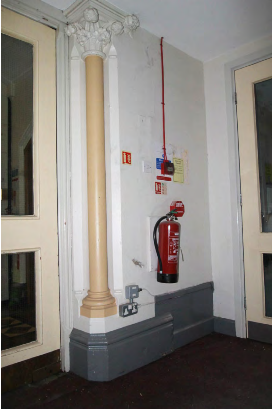
Plate 42. Corridor beneath balcony, bay 1, column detail, viewed from north-east.
