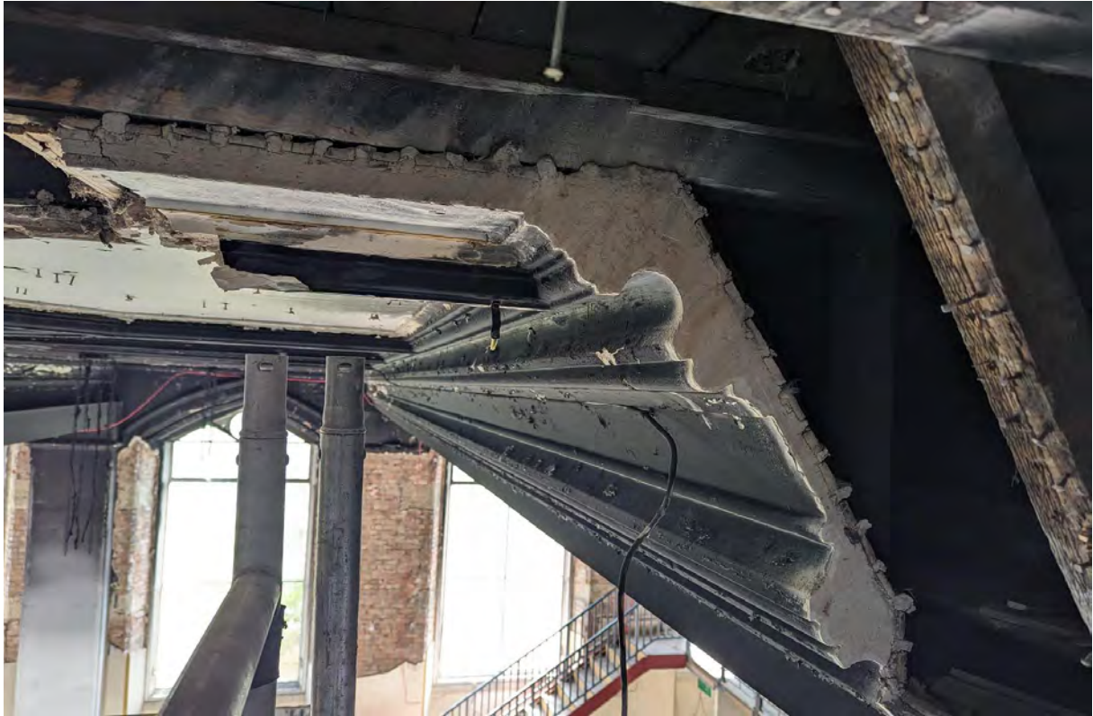
Plate 53. Cut section of plasterwork ceiling, bay 3, south side, viewed from east.
