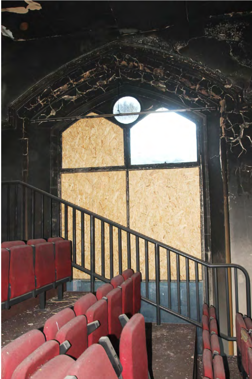
Plate 29. Window in bay 1, viewed from east, from balcony.
