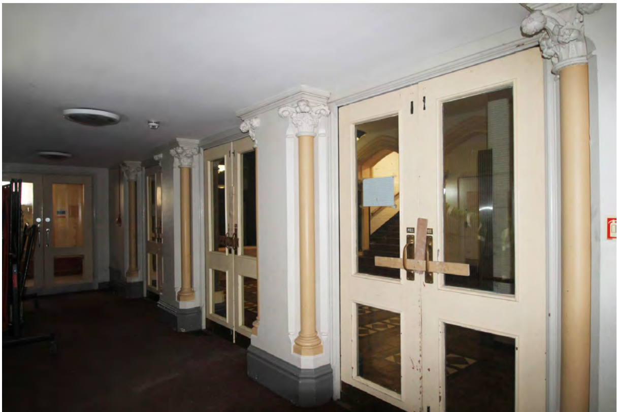
Plate 41. Corridor beneath balcony, bay 1, viewed from west.
