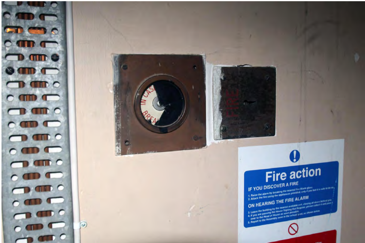
Plate 16. Stage, east side, store, fire alarm, viewed from north.
