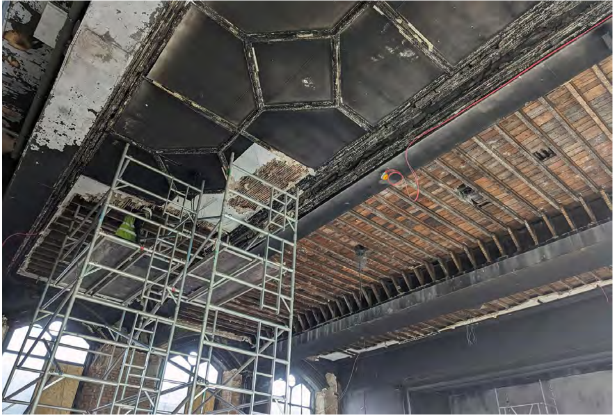
Plate 45. Ongoing ceiling removal within bay 2, viewed from south-east.
