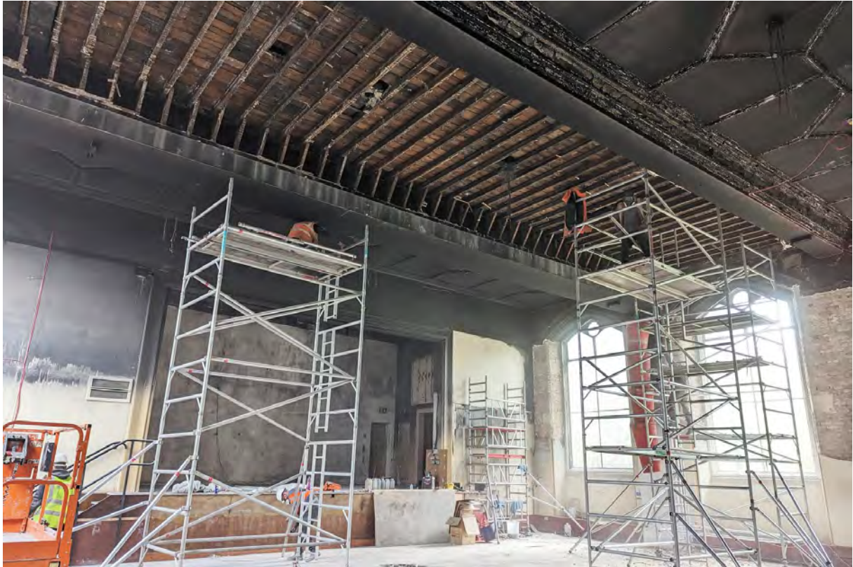
Plate 43. Ongoing ceiling removal within bay 2, viewed from north-east.
