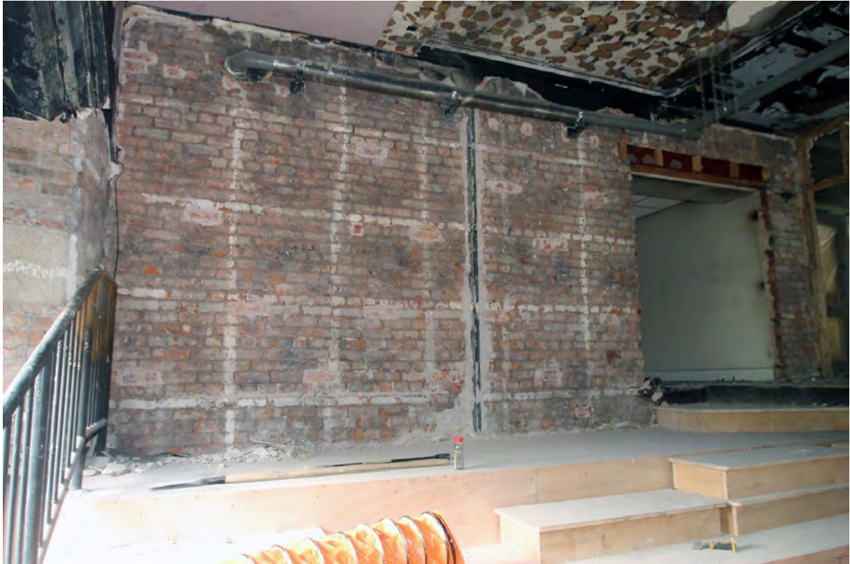
Plate 47. South wall of balcony, following removal of dry lining, viewed from north.
