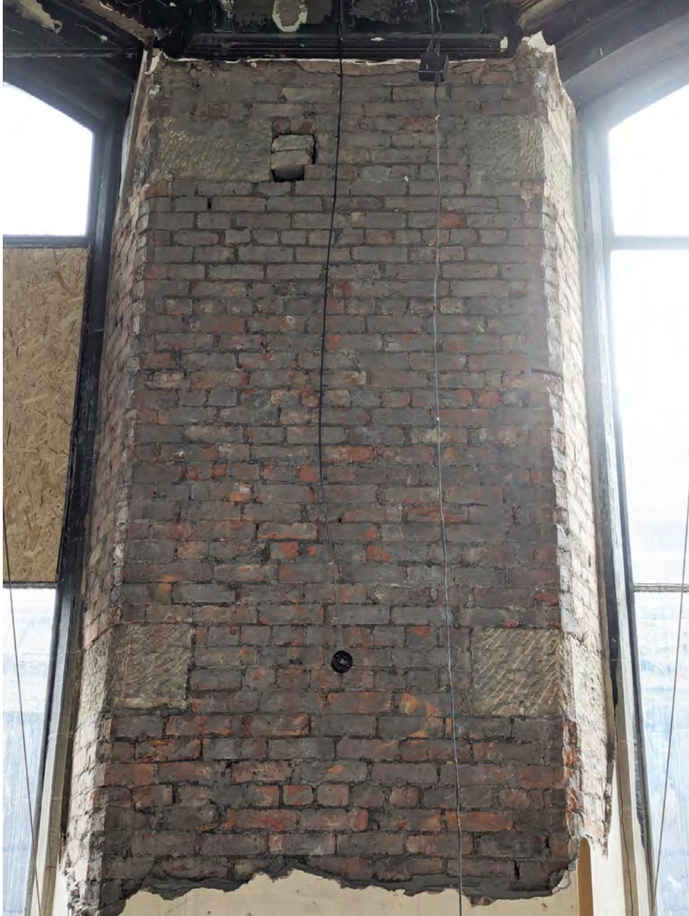
Plate 50. East elevation, between bays 2 and 3, following plaster removal.
