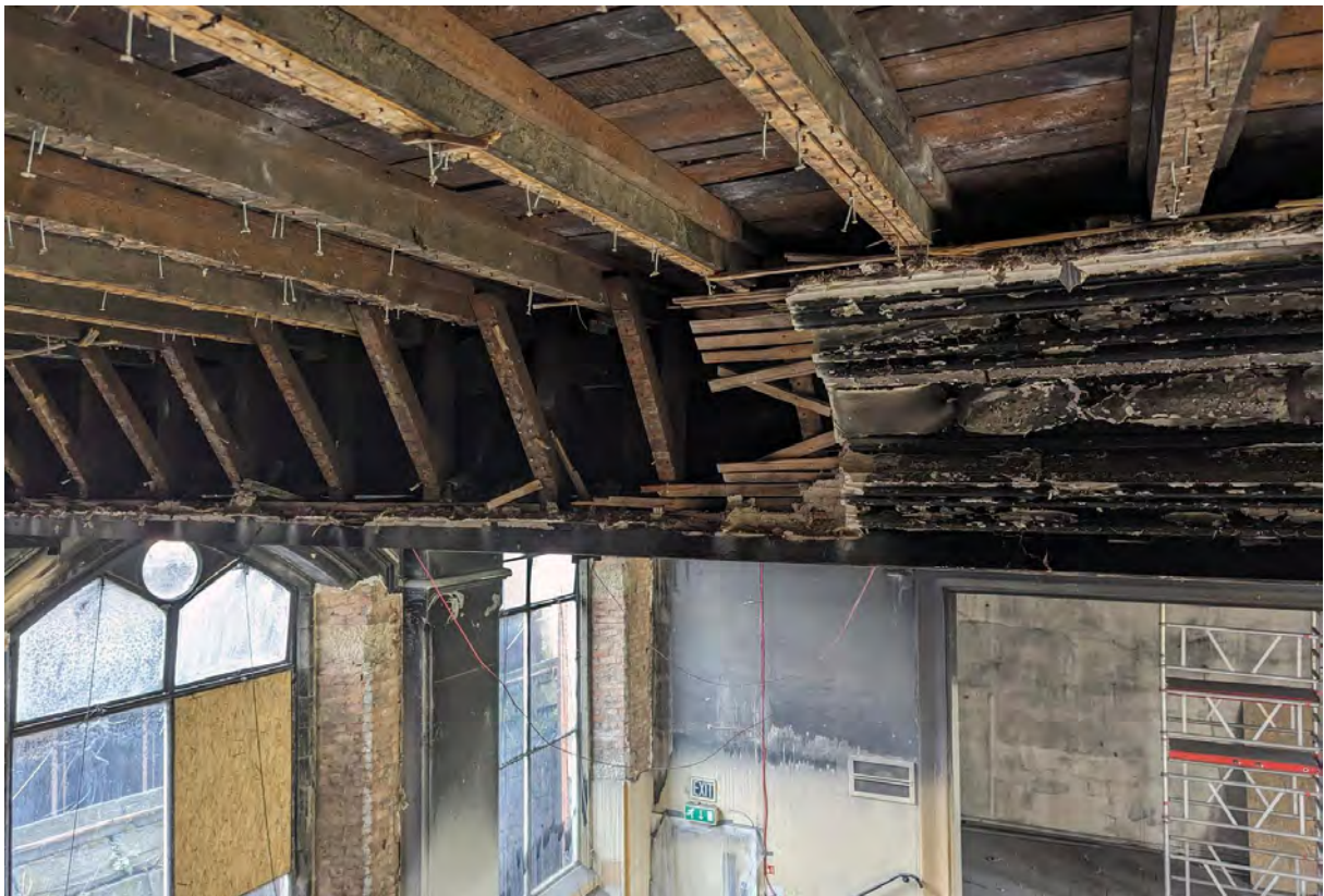
Plate 52. Beam with lathe & plaster being removed, between bays 2 & 3, viewed from south.
