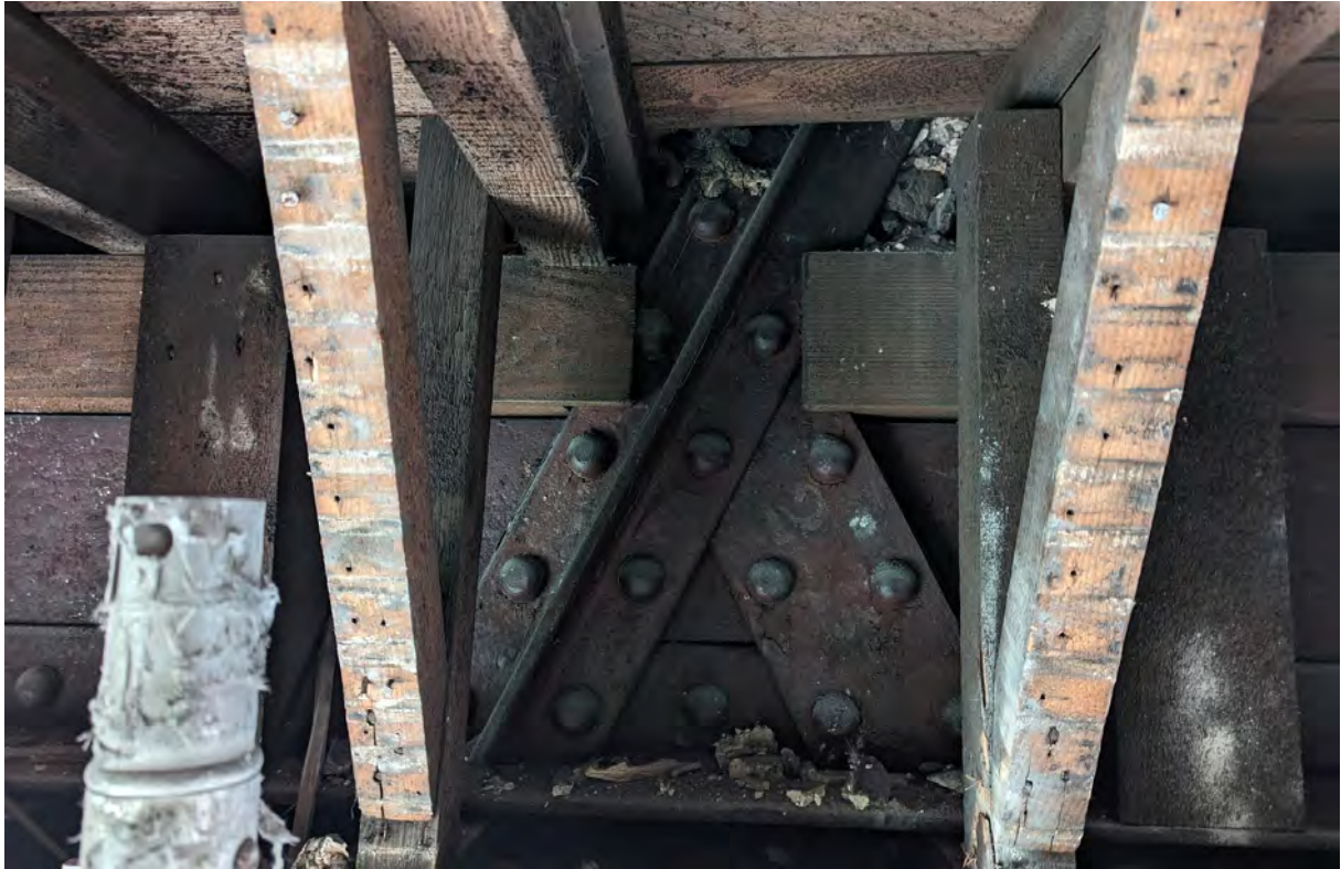
Plate 55. Wrought iron beam, bay 4, with diagonal braces, viewed from north.
