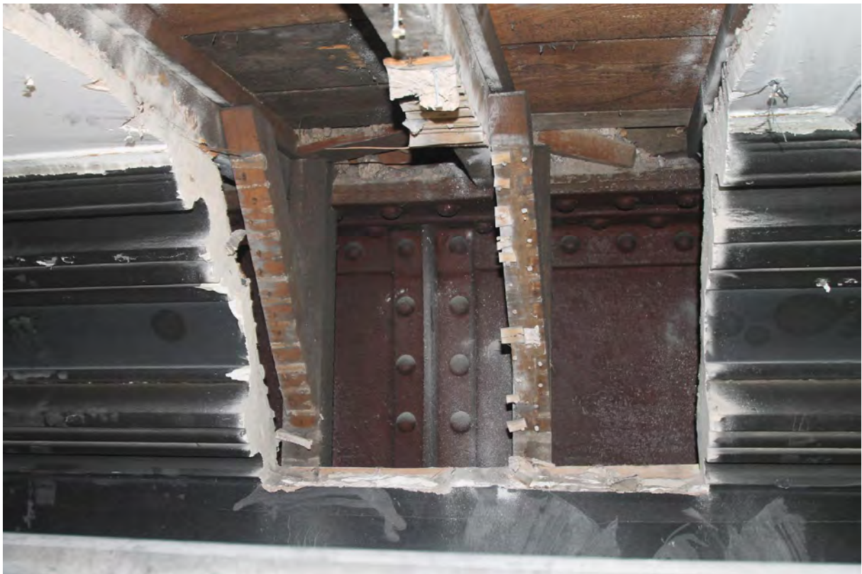
Plate 54. Plasterwork cut away to reveal wrought-iron beam, bay 3, viewed from north.
