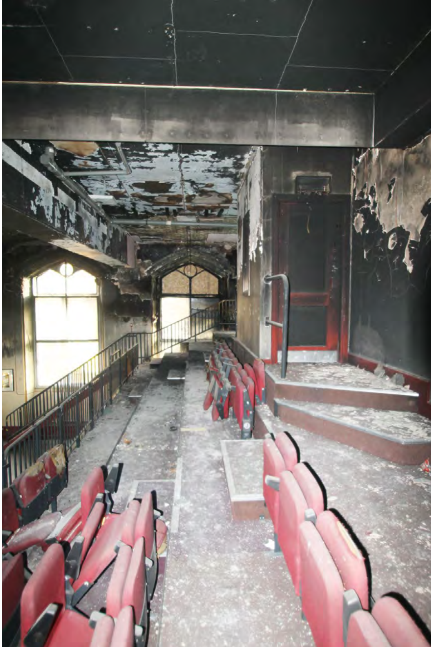
Plate 31. Balcony, bay 1, viewed from west
