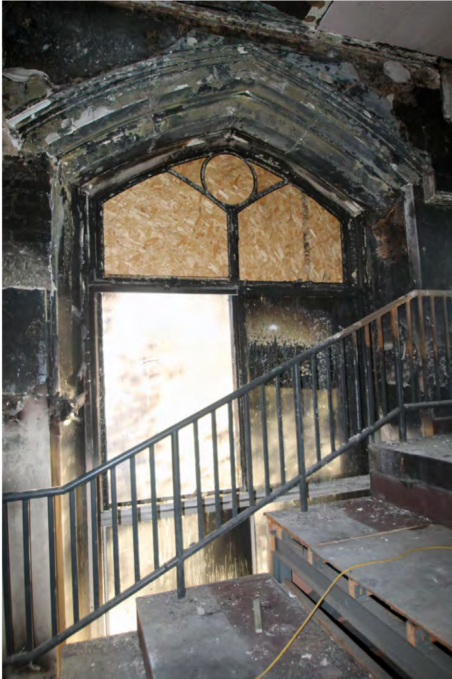
Plate 26. Window in east elevation, bay 1, viewed from west.
