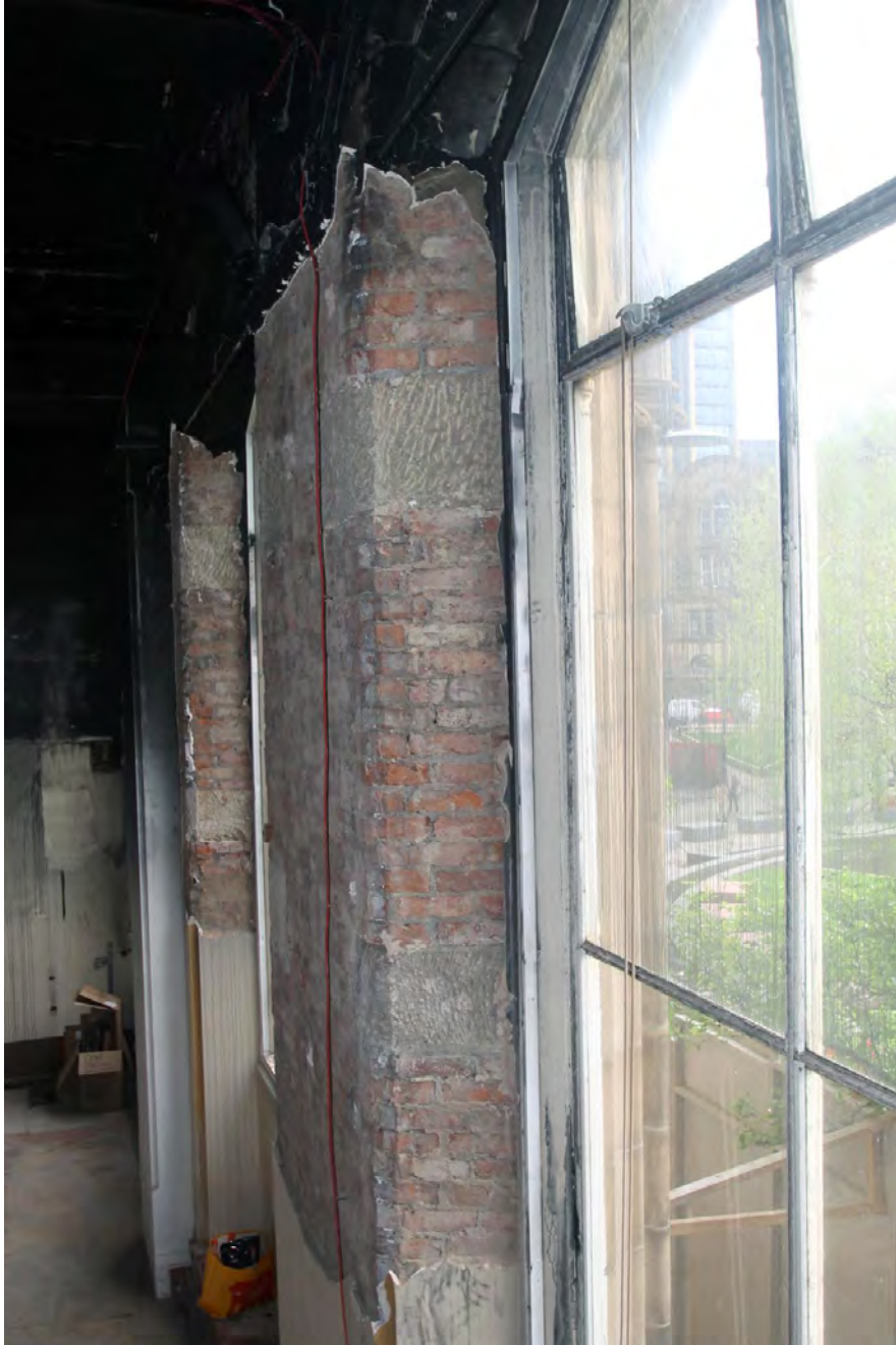
Plate 49. Window aperture, east elevation, bay 1, following plaster removal.
