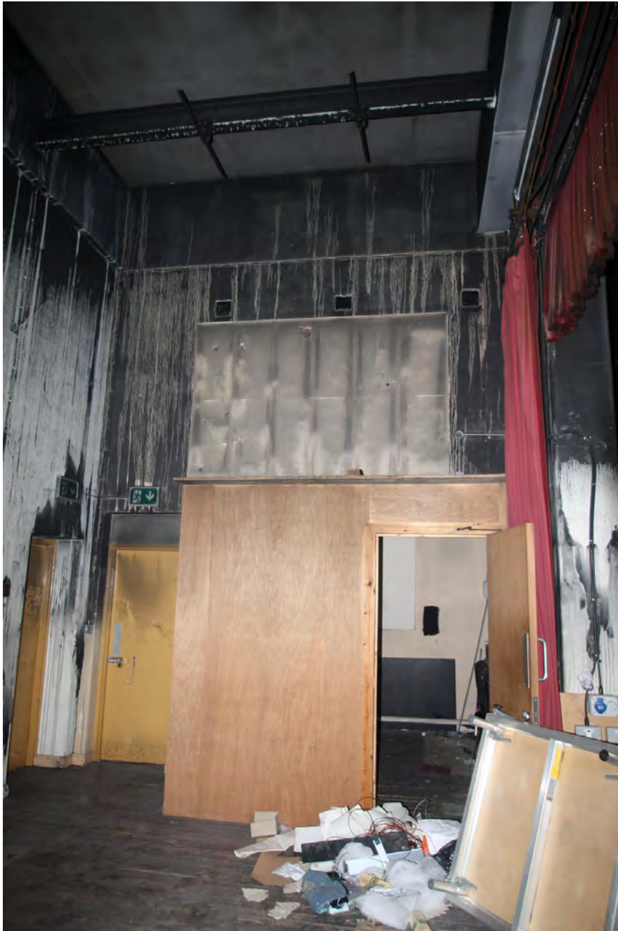
Plate 10. Stage, east side, viewed from west.
