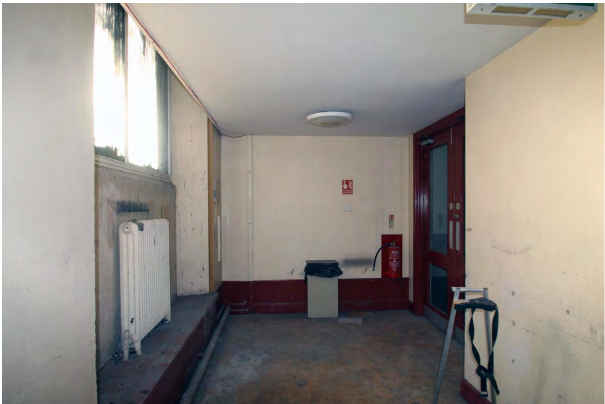
Plate 39. Corridor beneath balcony, bay 1, viewed from north.
