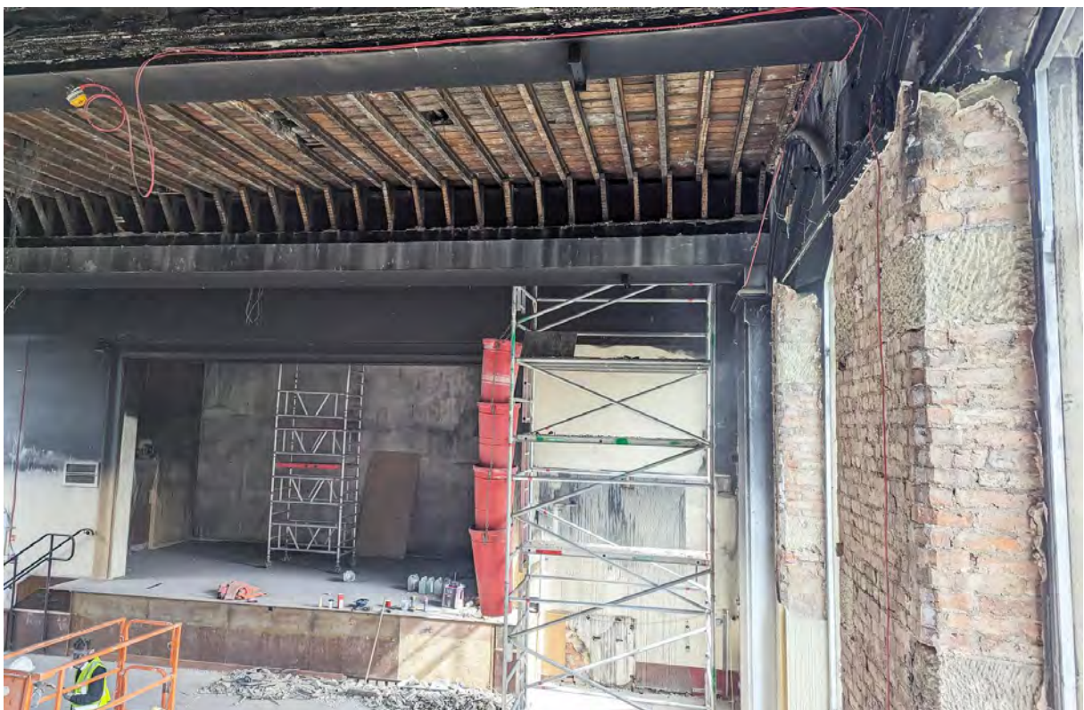
Plate 44. Ongoing ceiling removal within bay 2, viewed from south.
