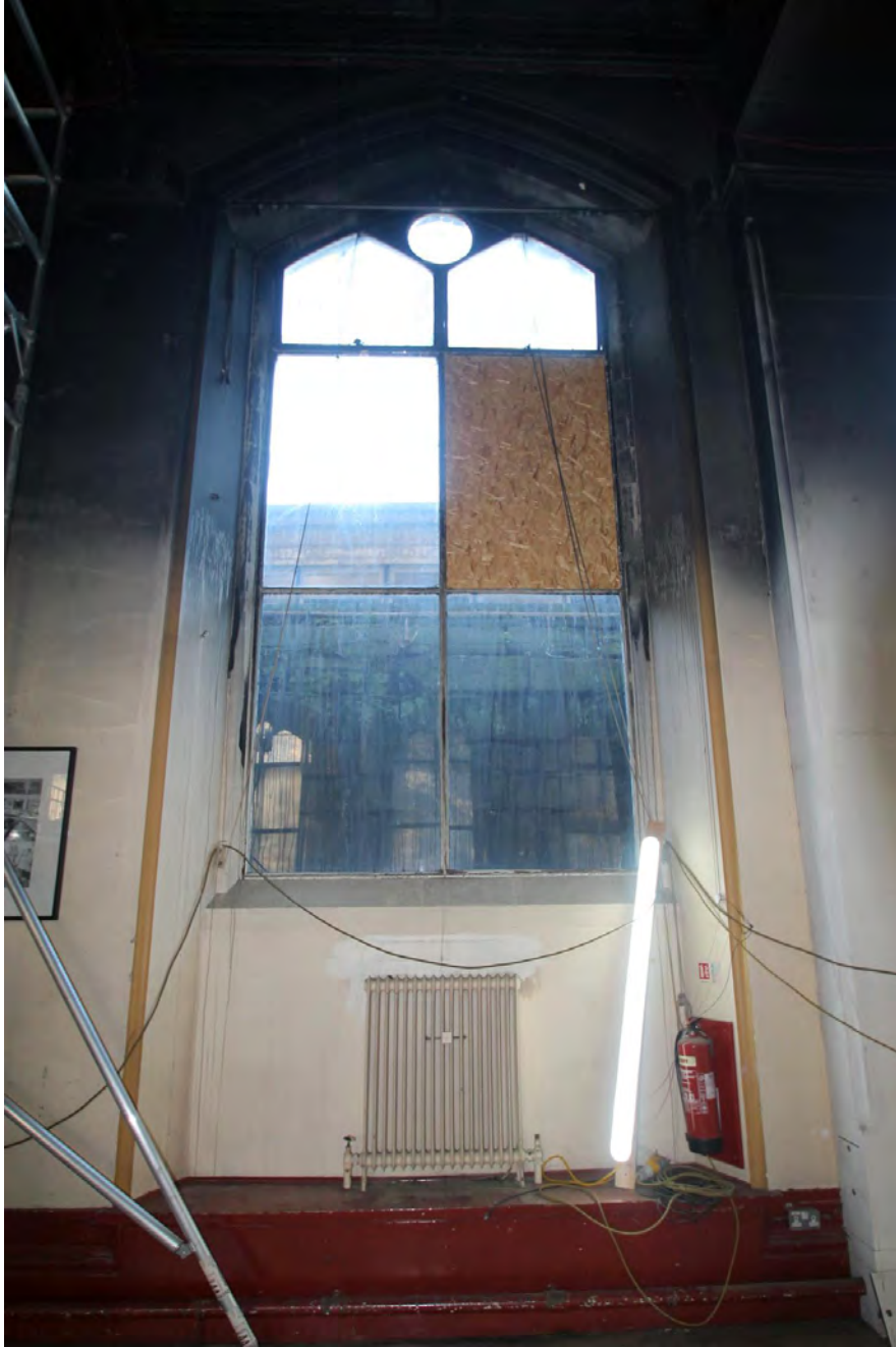
Plate 20. Window on west side of Hall, bay 3, viewed from east.
