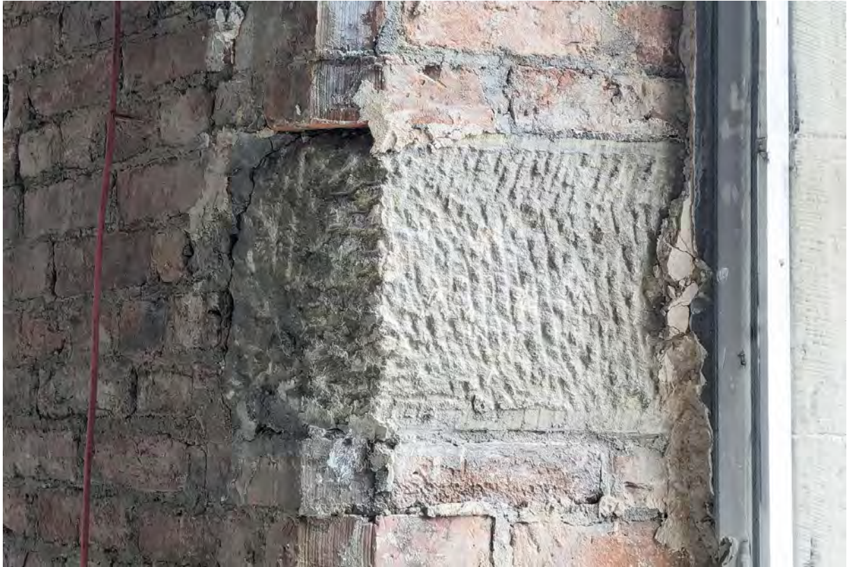
Plate 51. Gritstone block in south window reveal, west elevation, bay 2.
