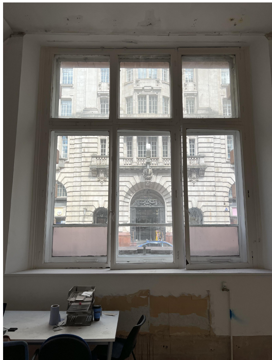
07 SECONDARY GLAZING REFERENCE 520 N/A PHOTOGRAPH EXAMPLE
