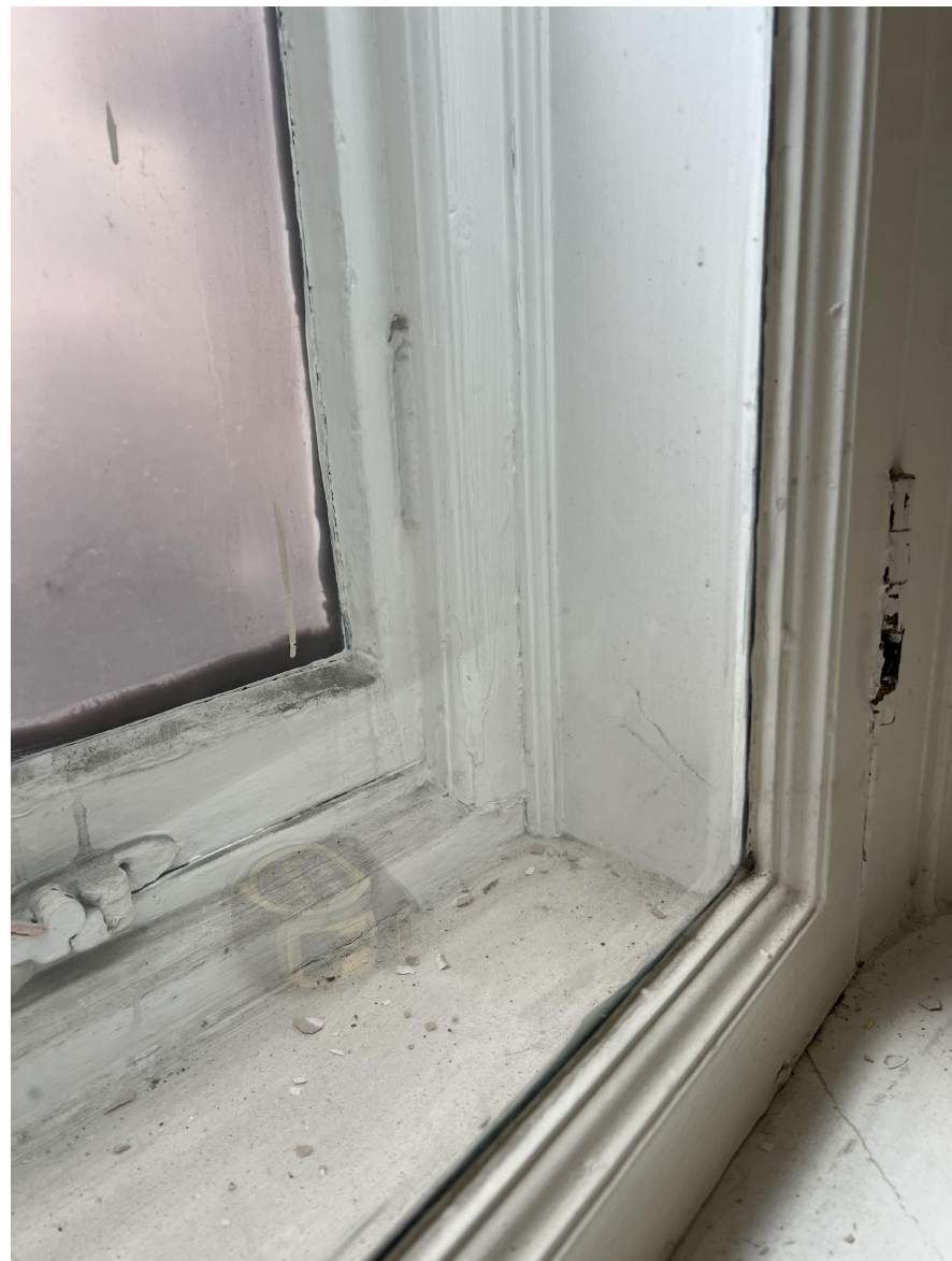
09 SECONDARY GLAZING REFERENCE 520 N/A PHOTOGRAPH EXAMPLE
