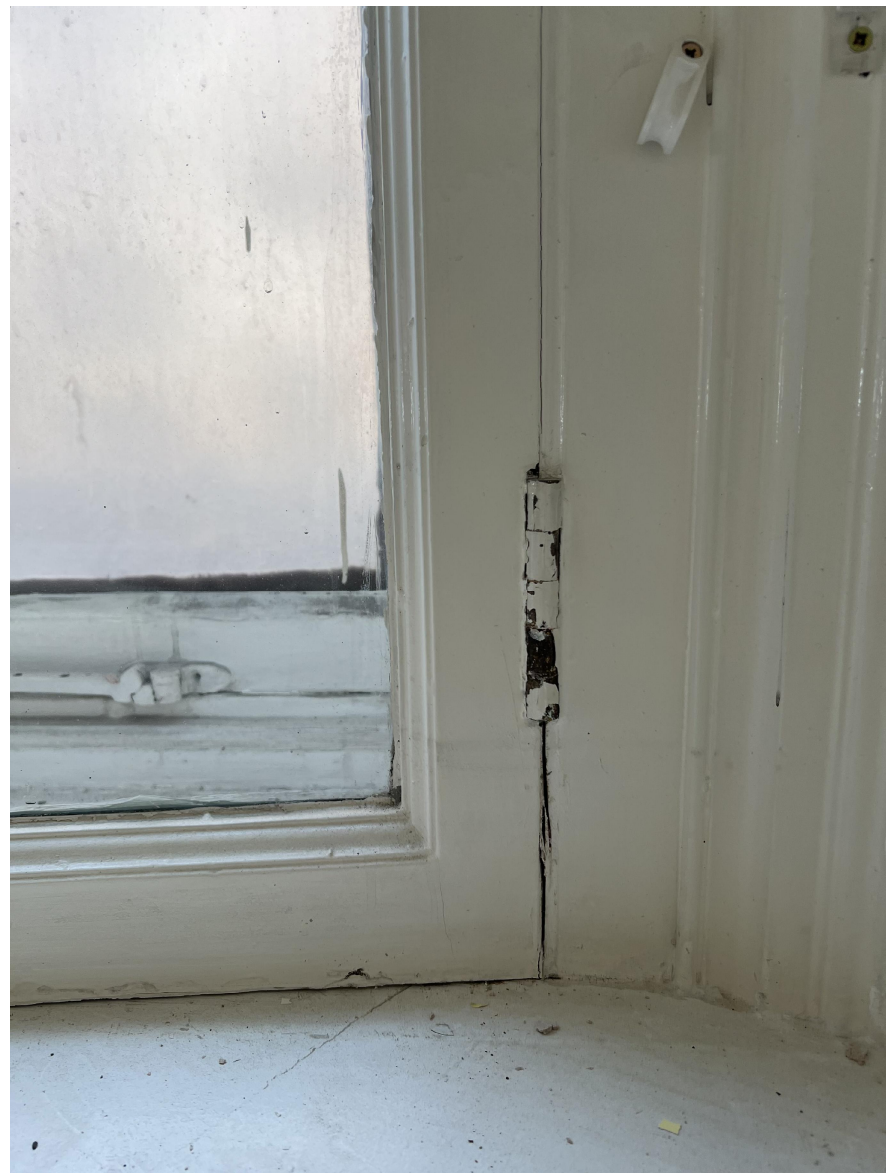
08 SECONDARY GLAZING REFERENCE 520 N/A PHOTOGRAPH EXAMPLE
