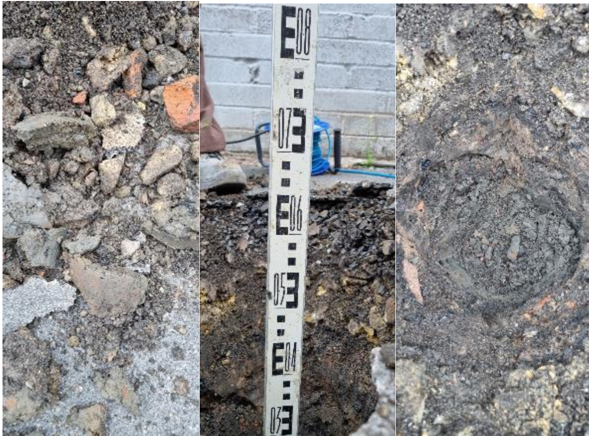
Trail Pit 3 – Front left side of site
