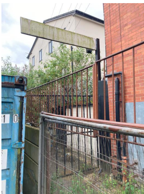
Photo 4: View of fencing at rear of 50 Bury New Road.
