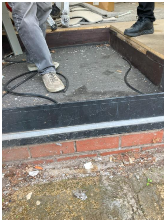
Photo 2: Photo showing steps into the commercial ground floor.
