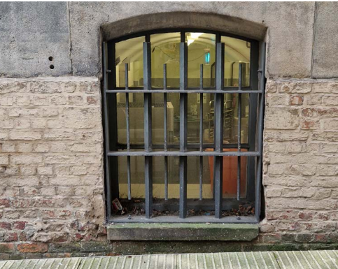
Figure 33 Existing security bars installed on the Grade I listed Art Gallery building
