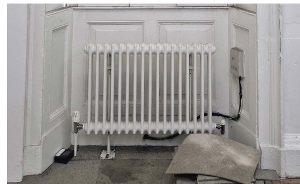
Figure 21 Photograph showing existing modern radiators
