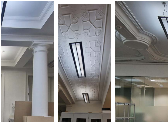
Figure 25 Photographs showing historic ceiling types (Left: Lath and plaster, Middle: Lath and Plaster decorative panels, Right: Fibrous Plaster)
