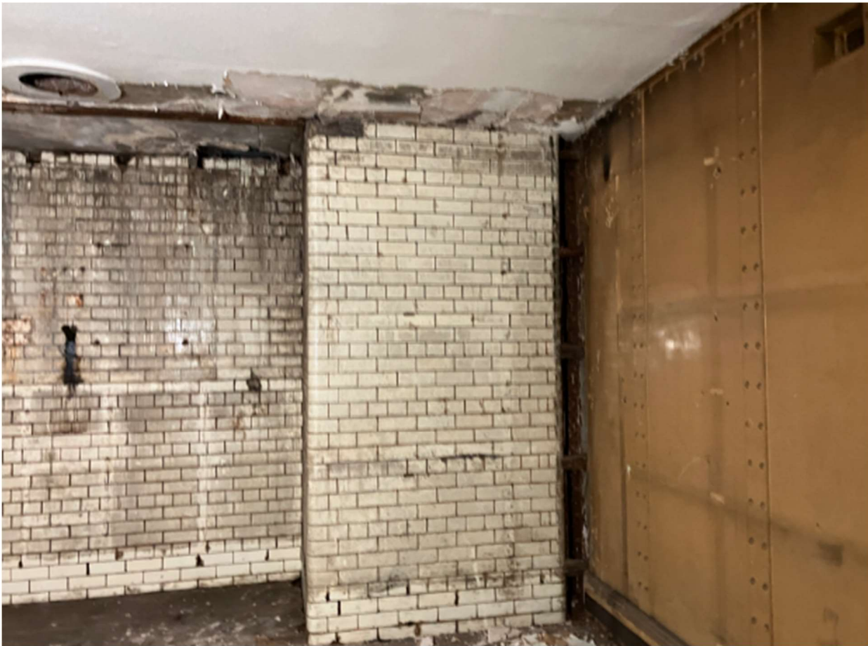
Figure 6 – View on Existing Basement Walls to Front Elevation (Metal Panel Partition Wall Shown to Right-Hand Side)
