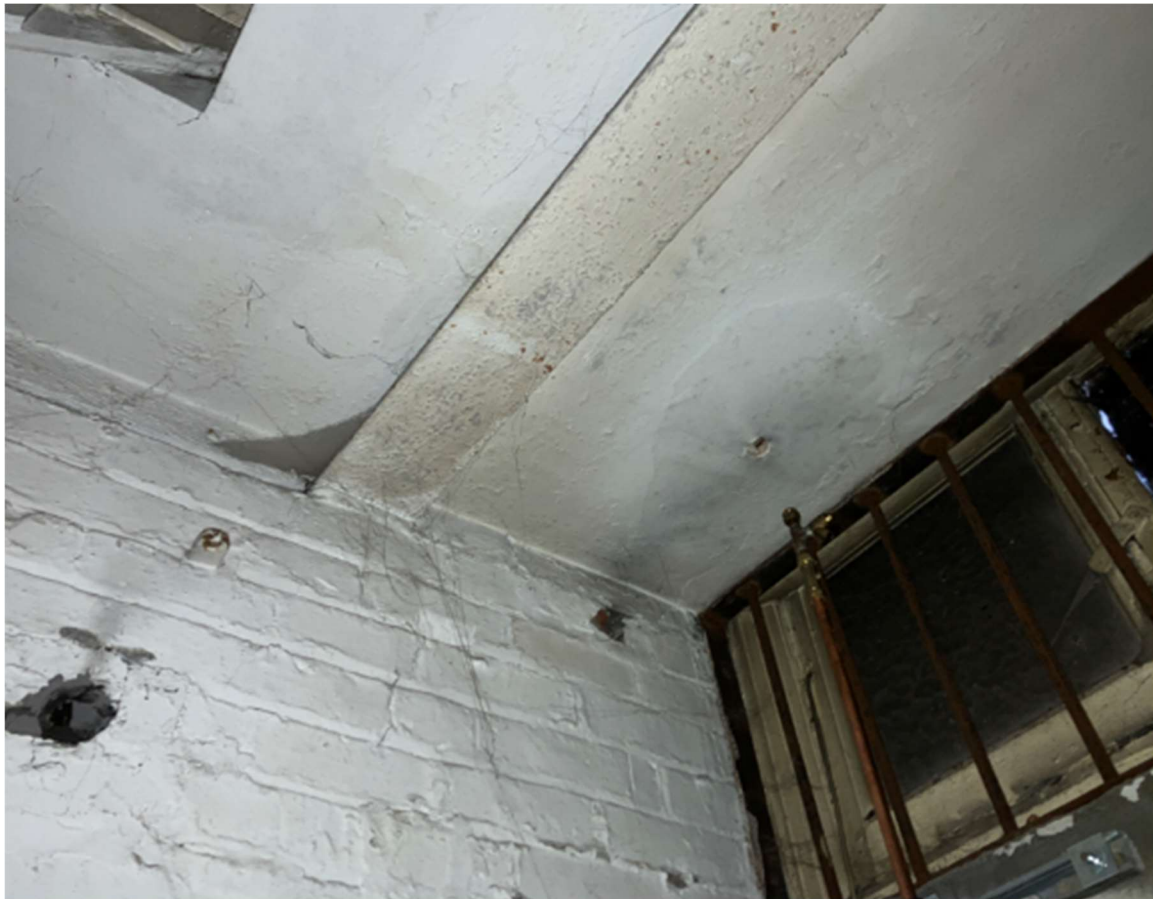
Figure 11 – Primary Beam Bottom Flange with Filler Joist Floor Infill (as Witnessed from Basement Level)
