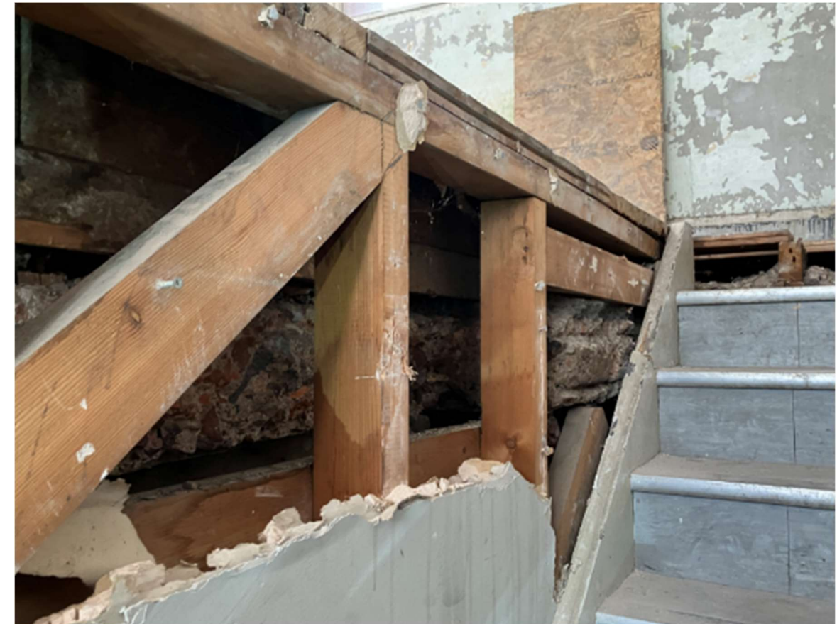
Figure 14 – View on Filler Joist Floor Slab Edge at Basement Access Stair
