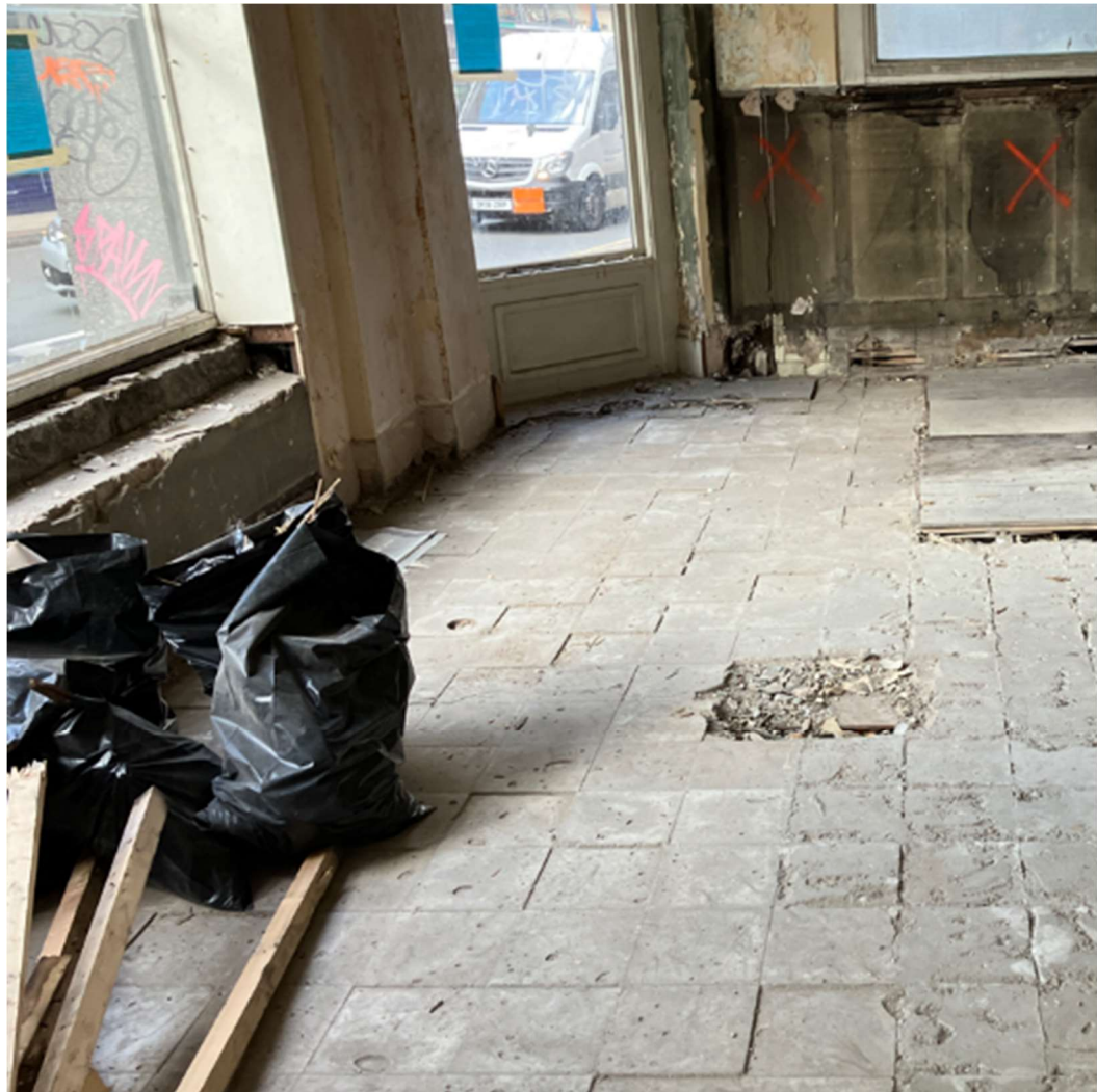
Figure 21 – Previous Intrusive Investigation Location (Top Flange of Primary Steelwork Member Visible)
