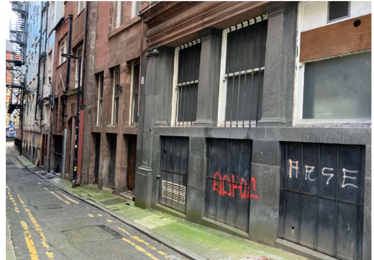
Figure 24 – Rear Elevation of Building (Four Yards)
