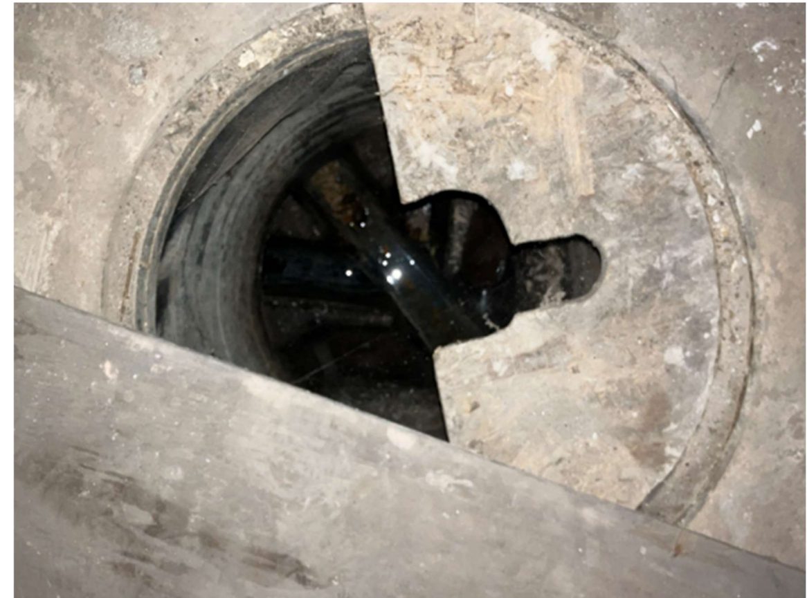
Figure 10 – Existing Uncovered Manhole Chamber
