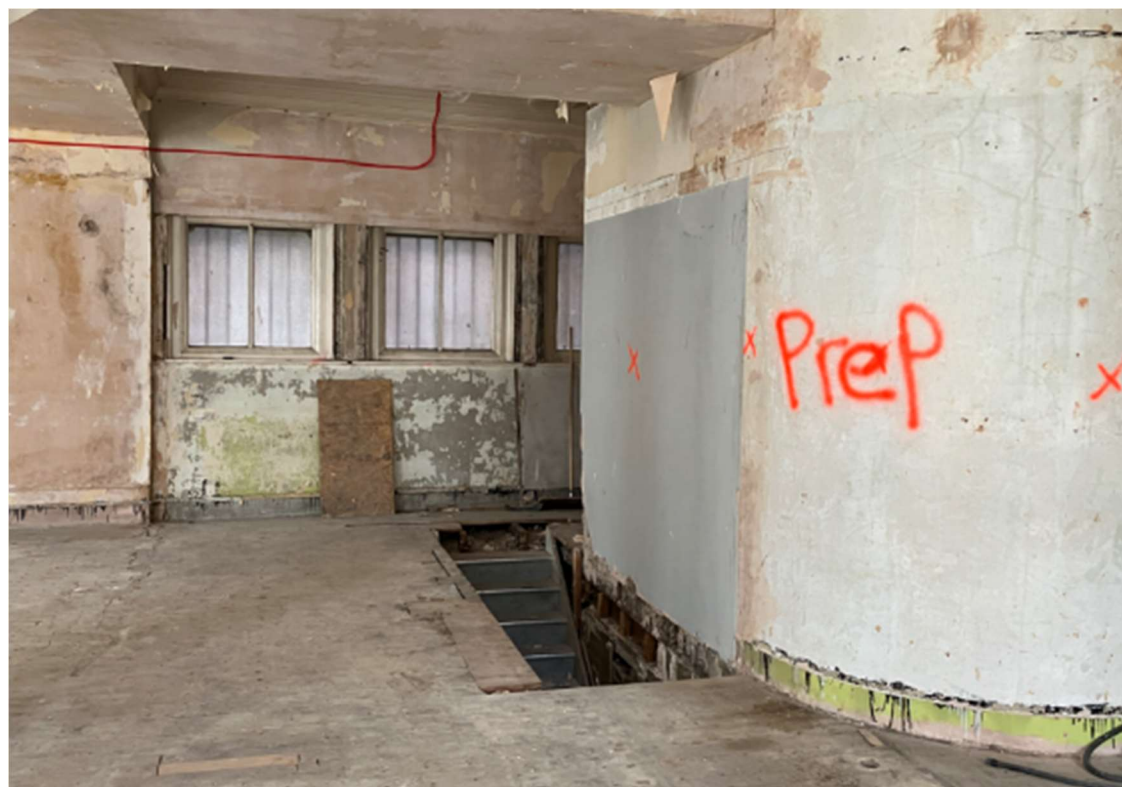
Figure 19 – Curved Masonry Wall Adjacent to Basement Access Stair
