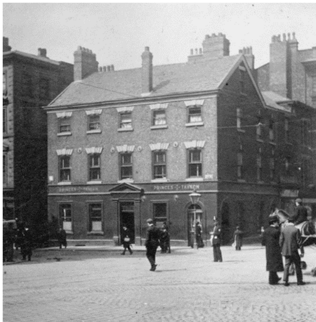
Figure 2 – Former Princes Tavern (on corner of John Dalton Street and Cross Street)
