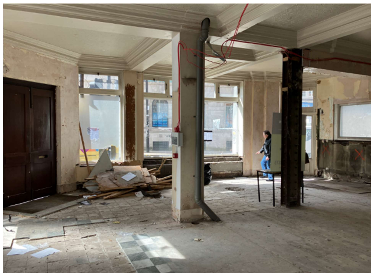
Figure 15 – General Ground Floor View Looking onto John Dalton Street
