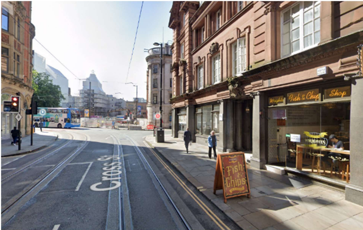
Figure 4 – Recent View Looking South on Cross Street (Showing Sub-Divided Ground Floor Commercial Units and Metrolink Infrastructure)
