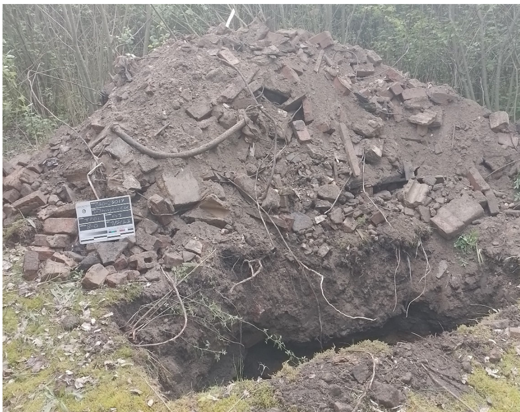
Photograph 1 – Excavated TP01 with arisings.
