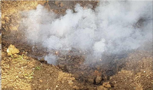
Aftermath of Demolition
