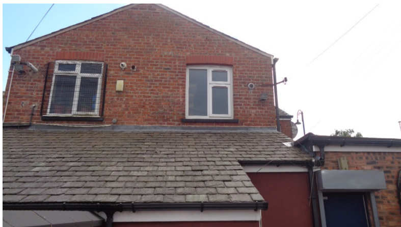
Rear of Application Property.
