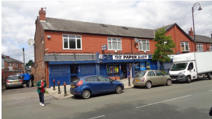
Front Elevation to Application Property.
