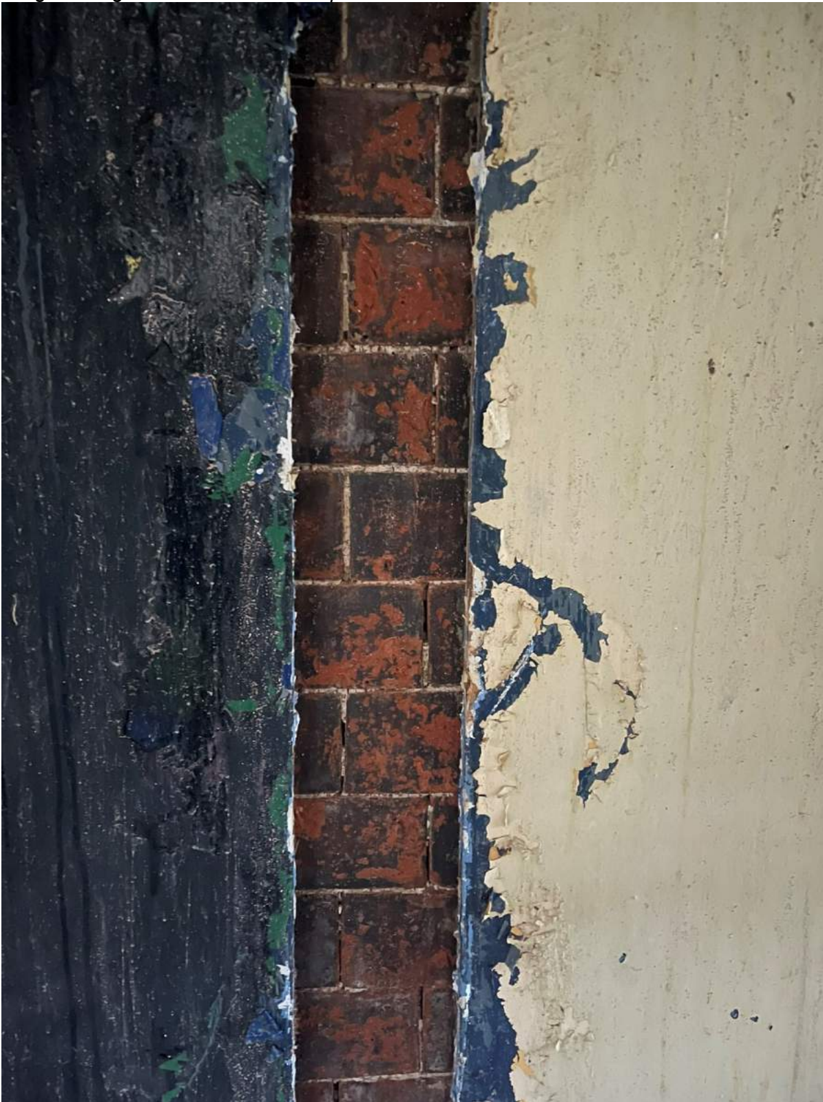
Image 6: Original Mortar to 125 Liverpool Road
