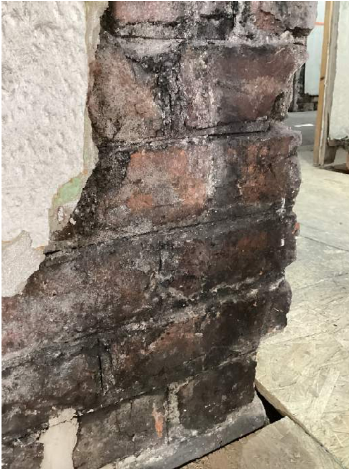
Image 3: Original Struck Pointing
