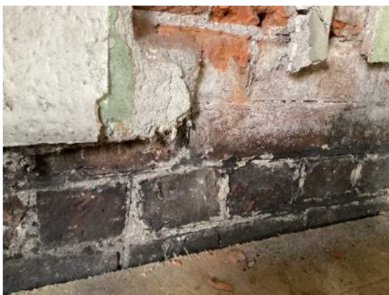
Image 2: Original Struck Pointing
