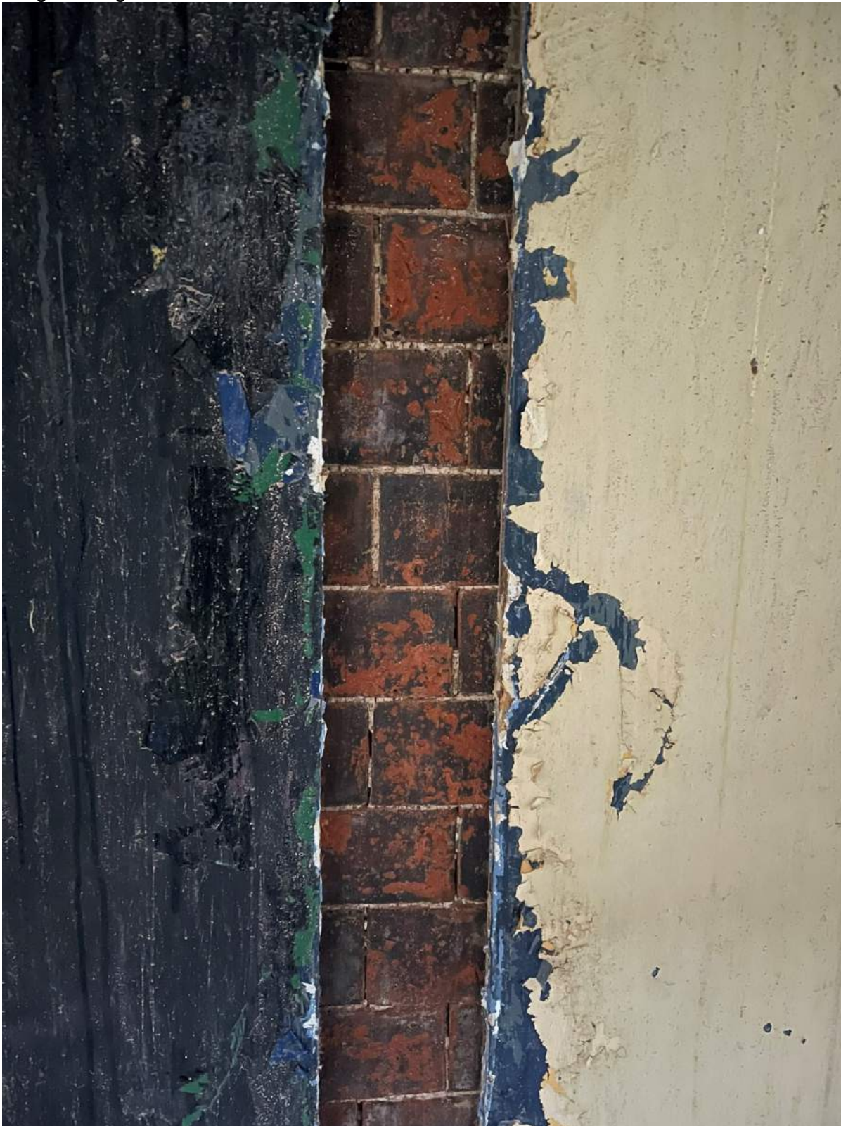
Image 5: Original Mortar to 125 Liverpool Road
