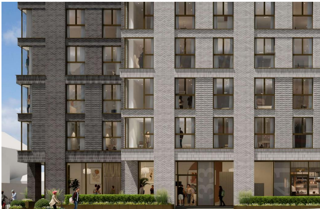
Figure 5 Appearance of the Site
